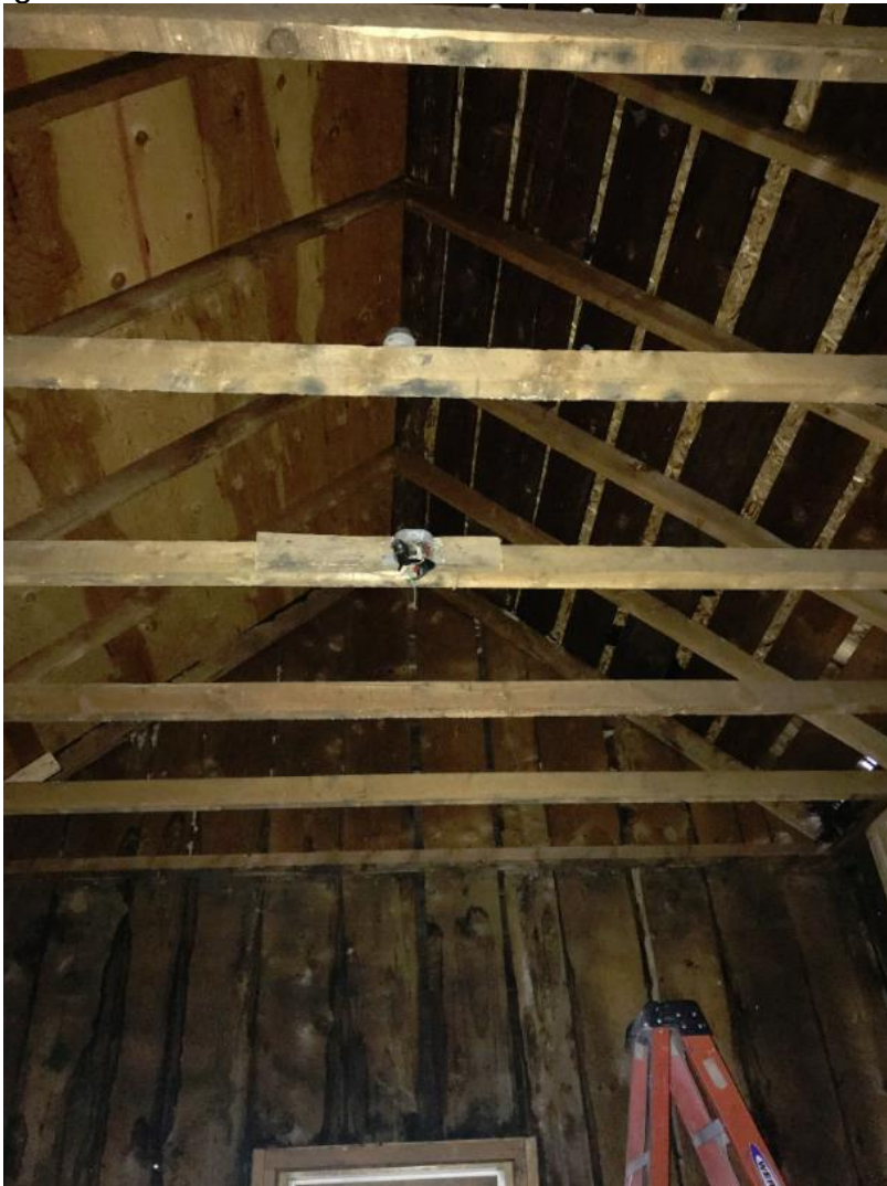
Figure 6 Existing interior roof structure
