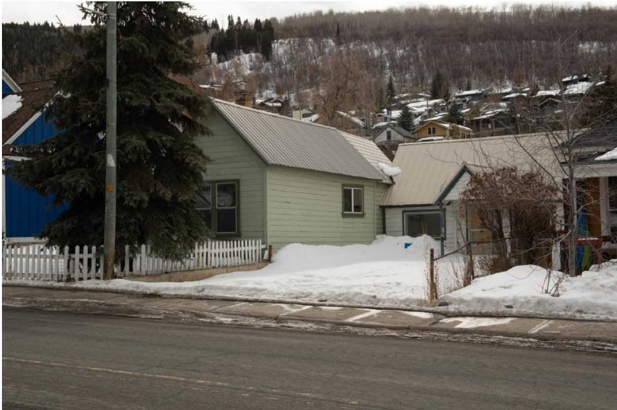
1125 (left) & 1129 (right) Park Avenue looking southerly
