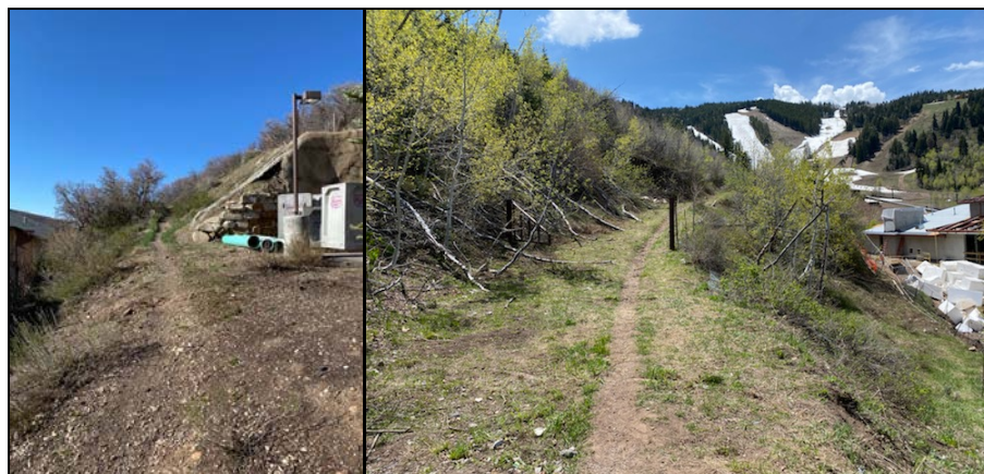
Photos Showing Trails Restored of Construction Debris
