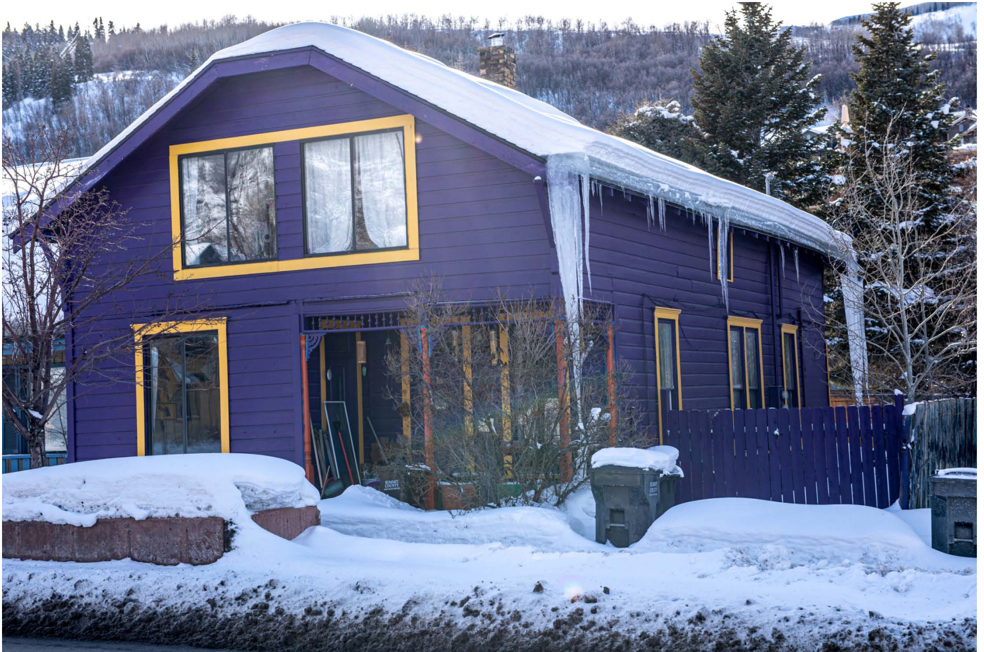
1209 Park Avenue – looking Southwesterly
