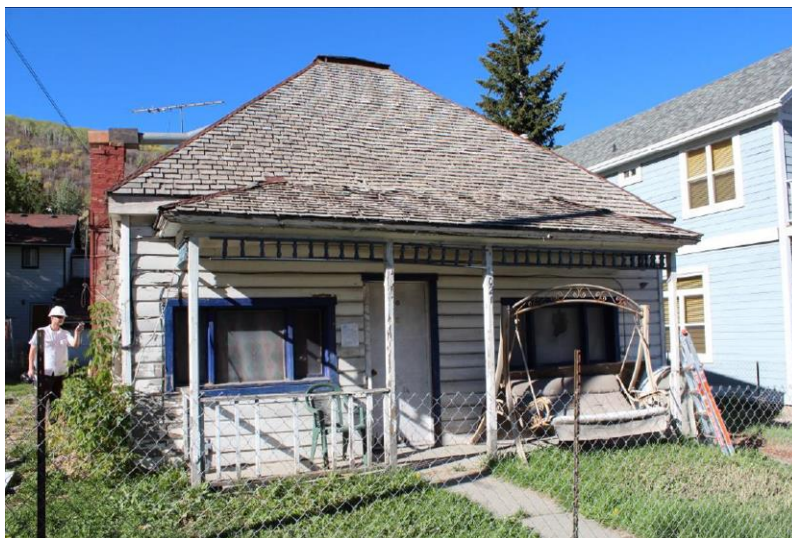
Porch as it existed in 2014
