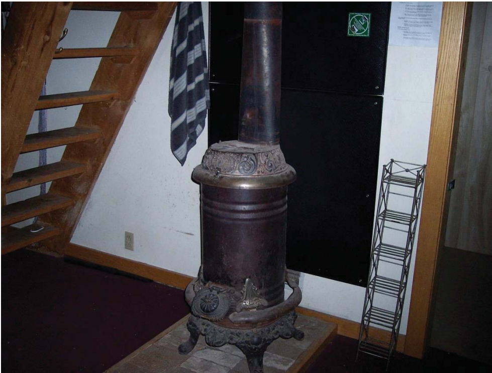
Photo 8j: Stove pipe to masonry chimney
