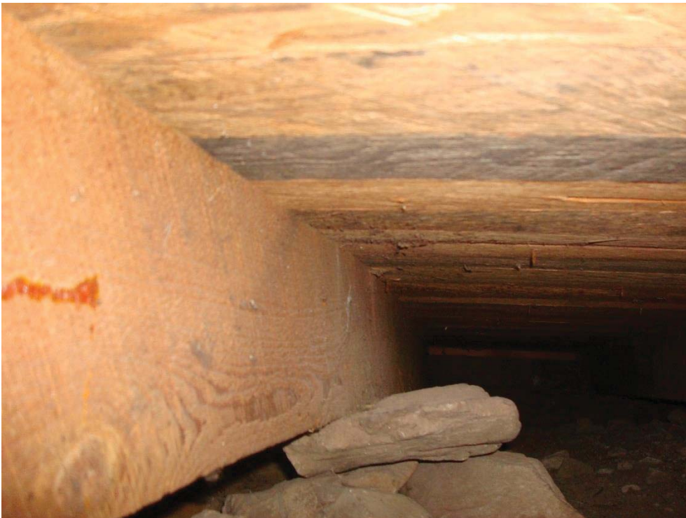
Photo 2c: Typical joist bearing on stone/soil
