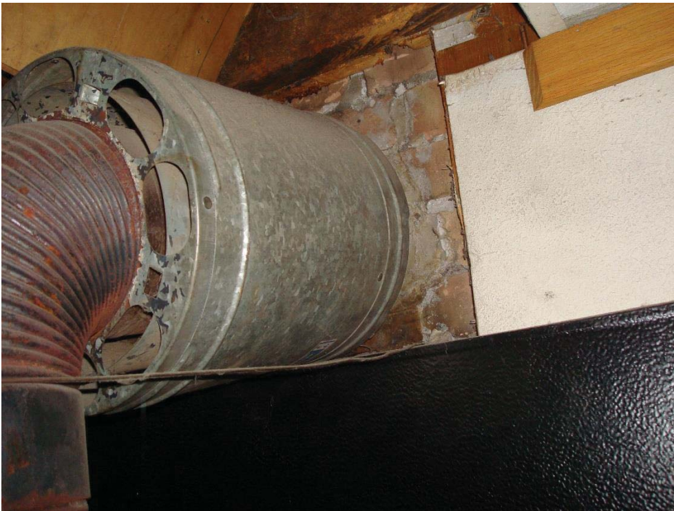
Photo 8j: Stove pipe to masonry chimney
