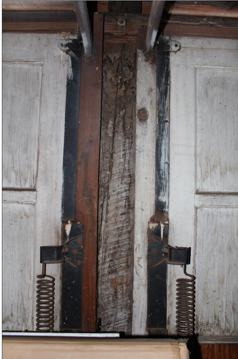
Figure 11. Door-opening and bracing hardware on original garage doors at 1503 Park Avenue, 2018, view facing south.
