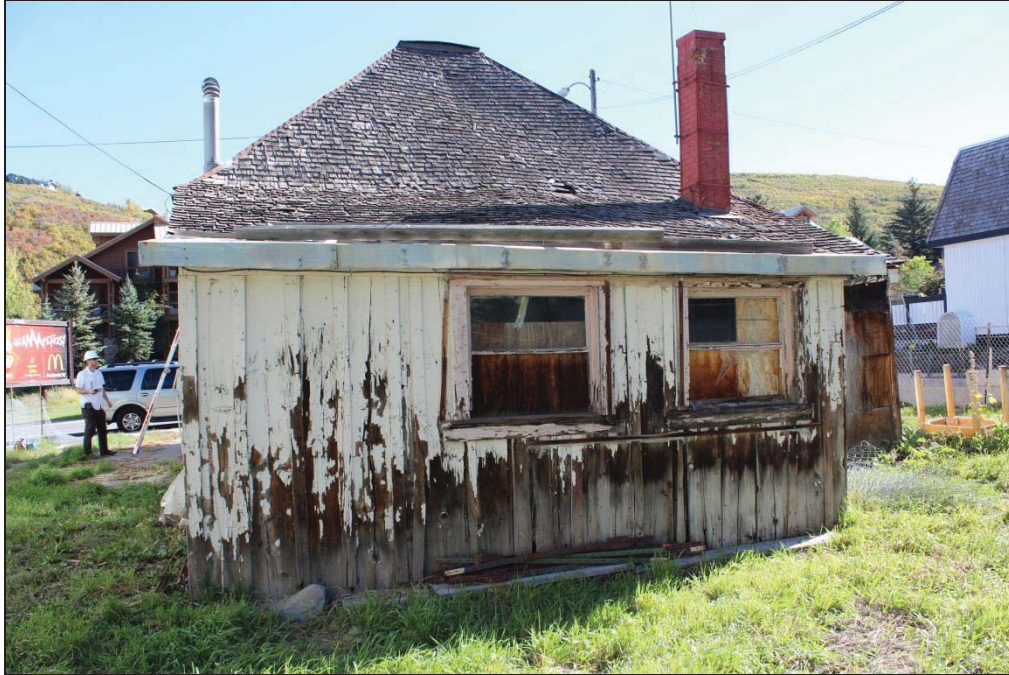
B.4. EXTERIOR WALL – REAR FAÇADE: West side, detail of Addition 2, facing east.
