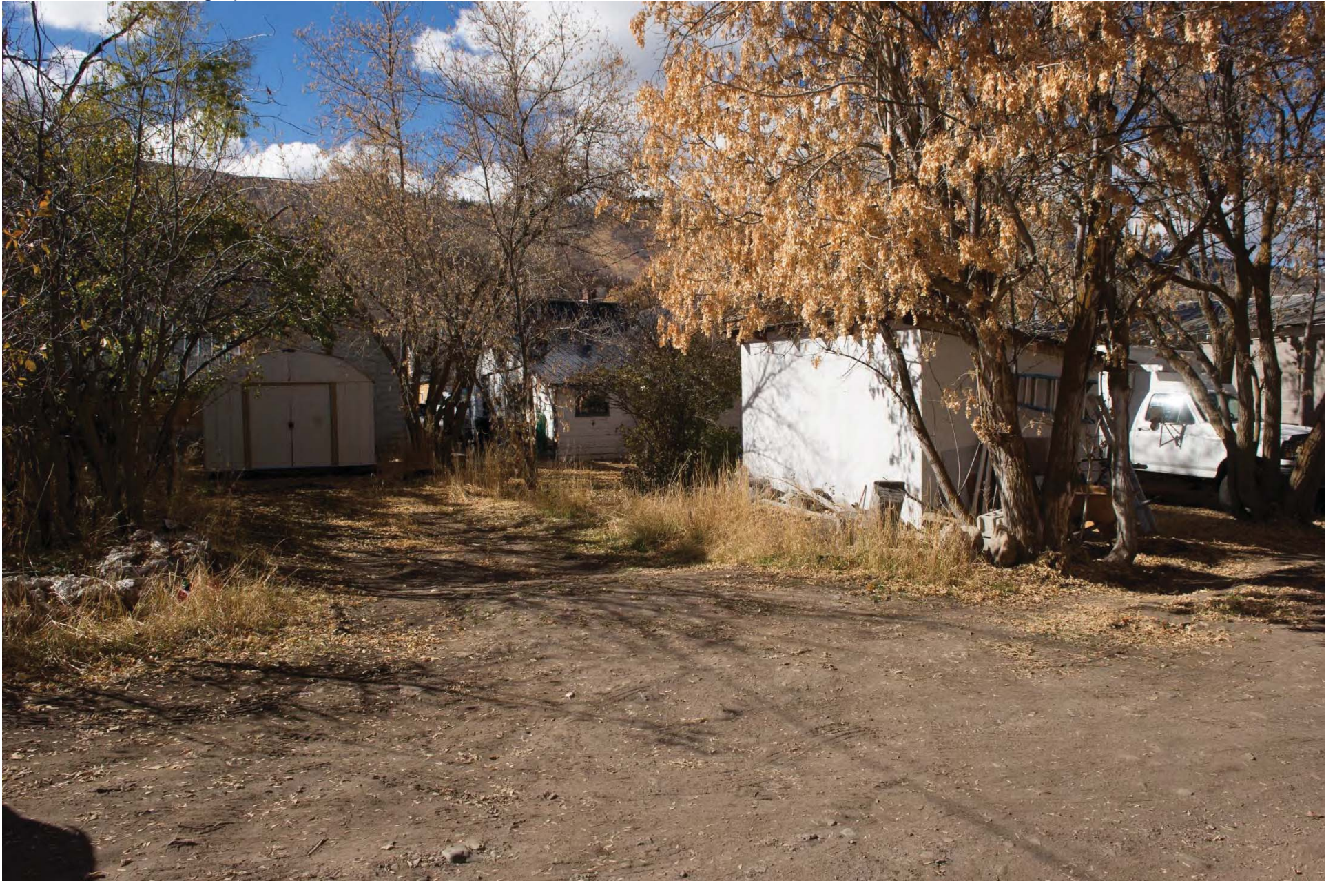
1124 & 1128 Park Avenue - looking westerly
