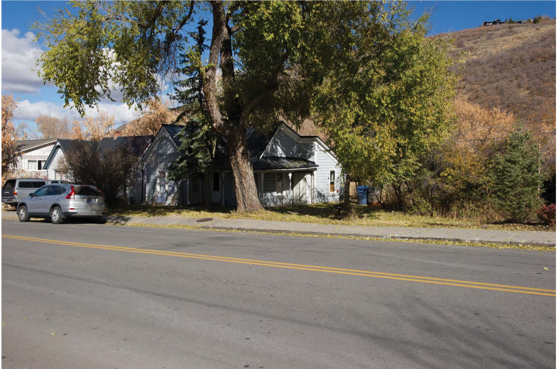
1124 & 1128 Park Avenue - looking northerly
