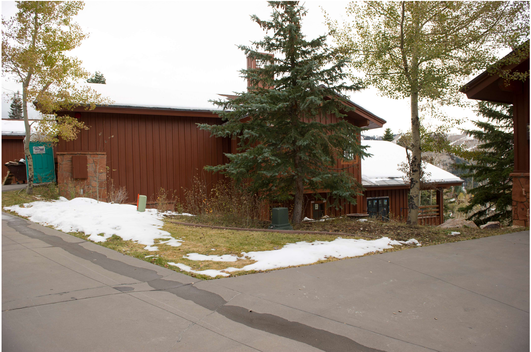
Stage Lodge Phase IV Unit 46 – Looking Southwesterly
