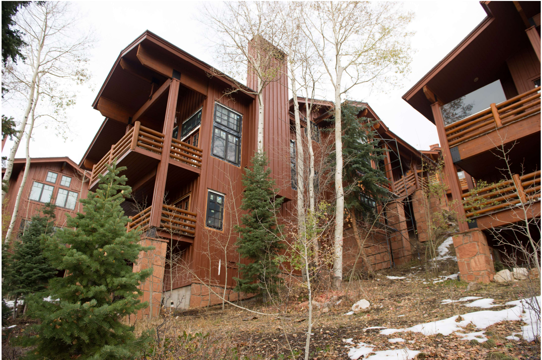
Stage Lodge Phase IV Unit 46 – Looking Northeasterly
