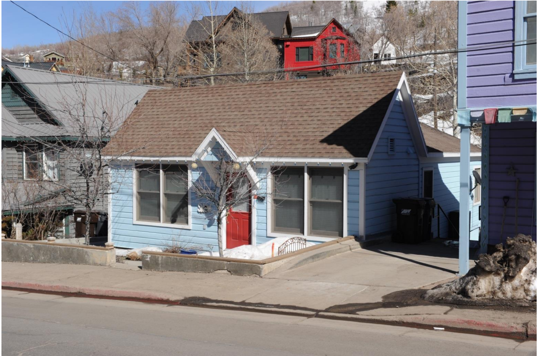
158 Main Street – looking northeasterly
