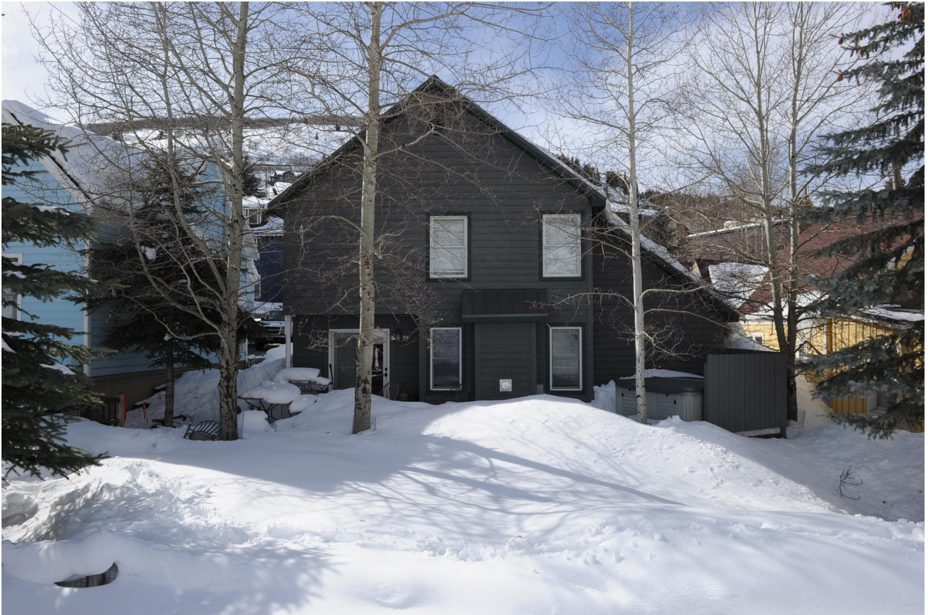
166 Main Street – looking westerly
