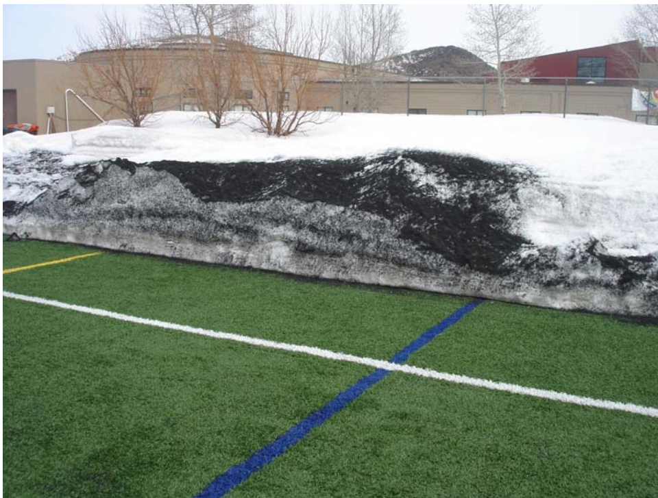
This picture shows crumb rubber mixed with snow. This is a result of using snow removal equipment.
