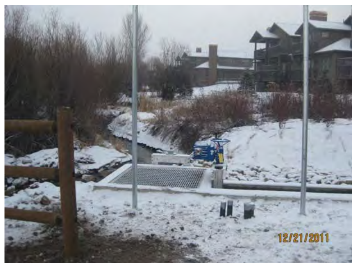
McLeod Creek Intake Structure, December 2011
