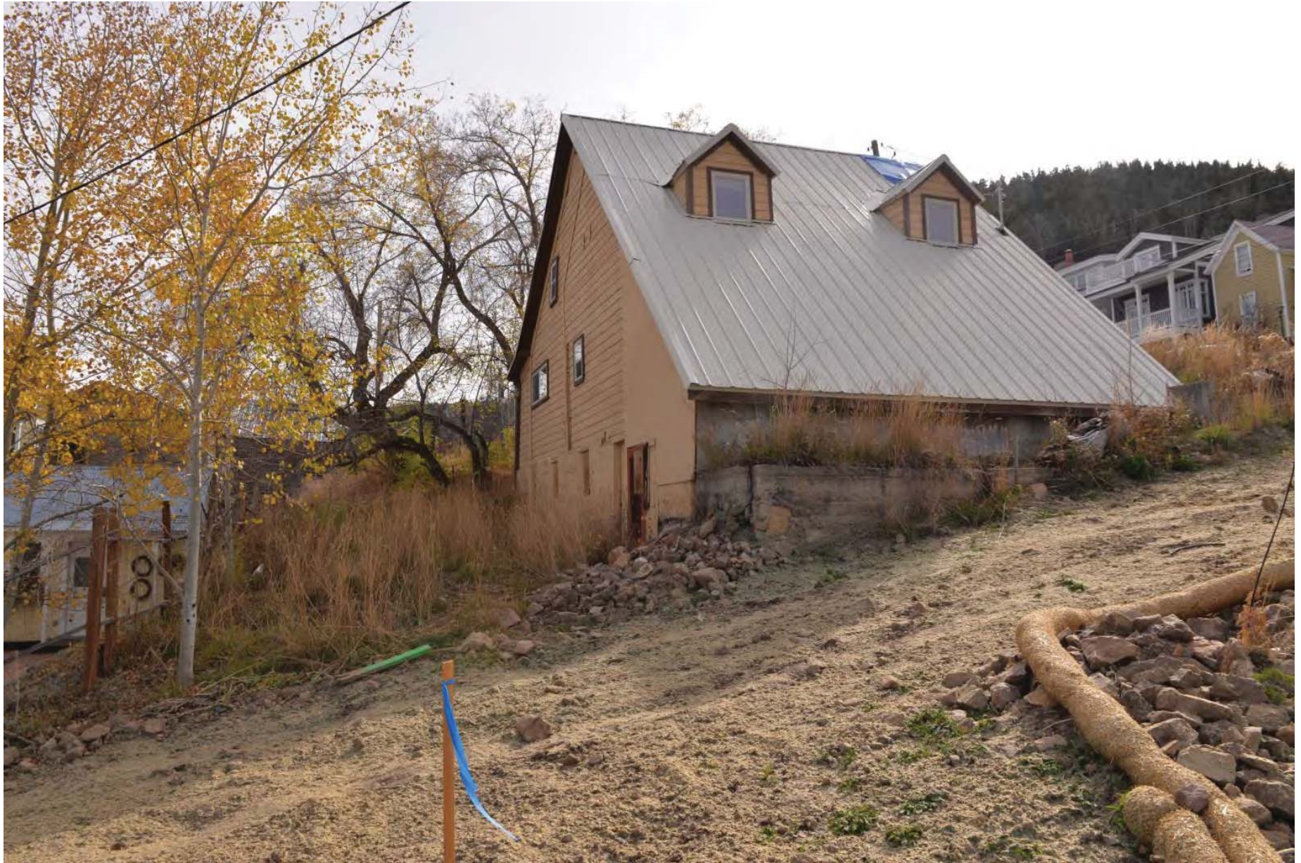
844 Empire Avenue looking southerly
