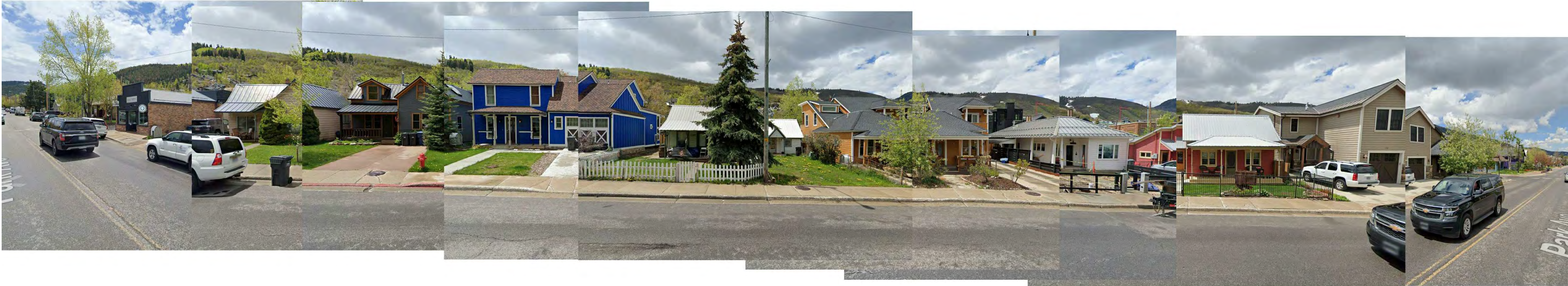
EXISTING PARK AVE STREETScape
