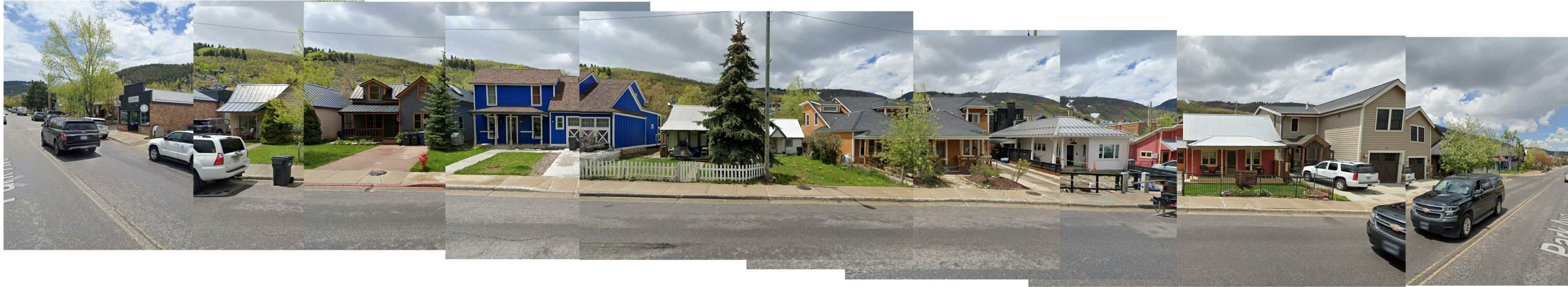
EXISTING PARK AVE STREETSCAPE
