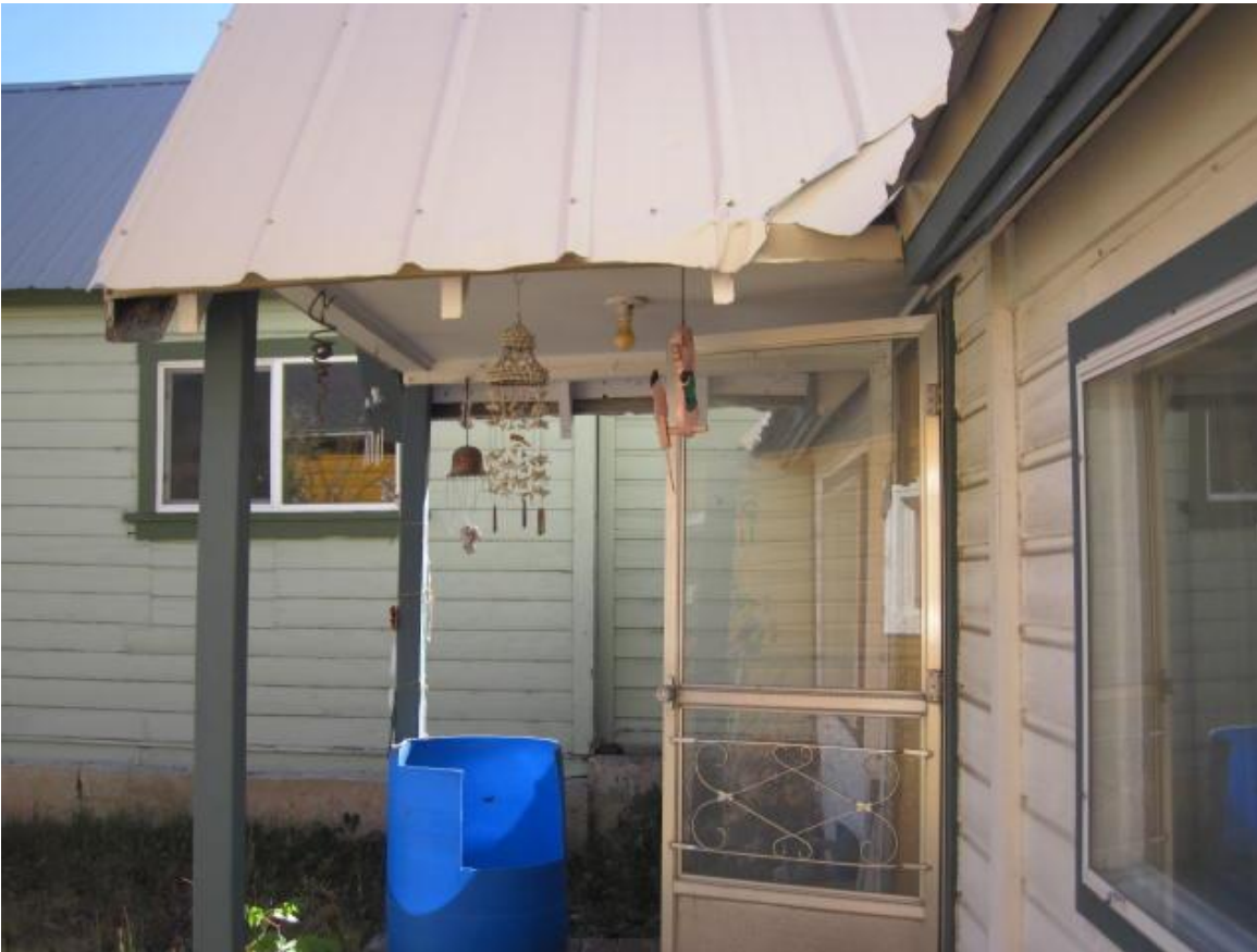
Photo 8: Covered entry porch, East elevation
