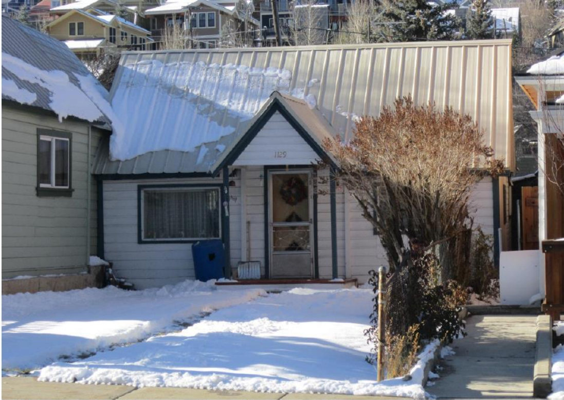
1129 Park Avenue. Northeast oblique. November 2013.
