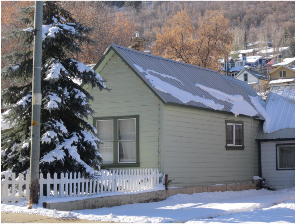
1125 Park Avenue. Northeast oblique. November 2013.
