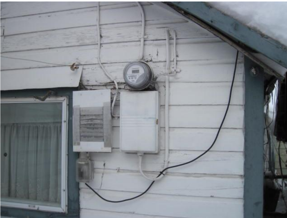
Photo 10: Electrical meter and panel
