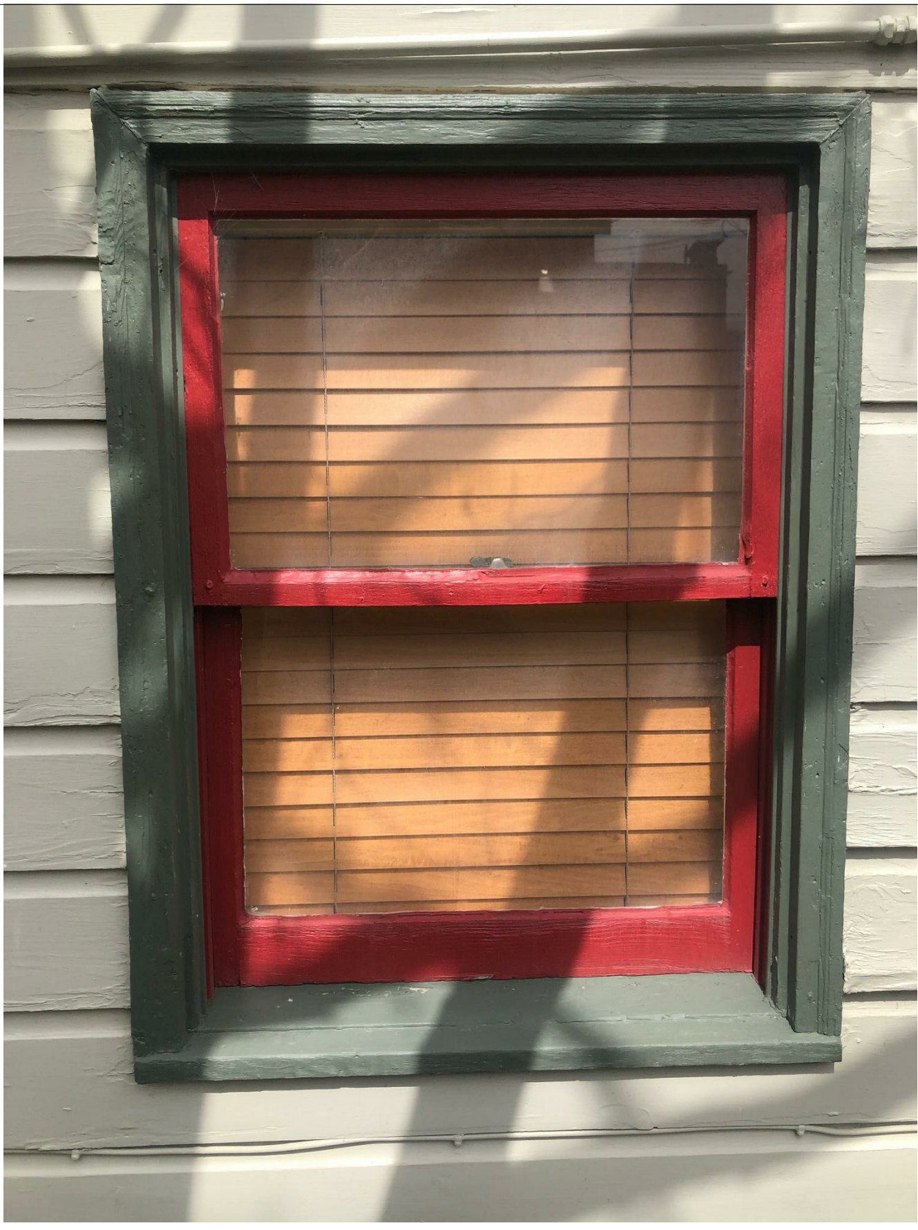
WINDOW 3 (NOT HISTORIC, TO BE REMOVED)
