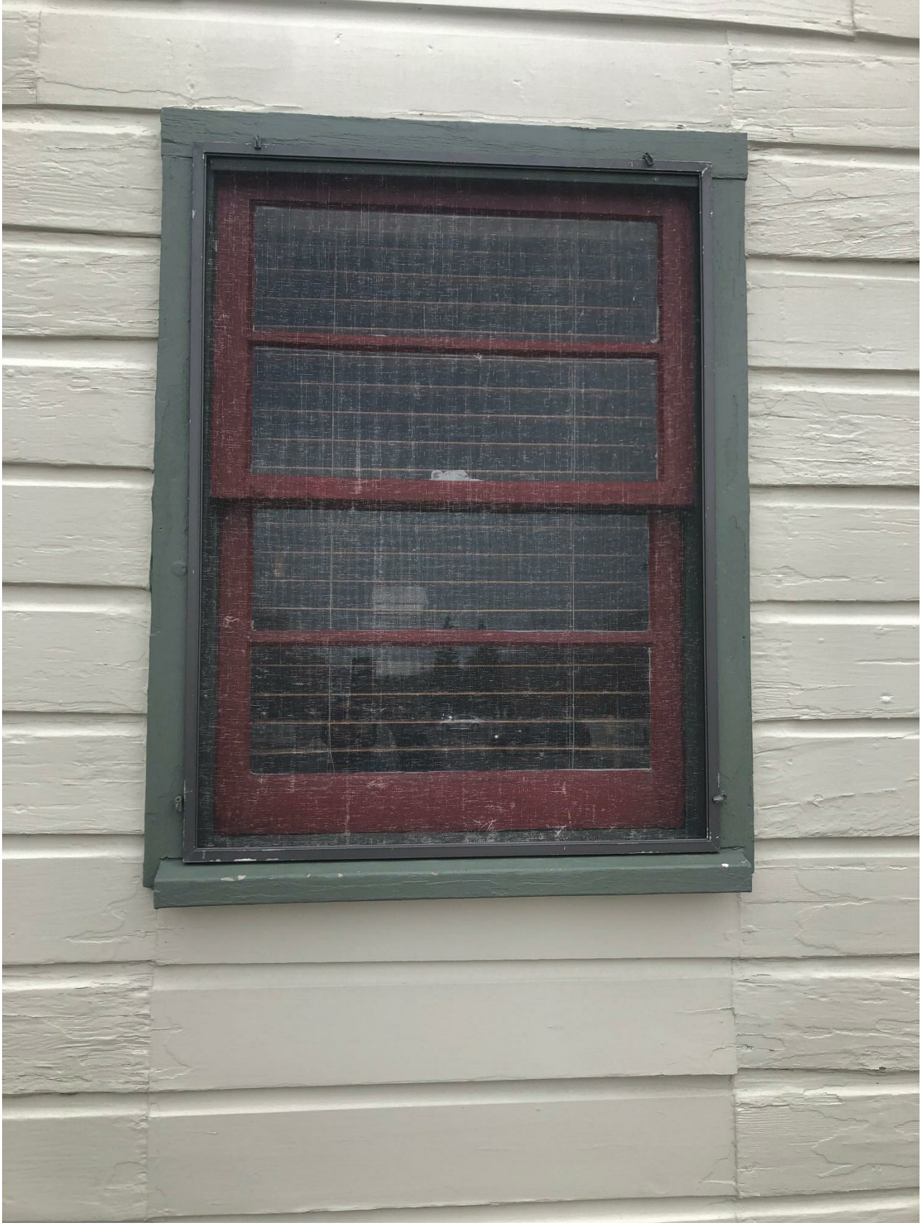
WINDOW 6 (NOT HISTORIC, TO BE REMOVED)
