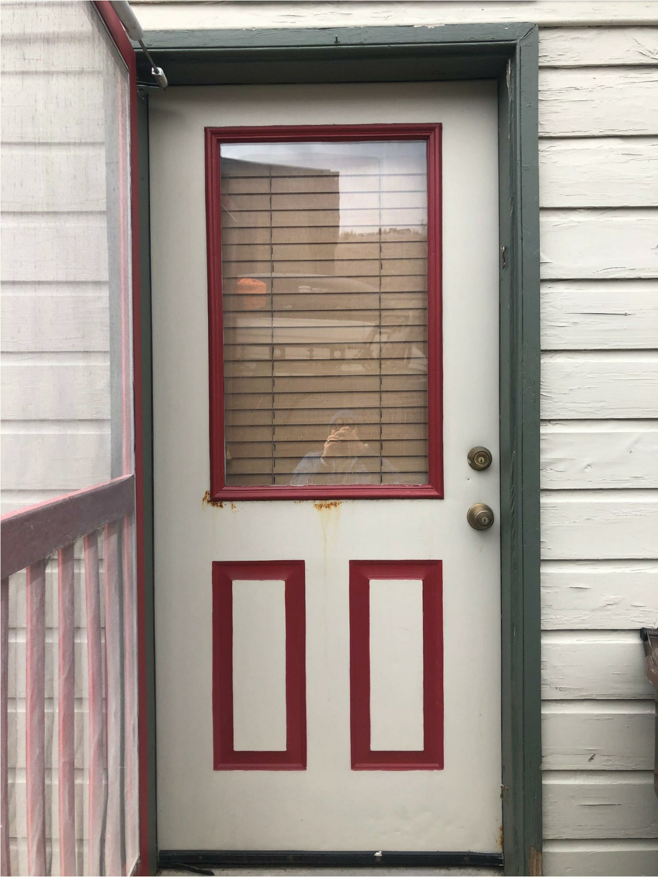
DOOR 2 (NOT HISTORIC, TO BE REMOVED)
