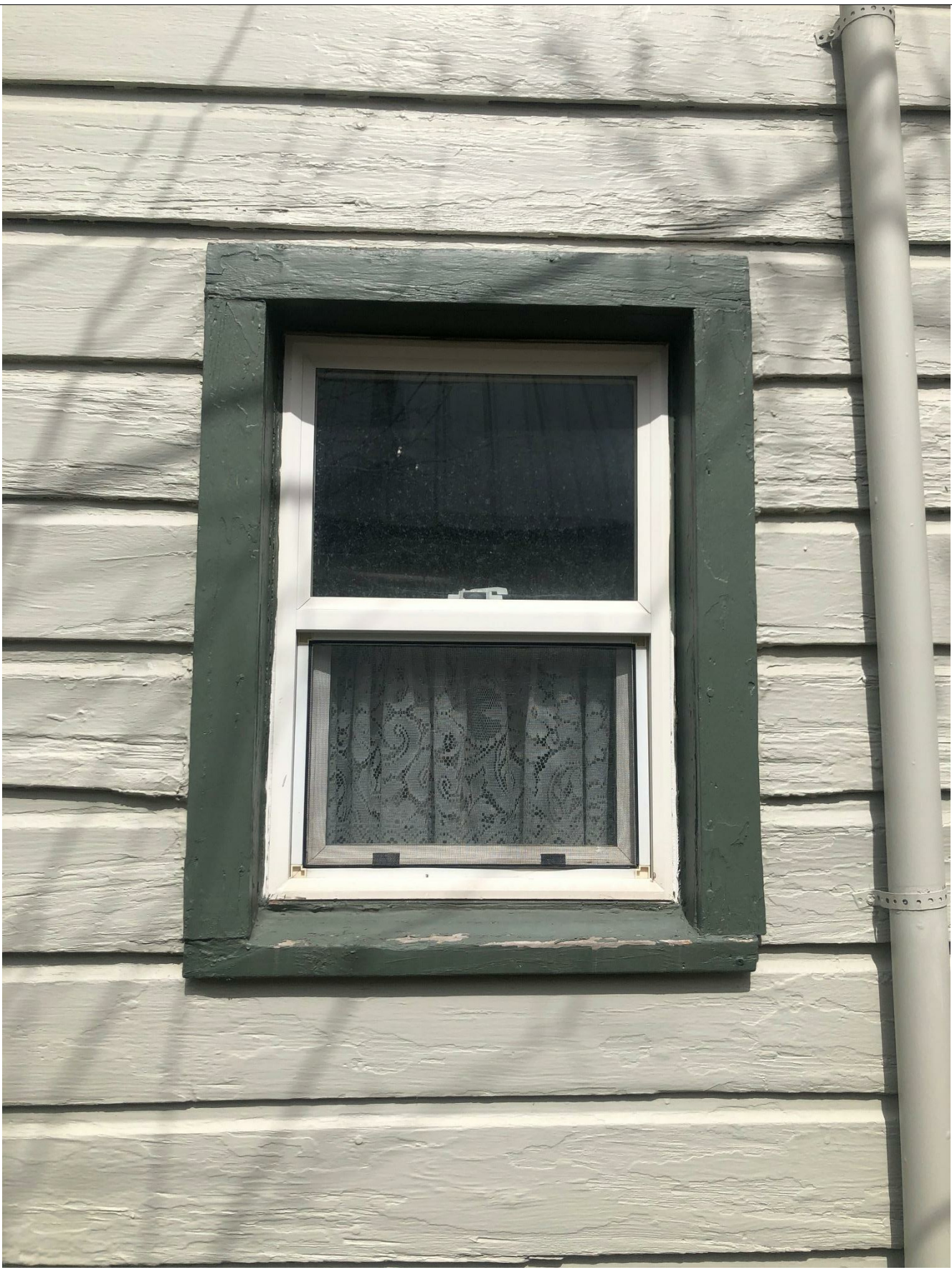
WINDOW 2 (NOT HISTORIC, TO BE REMOVED)
