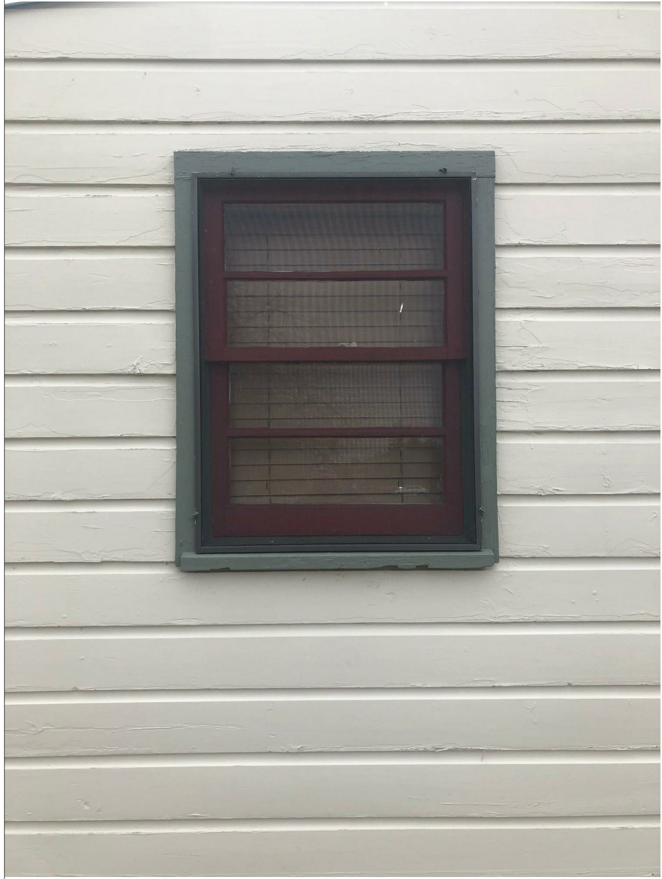
WINDOW 5 (NOT HISTORIC, TO BE REMOVED)
