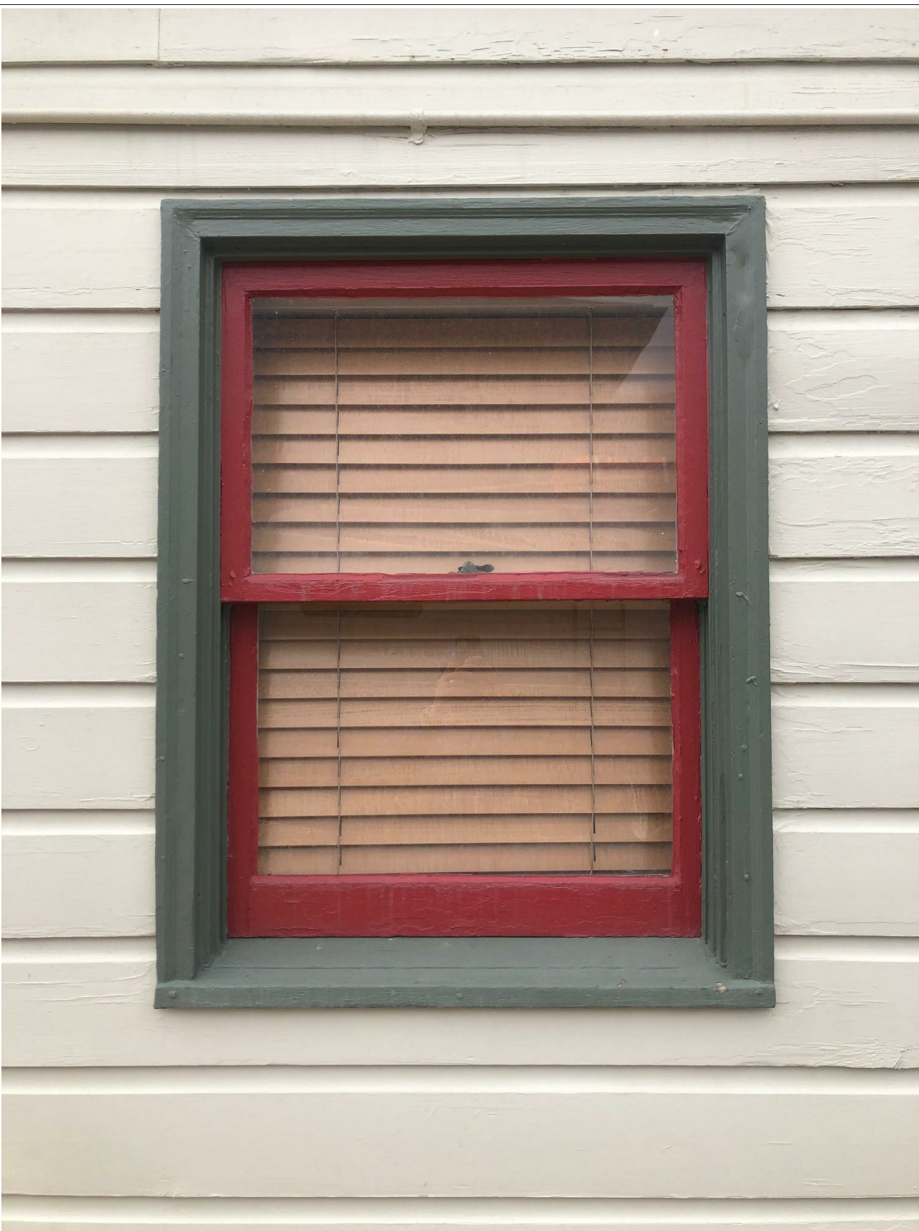
WINDOW 4 (NOT HISTORIC, TO BE REMOVED)
