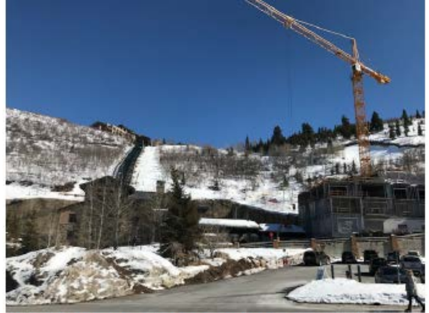
Figure 1: Phase 2 of the St. Regis Under Construction
