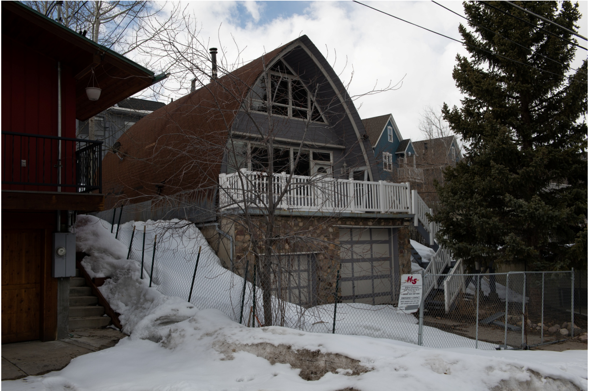
1121 Norfolk Avenue – looking Westerly
