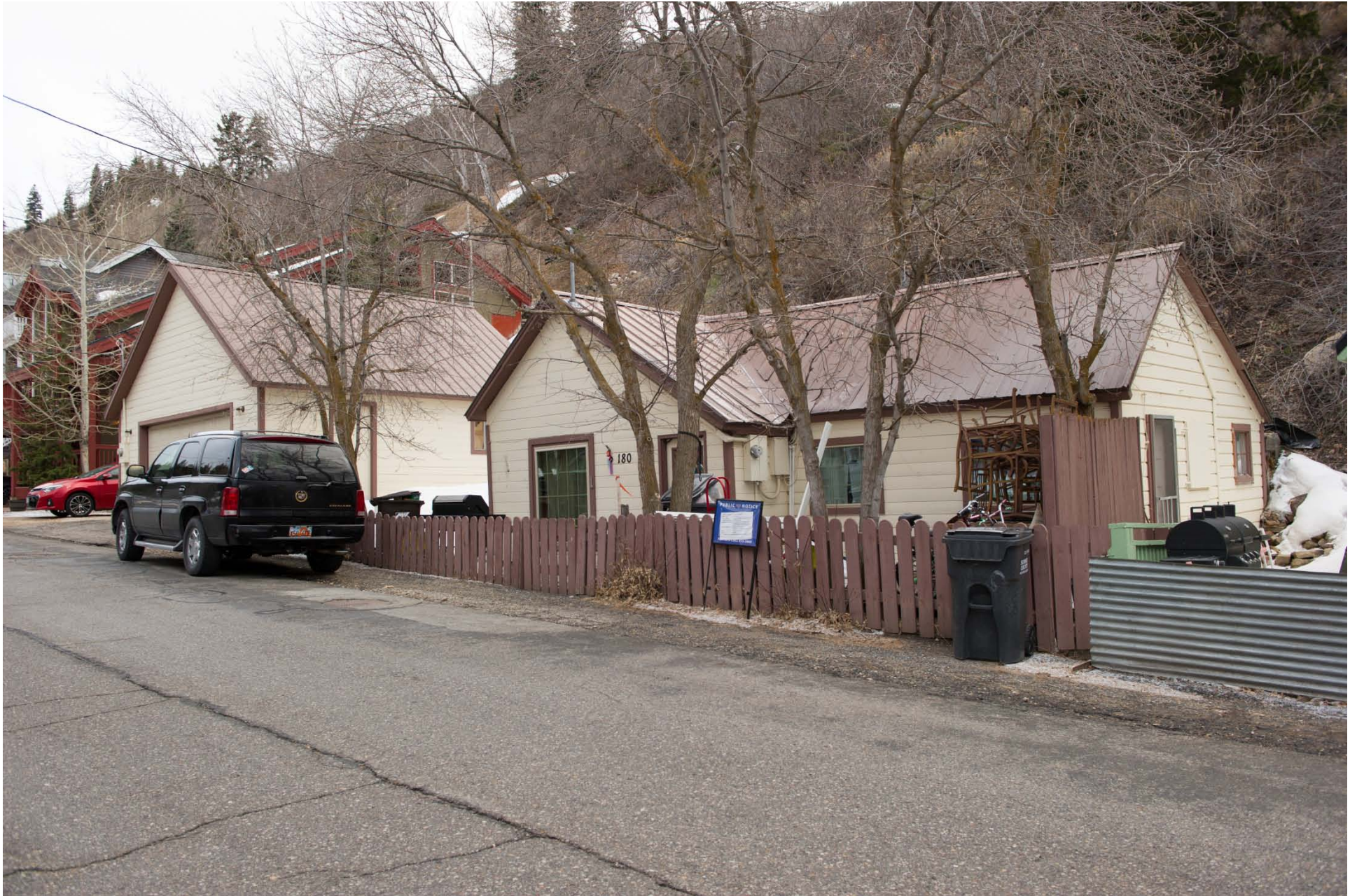
180 Daly Avenue - looking southwesterly
