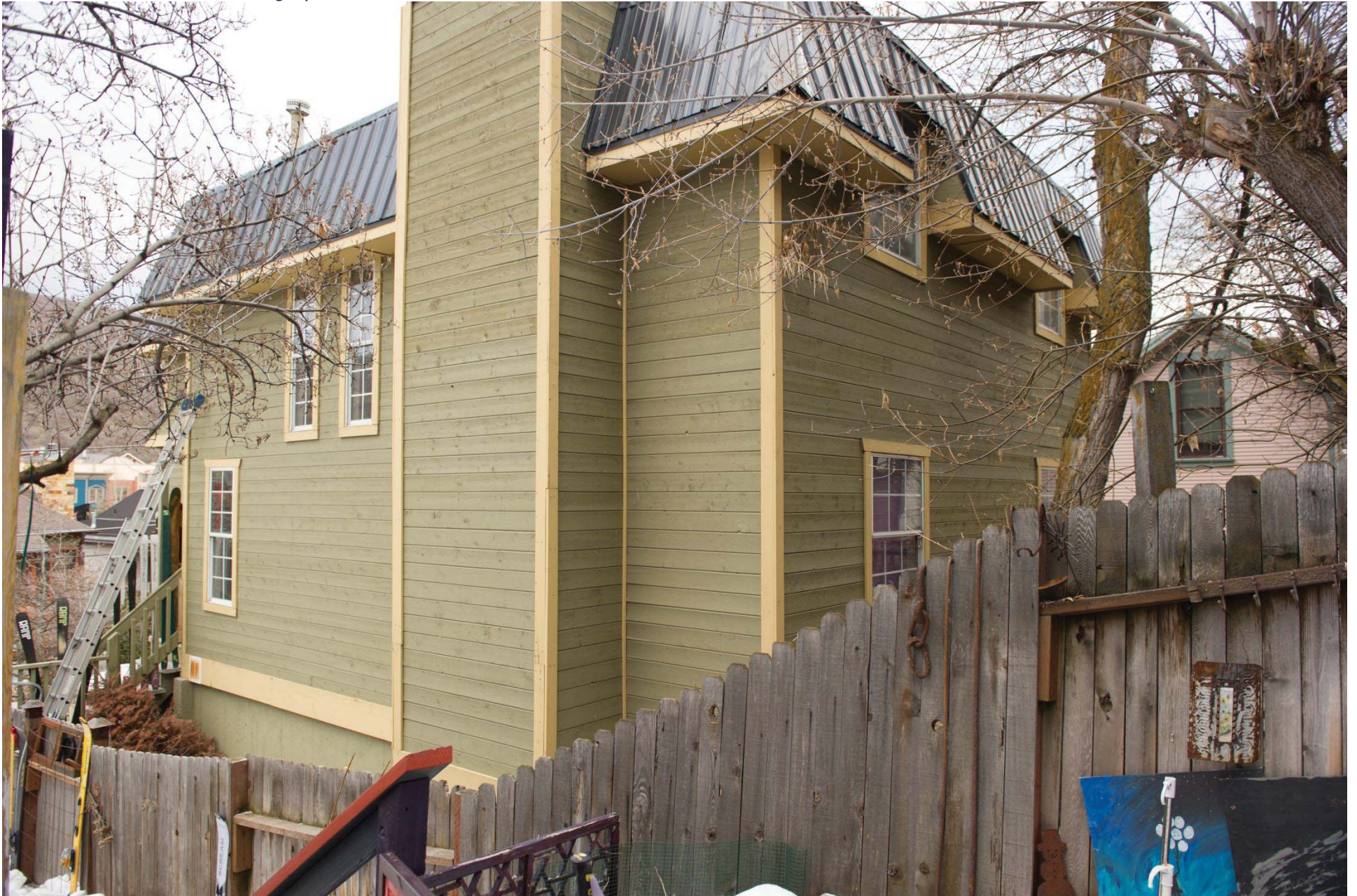
813 Woodside Avenue - looking easterly
