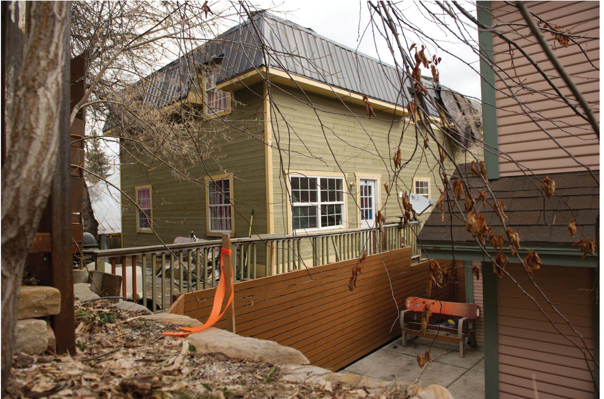
813 Woodside Avenue - looking to the north
