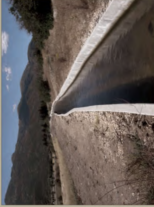
Wasatch County Water Efficiency Project cement canal lining.
