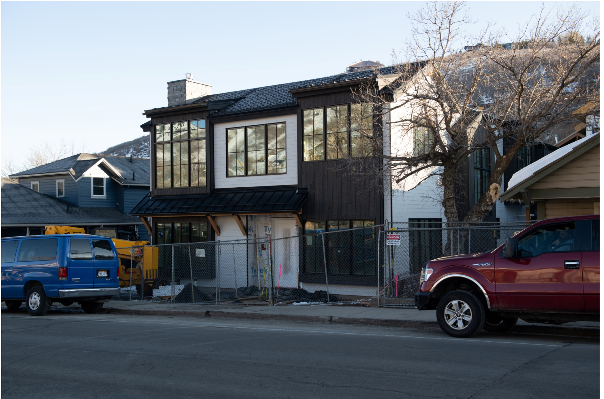
1064 Park Avenue - looking northerly
