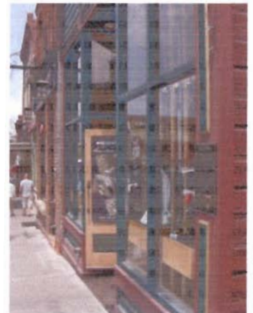
Front facade detail Park City Jewelers Building
