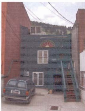
Rear View Park City Jewelers Building
