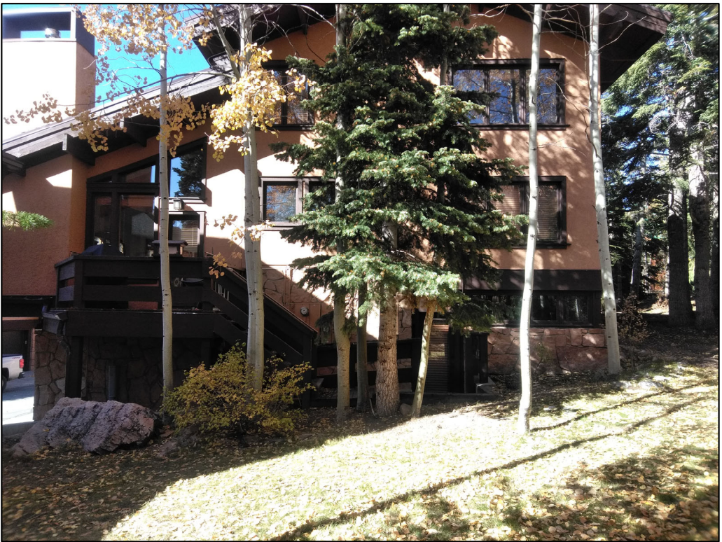
UNIT 26 SOUTH VIEW
