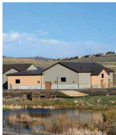
Quinns Junction WTP
