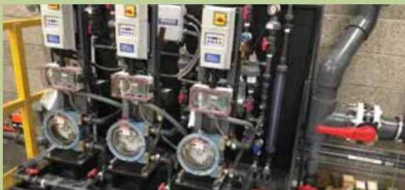
Chlorine-feed pumps
