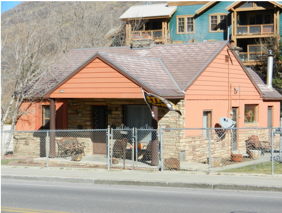
1060 Park Avenue. Southwest oblique. November 2013.
