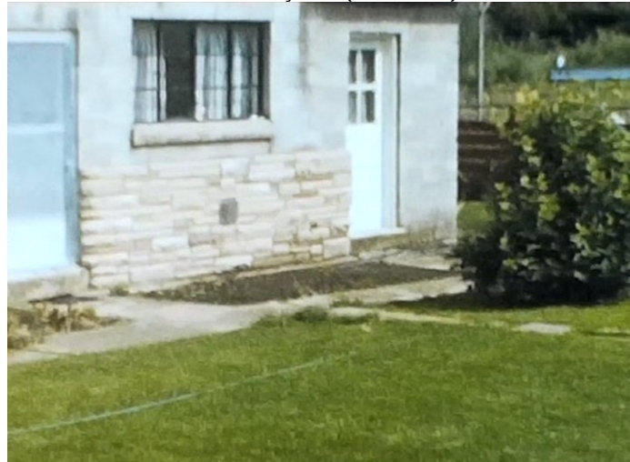
South façade (rear half)
