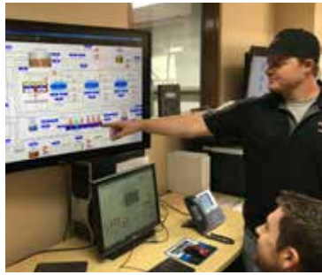
Operators monitoring water treatment plants
