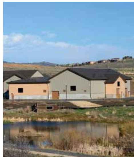
Quinns Junction Water Treatment Plant
