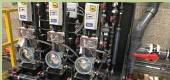
Chlorine-feed pumps
