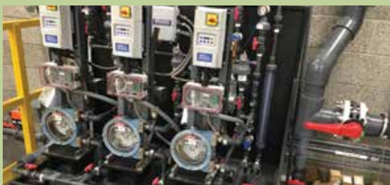
Chlorine-feed pumps
