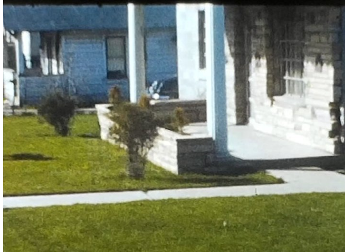
Front porch facing north.
