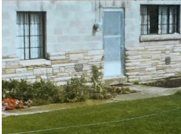
South façade (front half)
