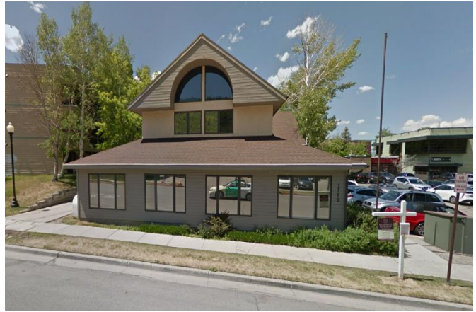
Previous Structure from 1988
