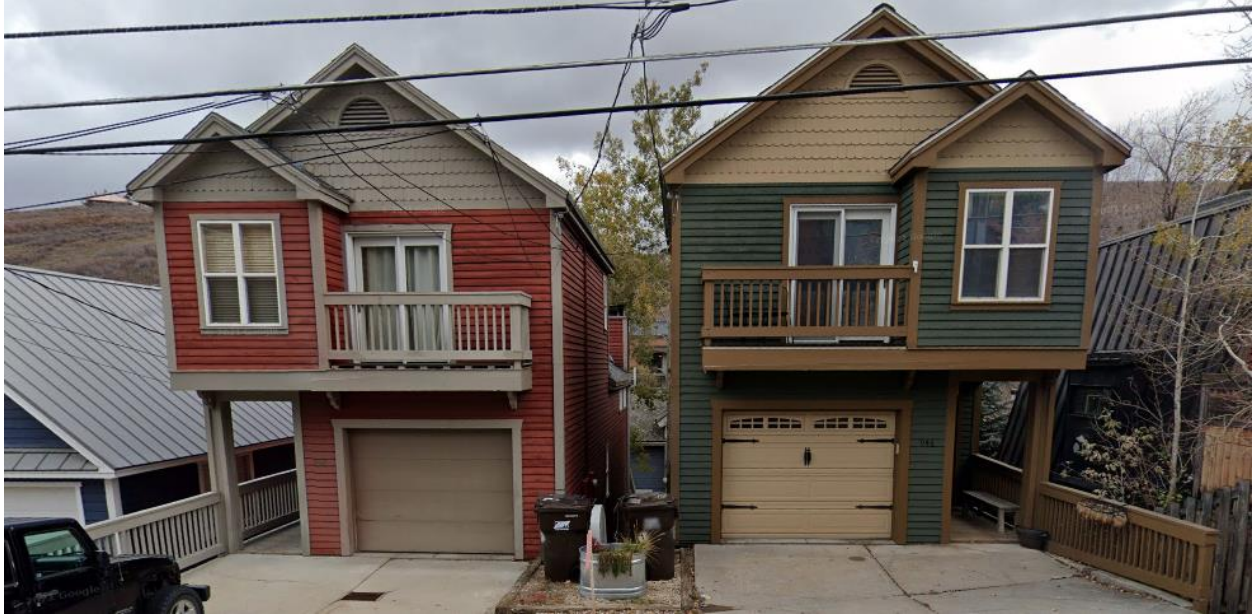
Figure 1: Street view of 948 Woodside Avenue (left).
