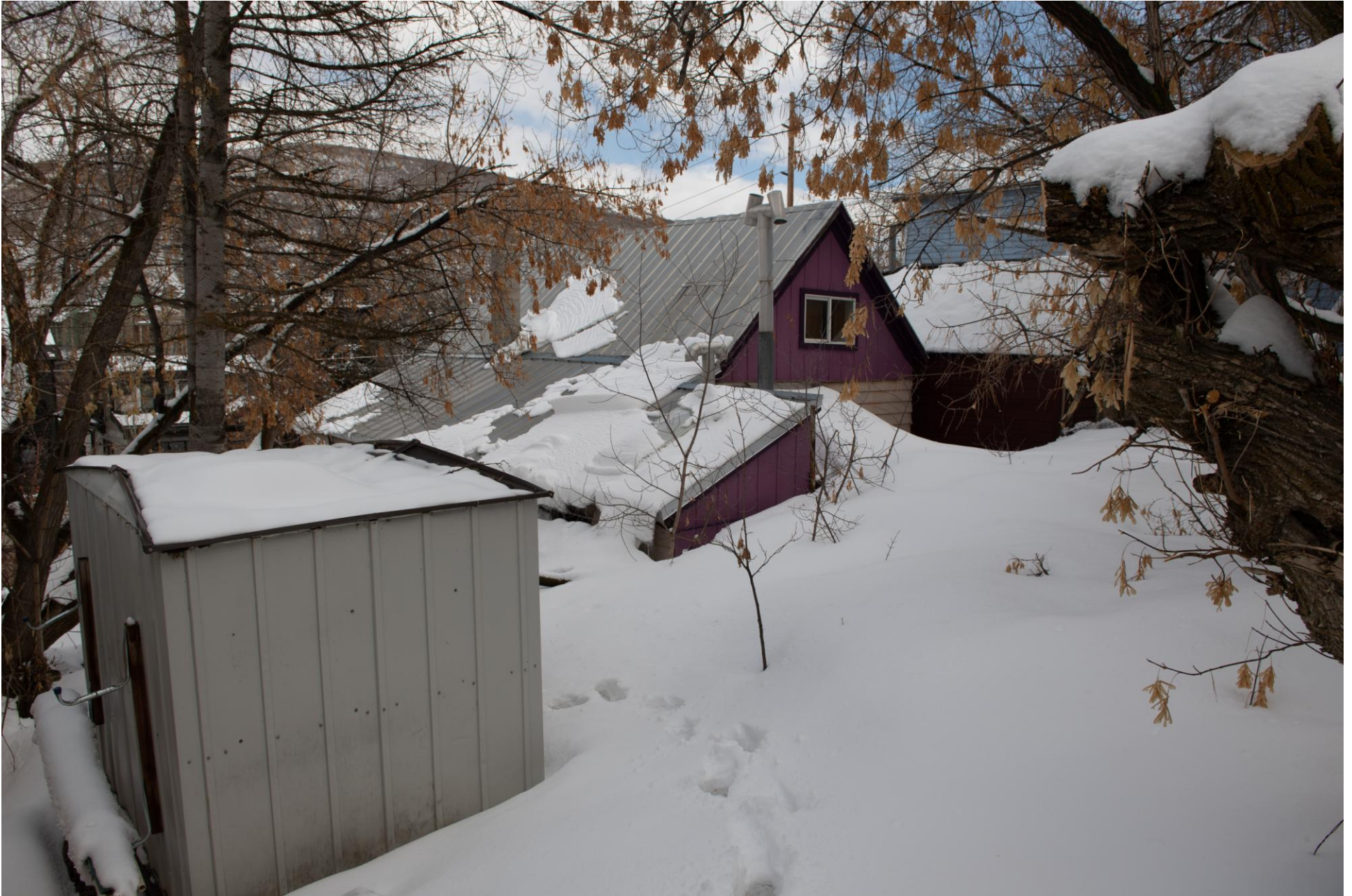
909 Woodside Avenue - rear - looking easterly
