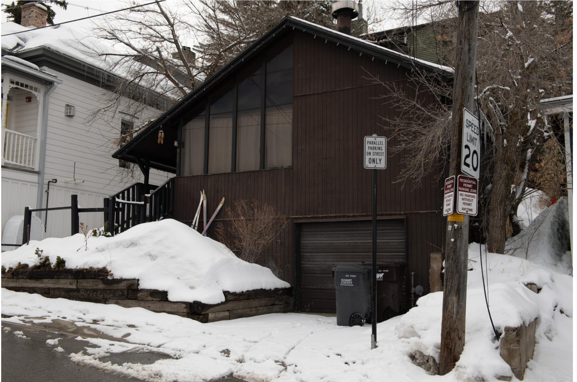
917 Empire Avenue - front - looking southwesterly
