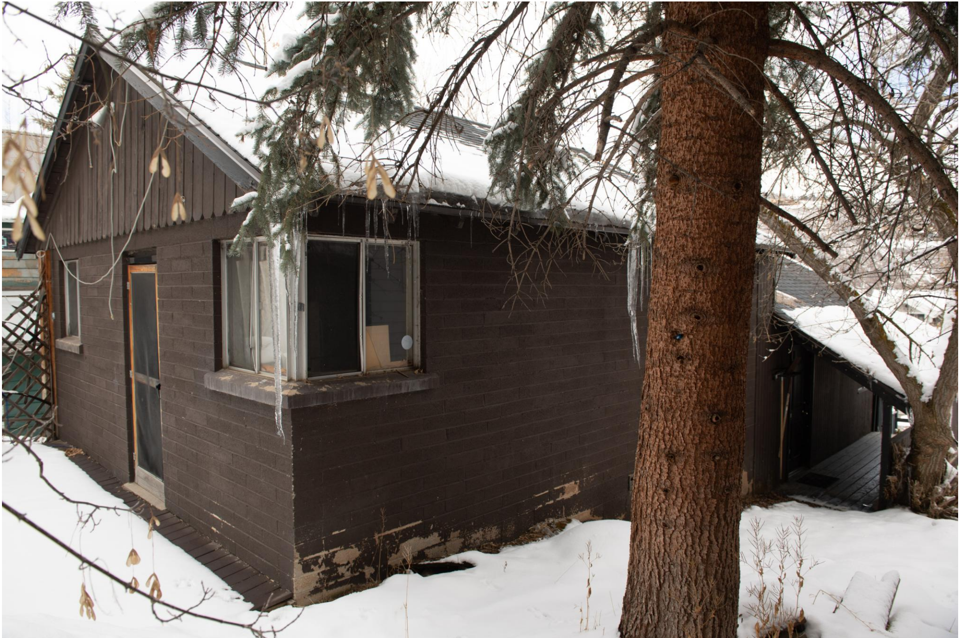
917 Empire Avenue - rear - looking north
