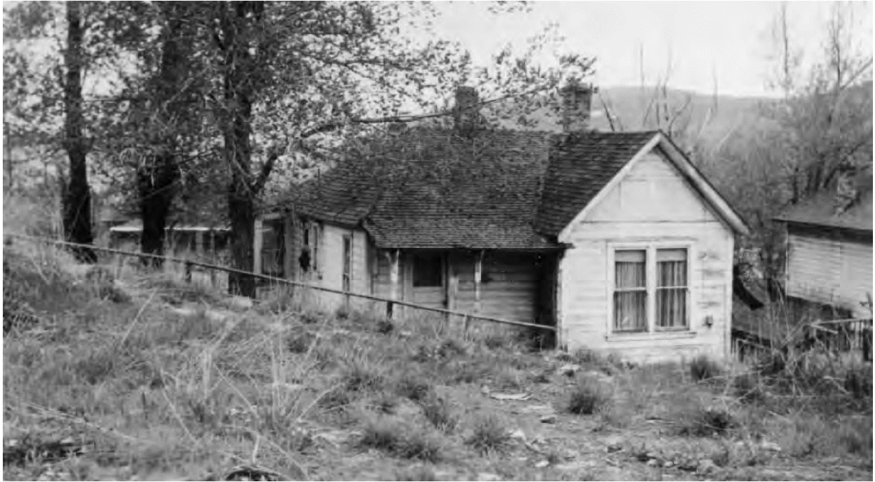
Figure 1: 1920s photograph facing south and looking at Front Facade.
