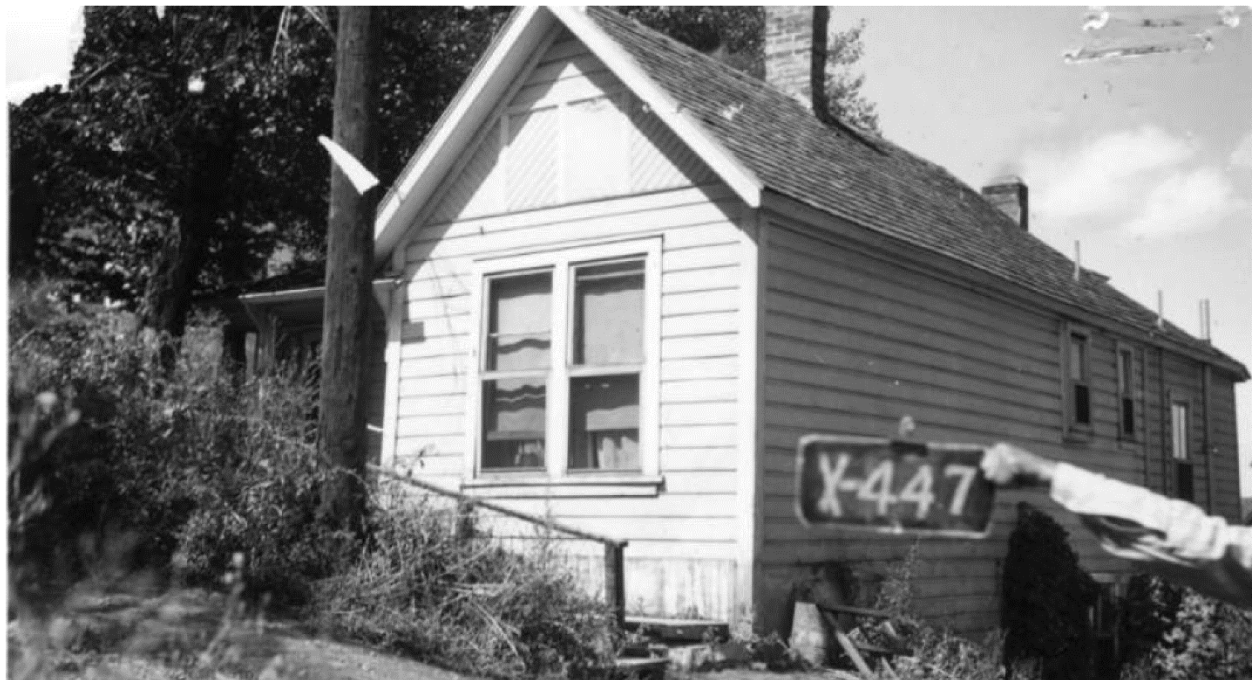
Figure 2: Oblique front view looking southwest c. 1940s
