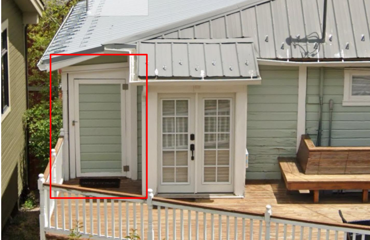
Figure 3: View of non-historic siding material to be removed.
