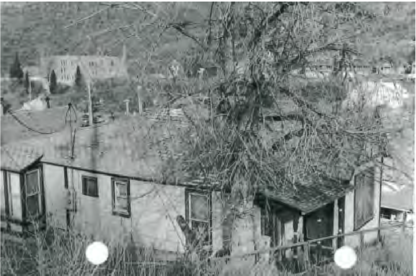
1982 Photo showing West facade & historic bay window
