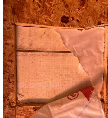
Figure 10. Inside of the Southwest c 1900 bump out. 1992 Siding material shown, no historic material remains.
