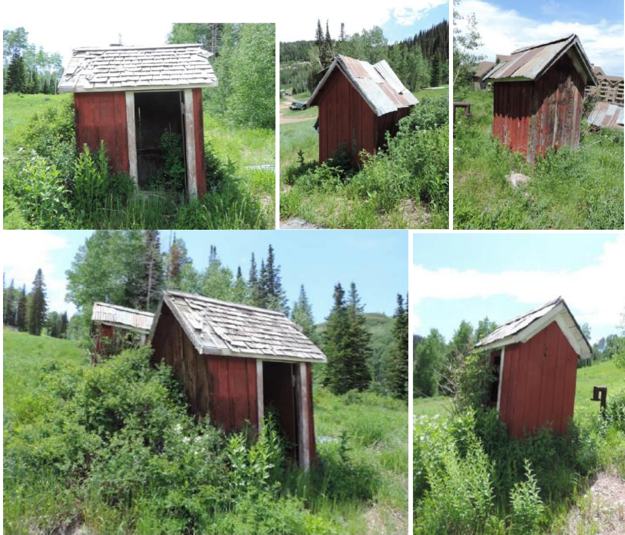
Daly-West Fire Hydrant Shacks, approx. 100 ft. Southwest of the headframe.
