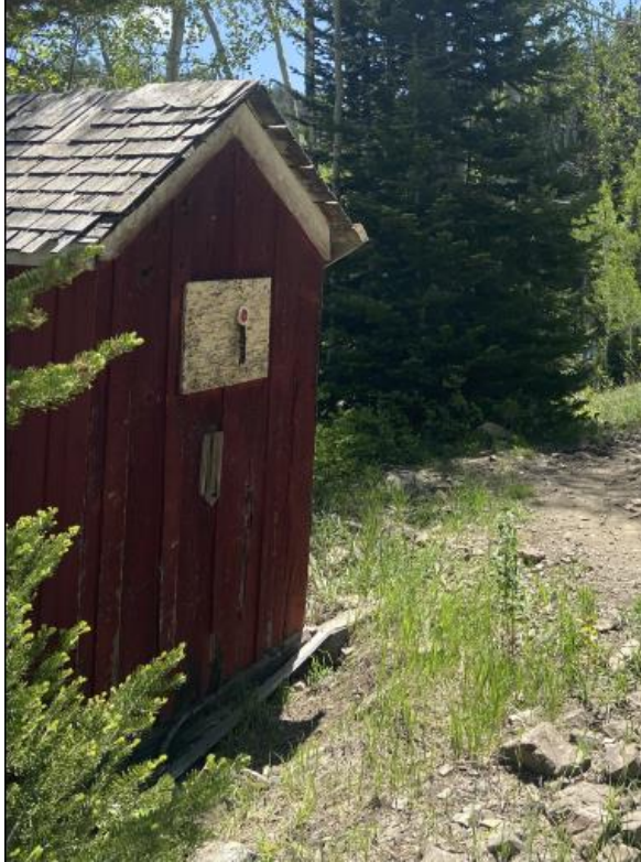
Daly West Fire Hydrant Shack #1 in its original location (will not be moved)
