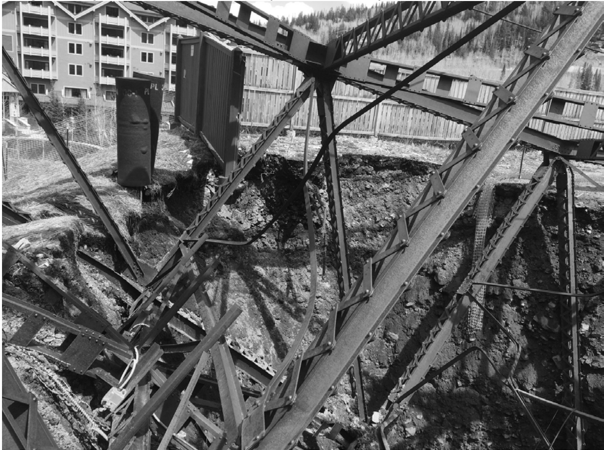
Image 5: Daly-West Mine, circ. 2015, post-shaft collapse
