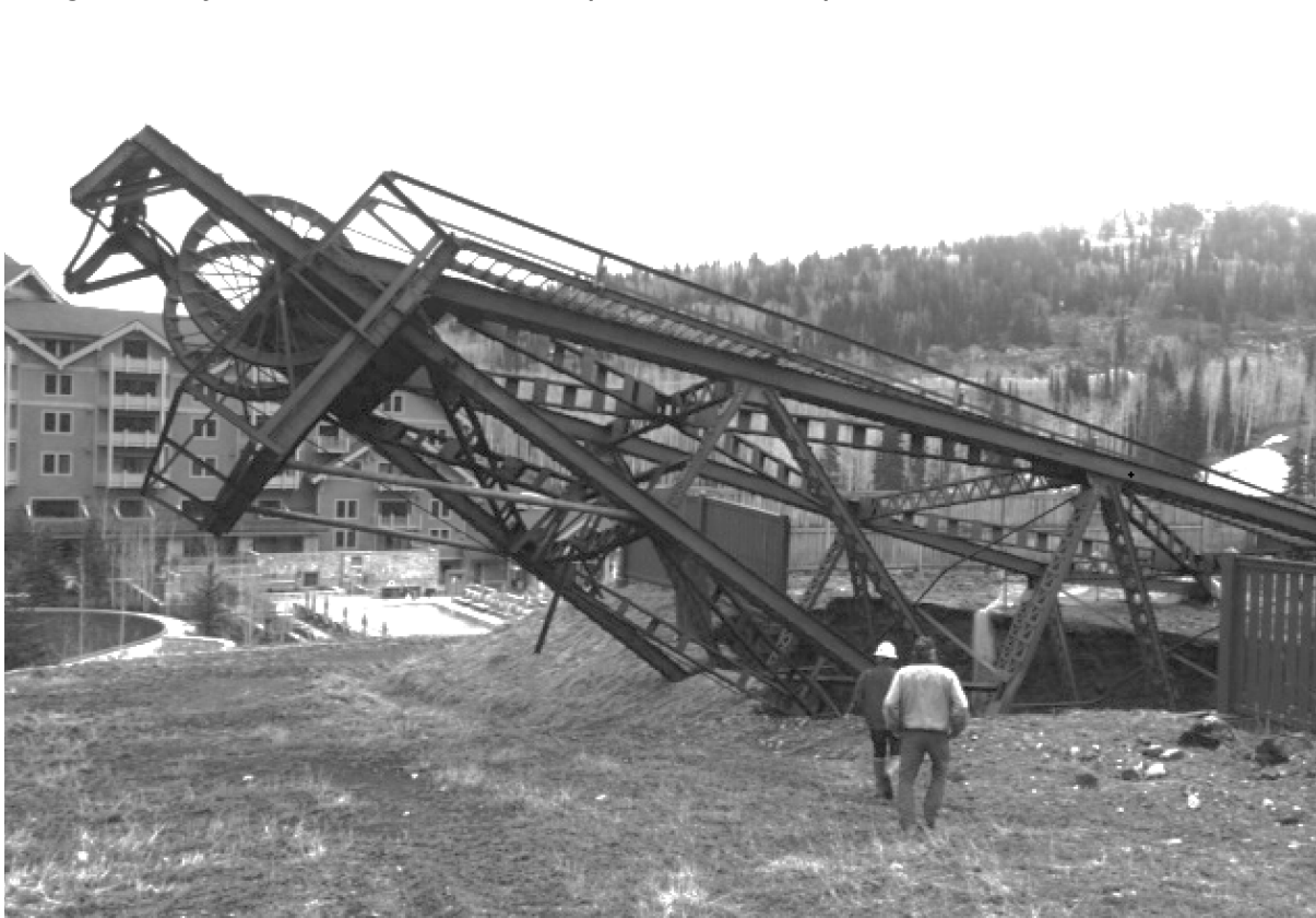
Image 4: Daly-West Mine, circ. 2015, post-shaft collapse
