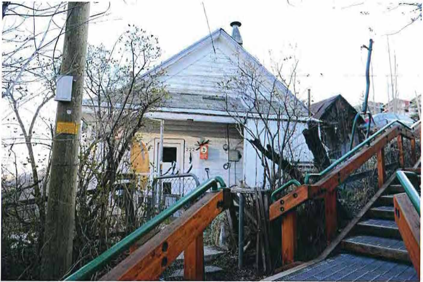
222 Sandridge Avenue looking North
