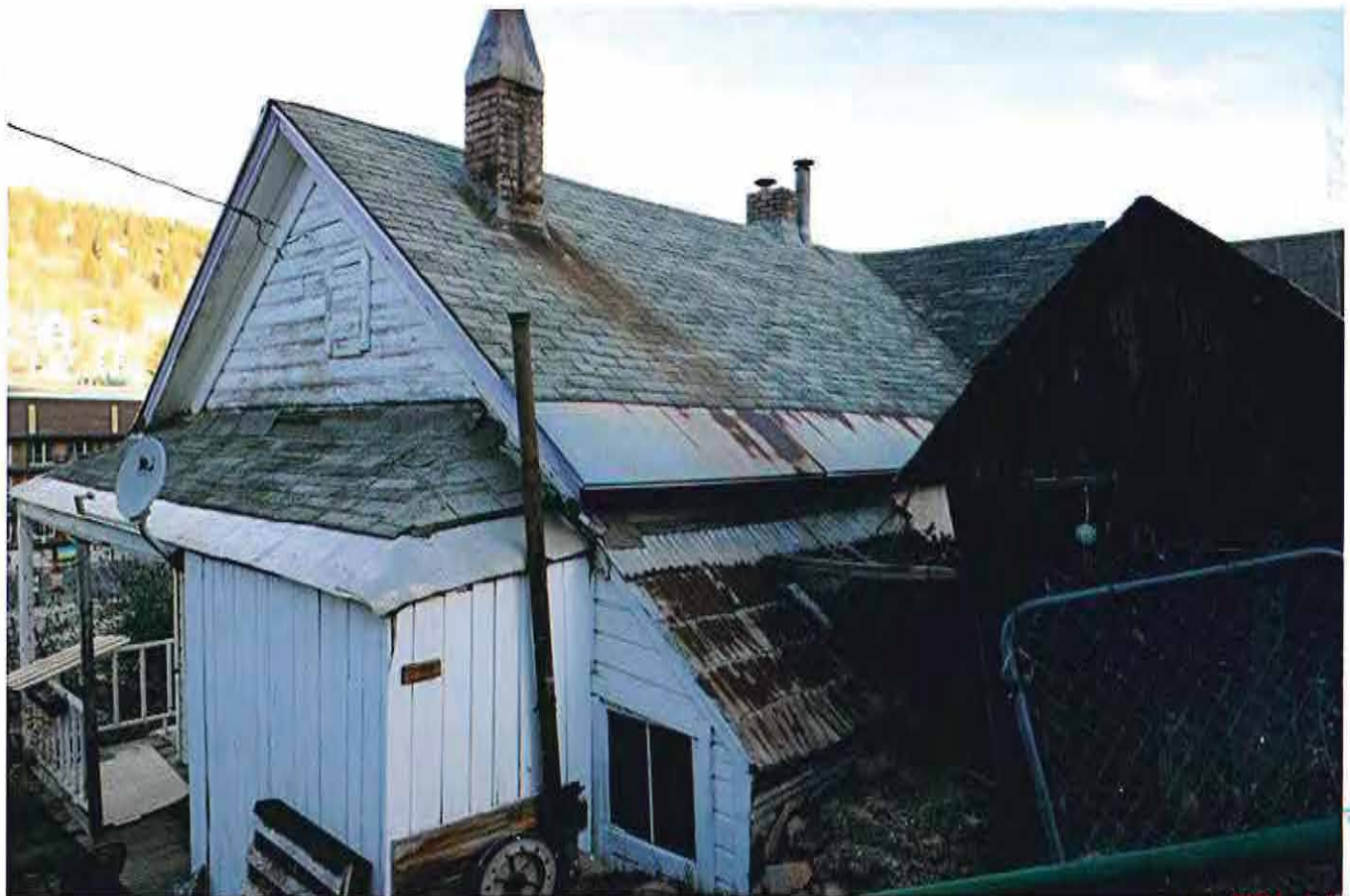
222 Sandridge Avenue looking Northwest
