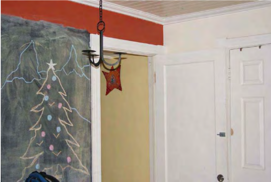
Typical ceiling trim and door casing
