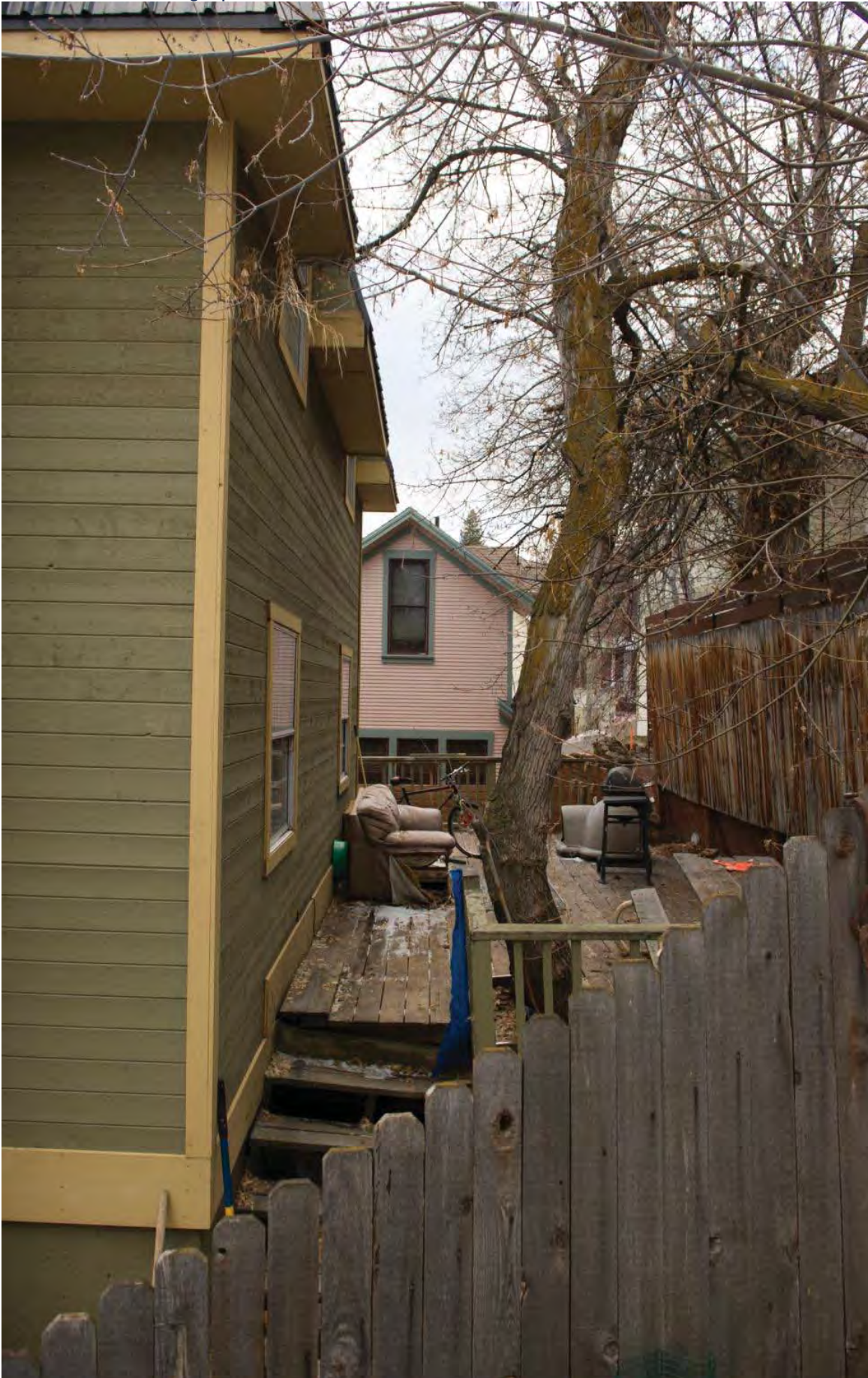
813 Woodside Avenue - looking southeasterly
