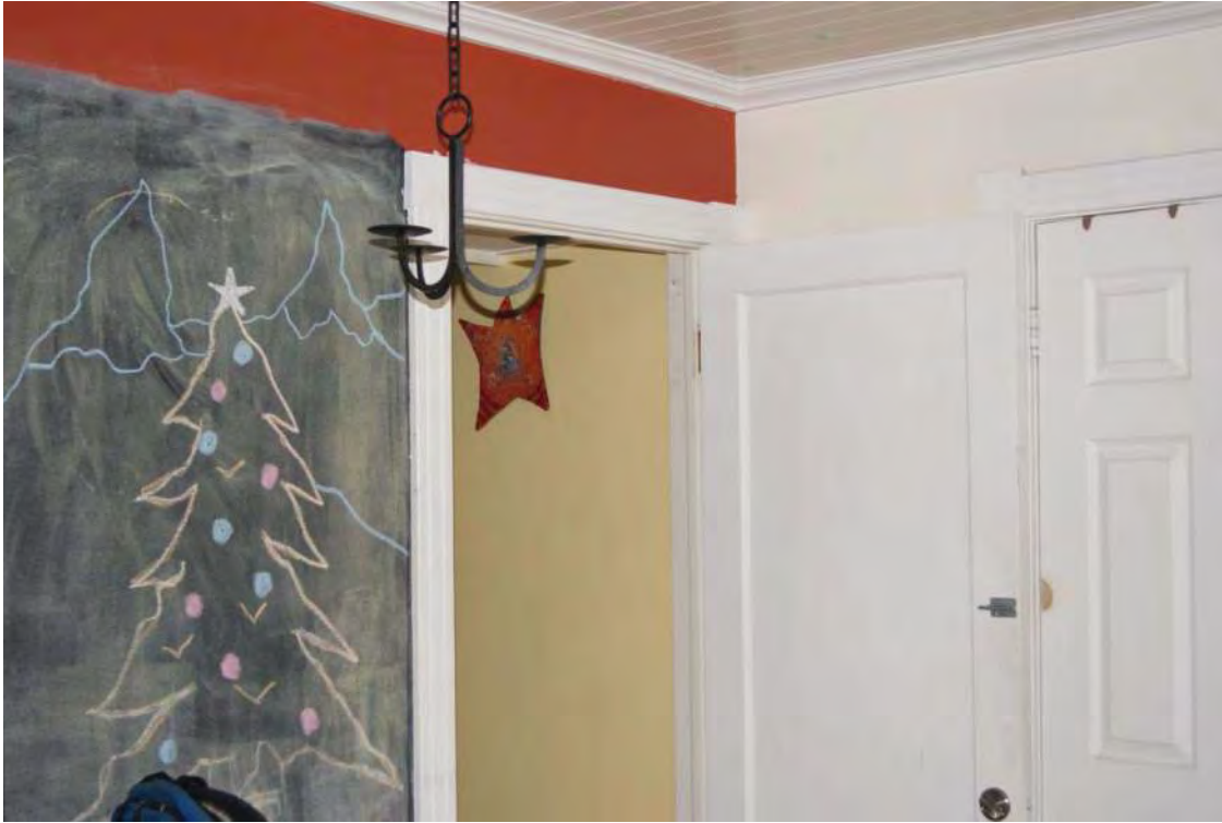
Typical ceiling trim and door casing
