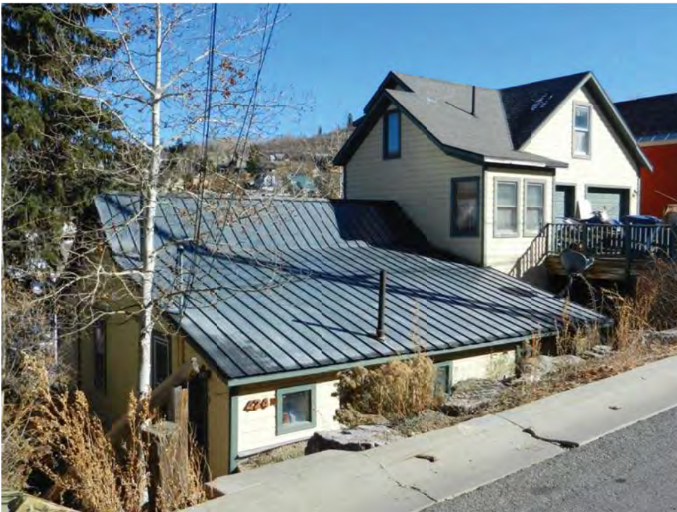
424 Woodside Avenue. Northwest oblique. November 2013.
