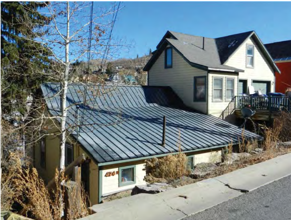
424 Woodside Avenue. Northwest oblique. November 2013.
