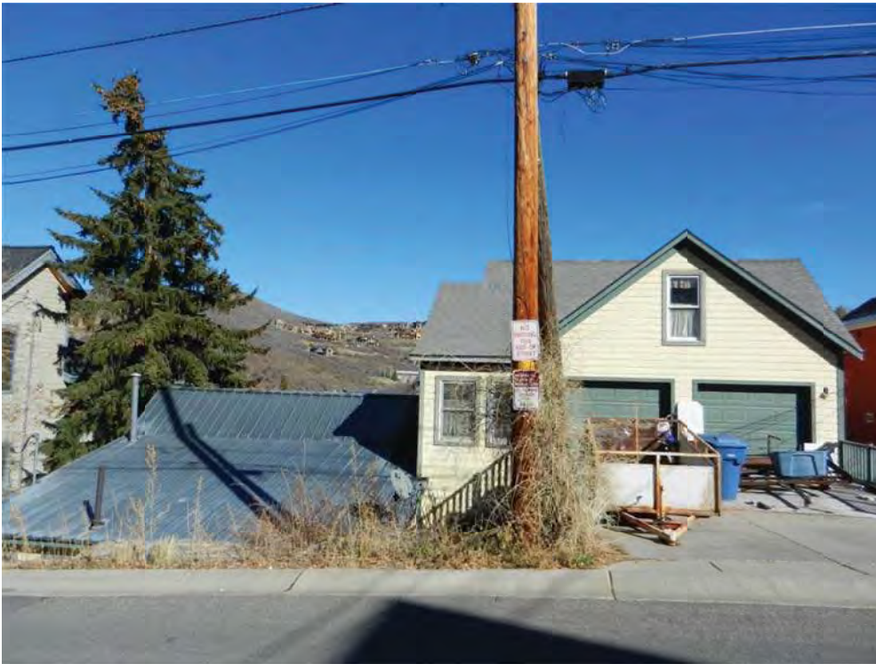
424 Woodside Avenue. West elevation. November 2013.
