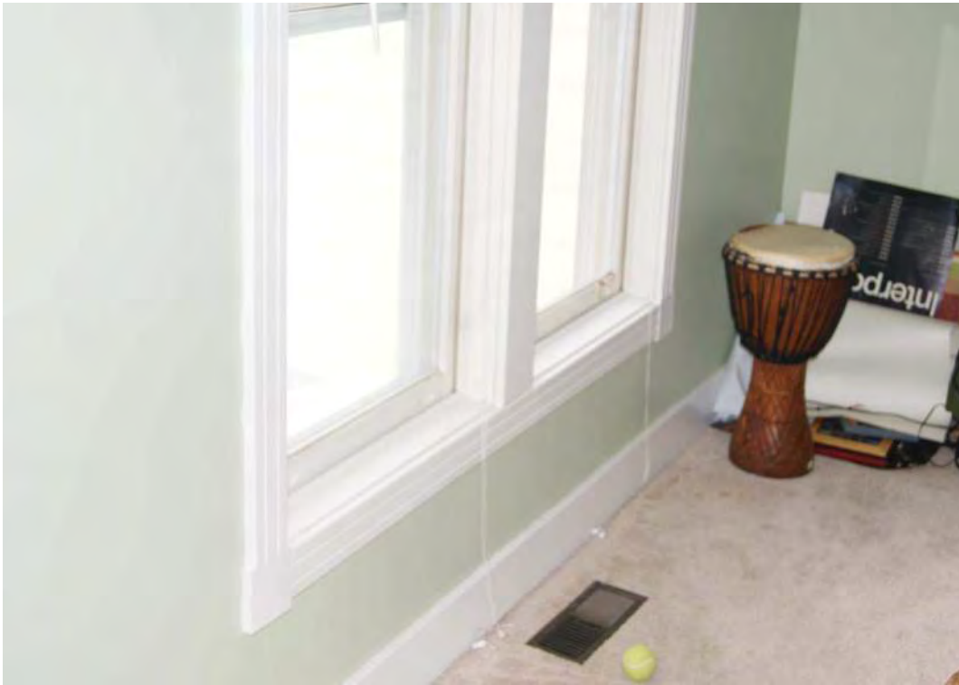
Typical base and window casing
