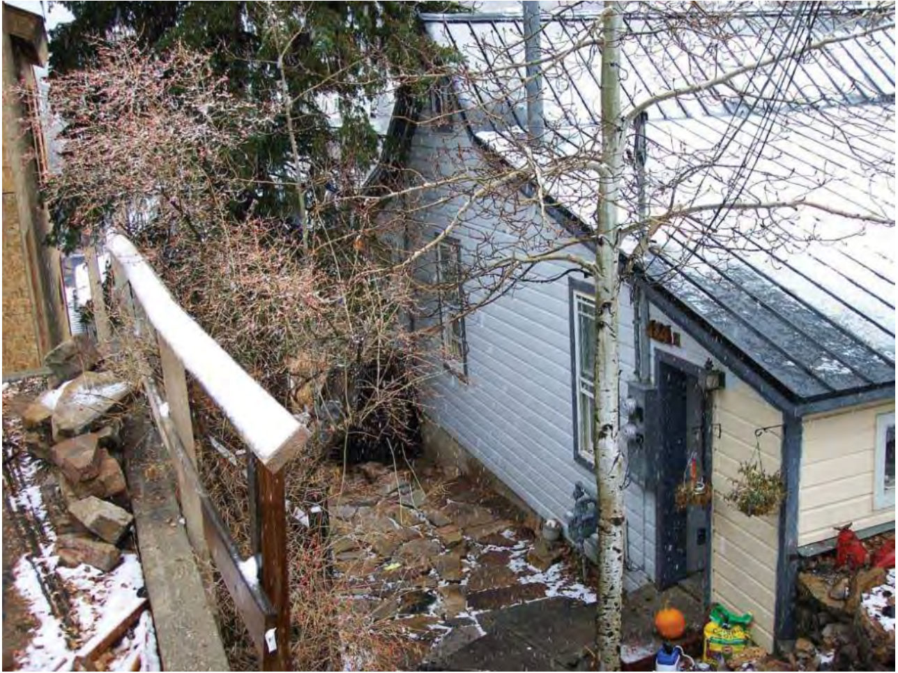
Roof looking southeast
