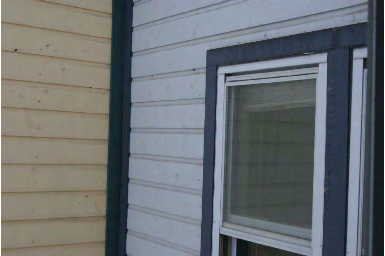
Wood aluminum clad window- typical
