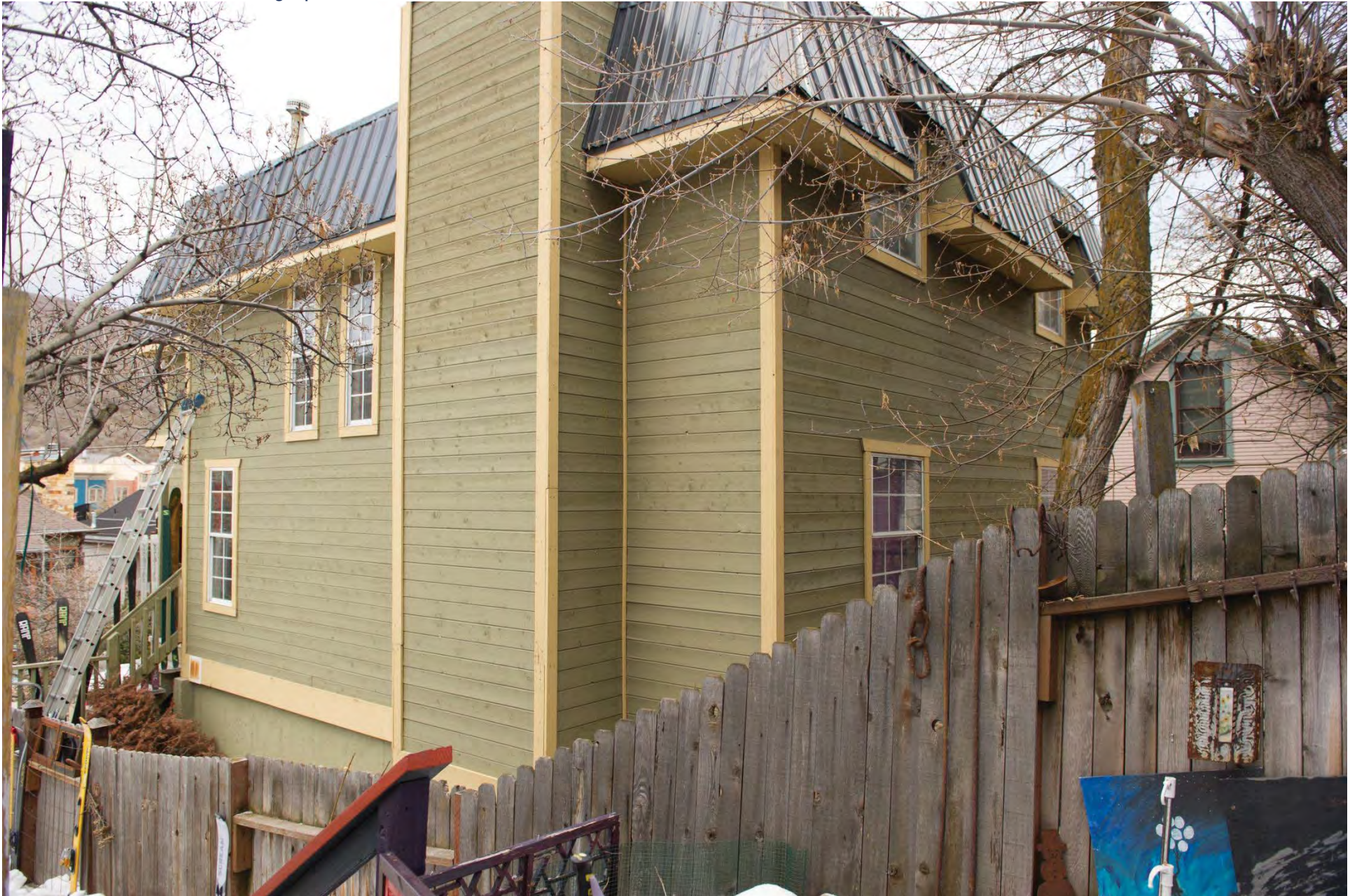
813 Woodside Avenue - looking easterly
