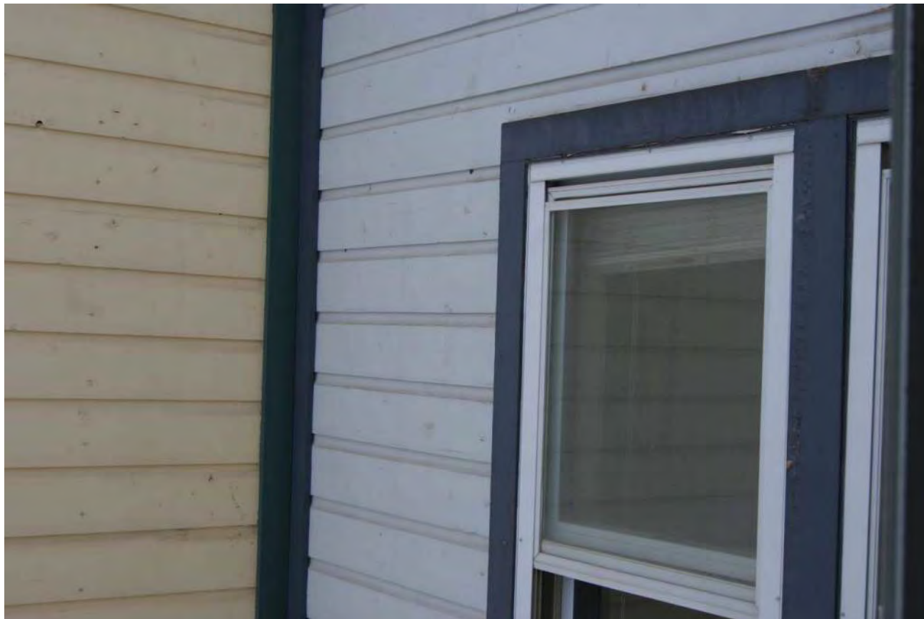
Wood aluminum clad window- typical
