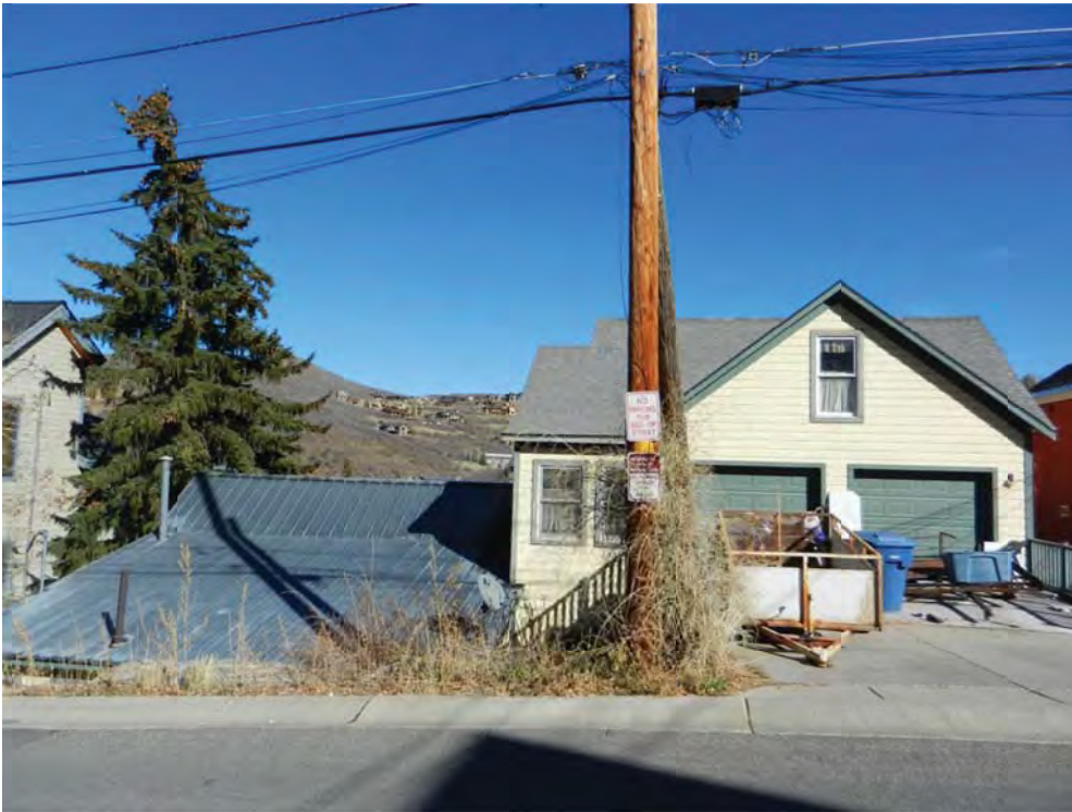
424 Woodside Avenue. West elevation. November 2013.
