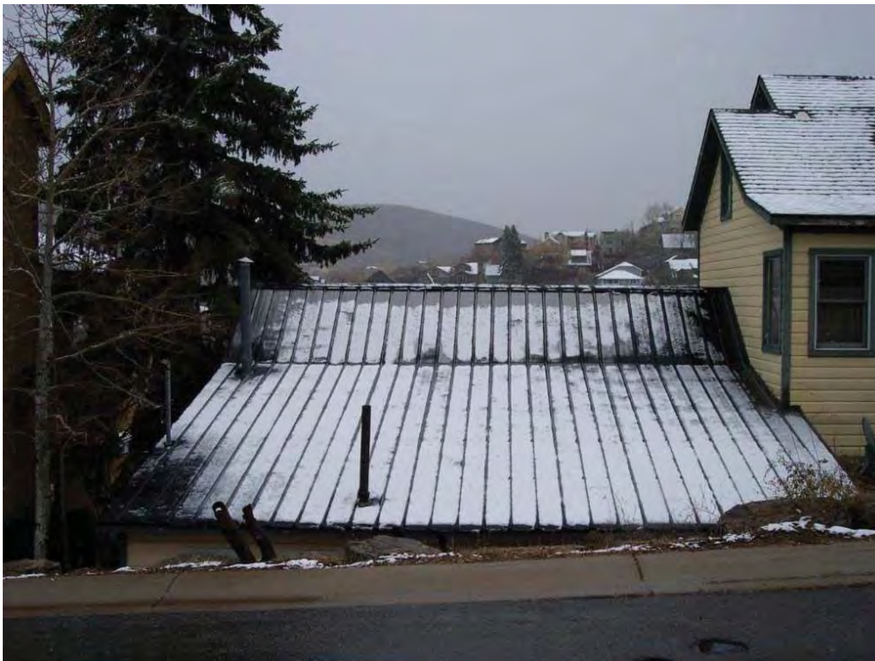
Roof looking east
