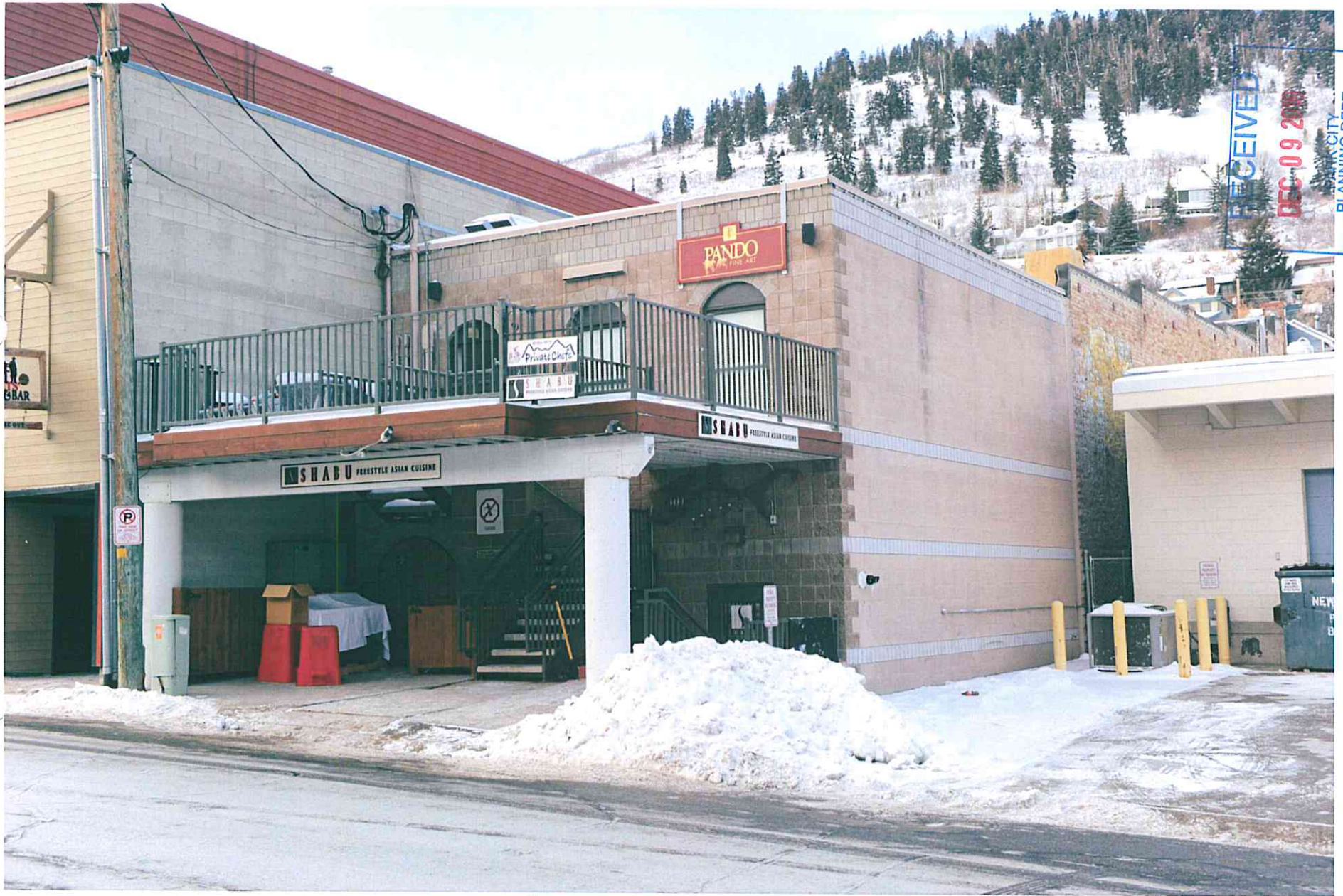
442/444 Main Street – looking southwest
