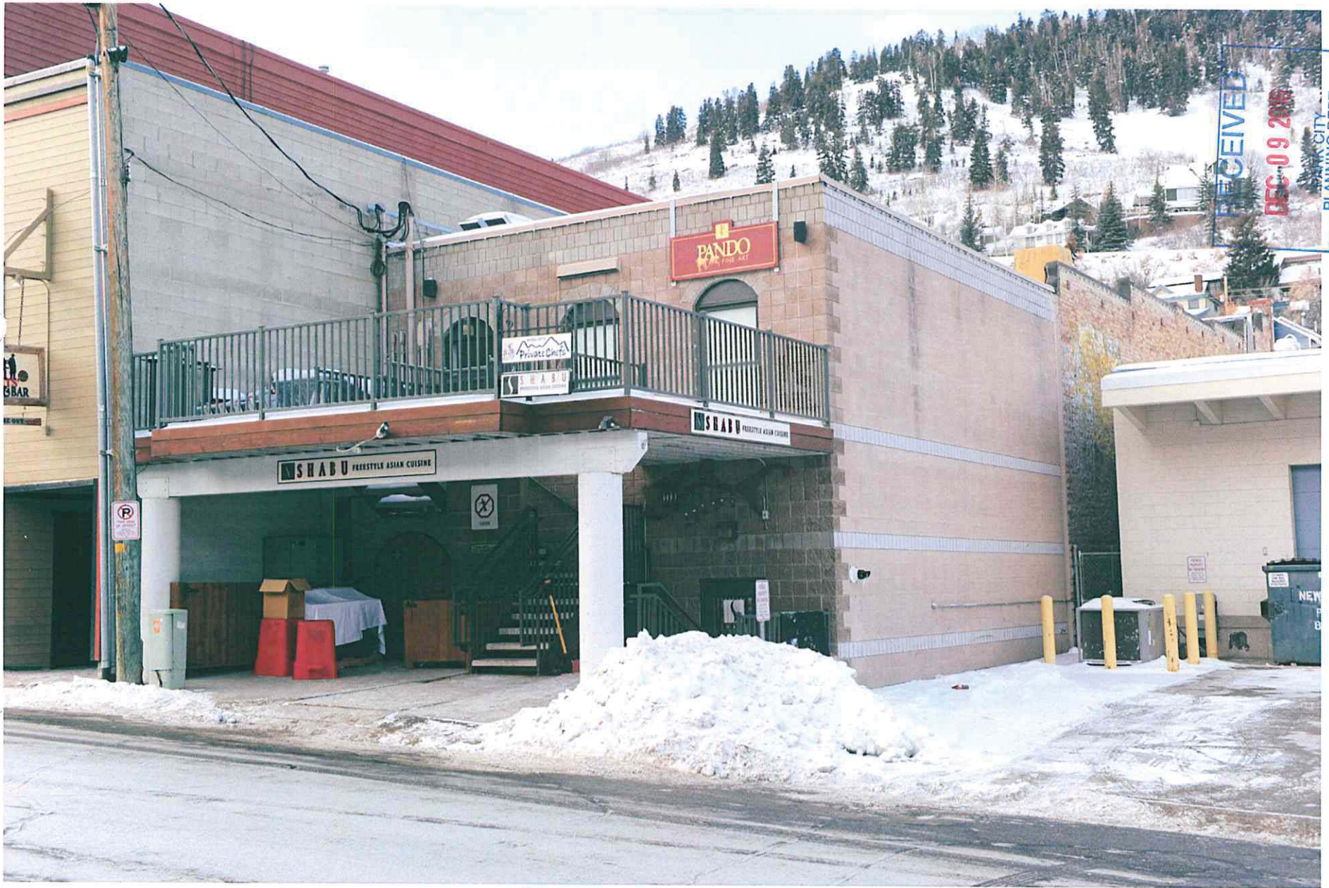
442/444 Main Street – looking southwest
