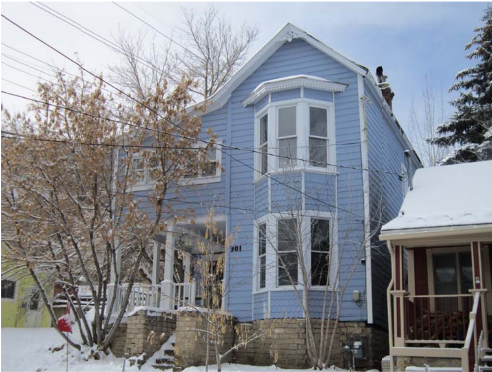
901 Woodside Avenue. Northeast oblique. November 2013.
