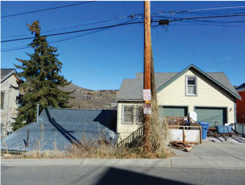
424 Woodside Avenue. West elevation. November 2013.
