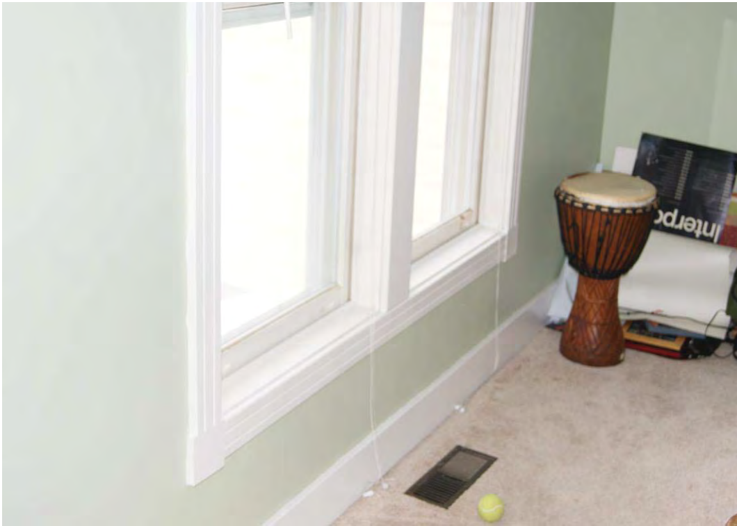
Typical base and window casing
