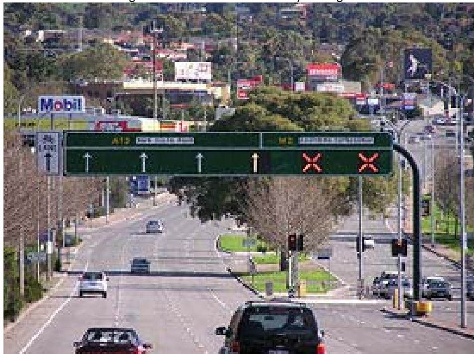
Figure 4: Direction Control Gantry and Lights
