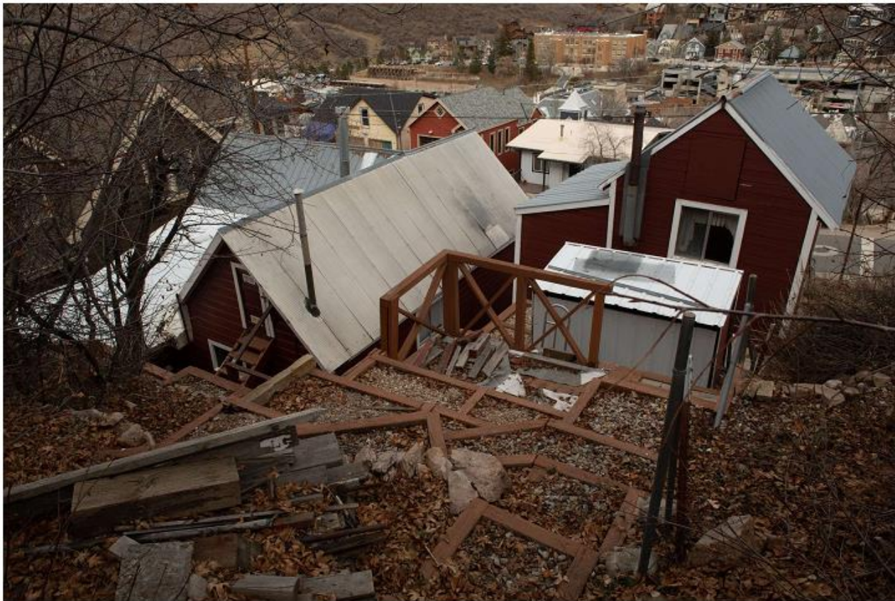
405 Woodside Avenue - rear - looking northeasterly
