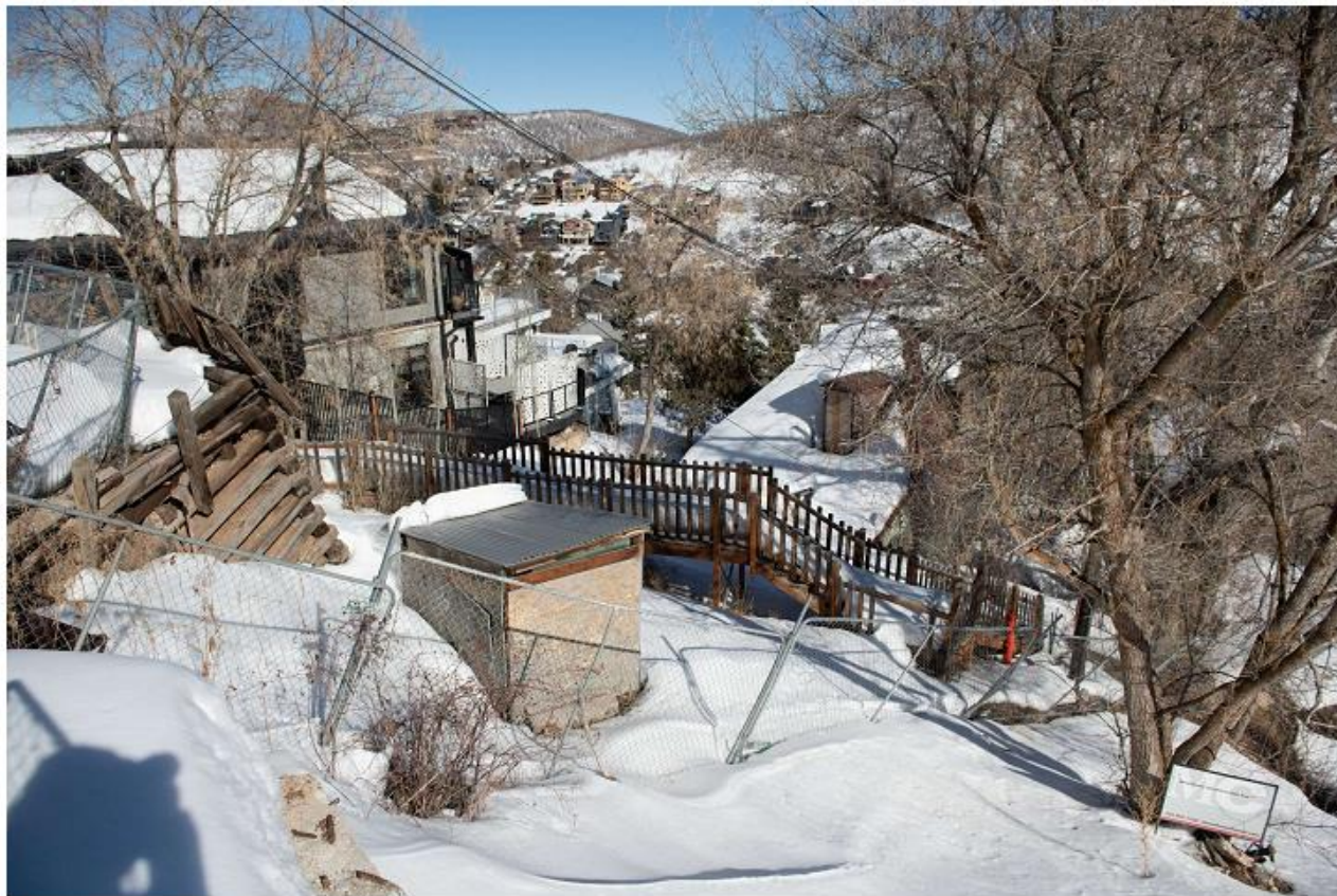
115 Sampson Ave - front - looking northeasterly
