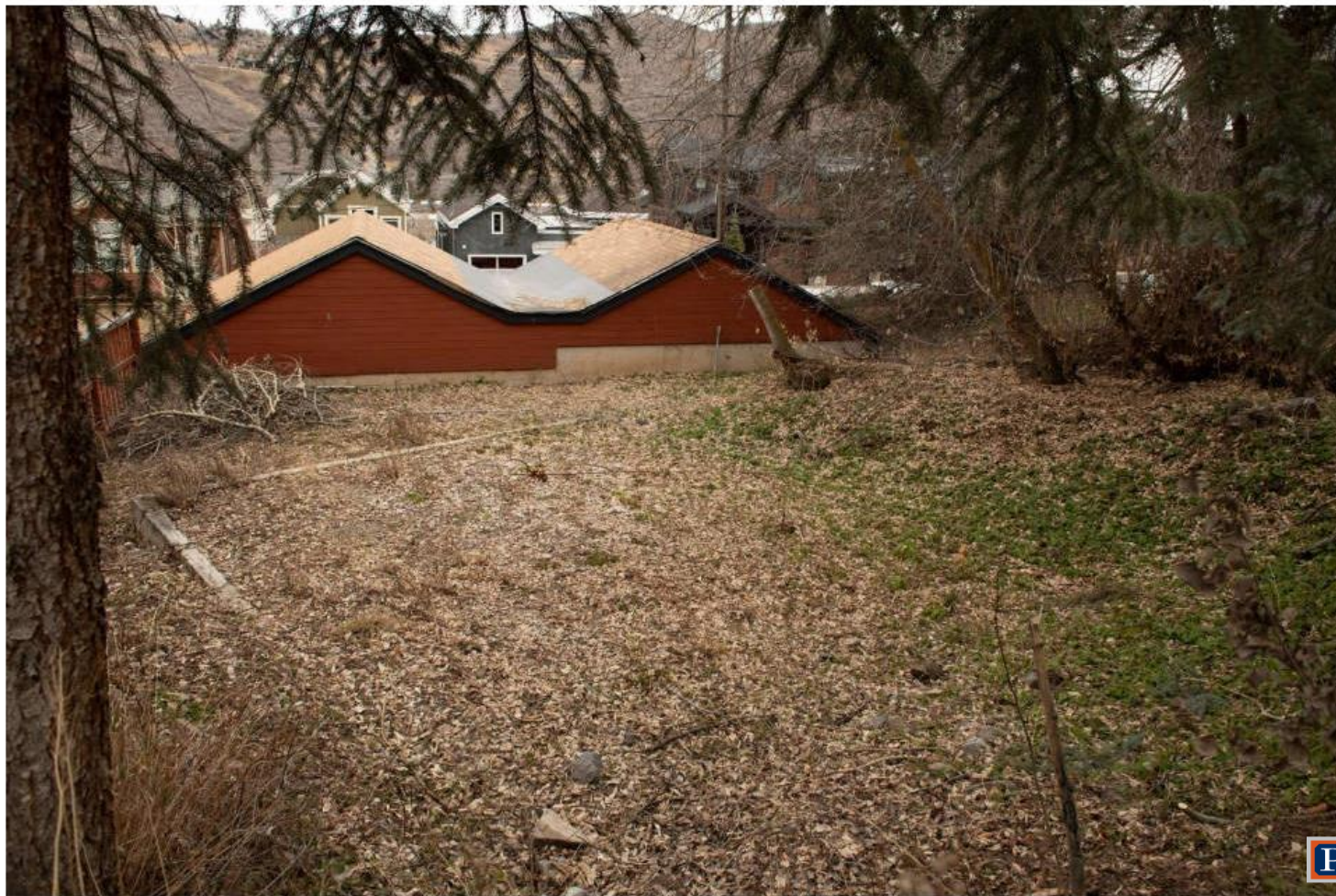
949 Empire Avenue - rear - looking northeasterly
