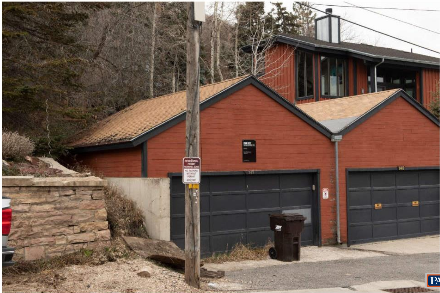
949 Empire Avenue - front - looking westerly
