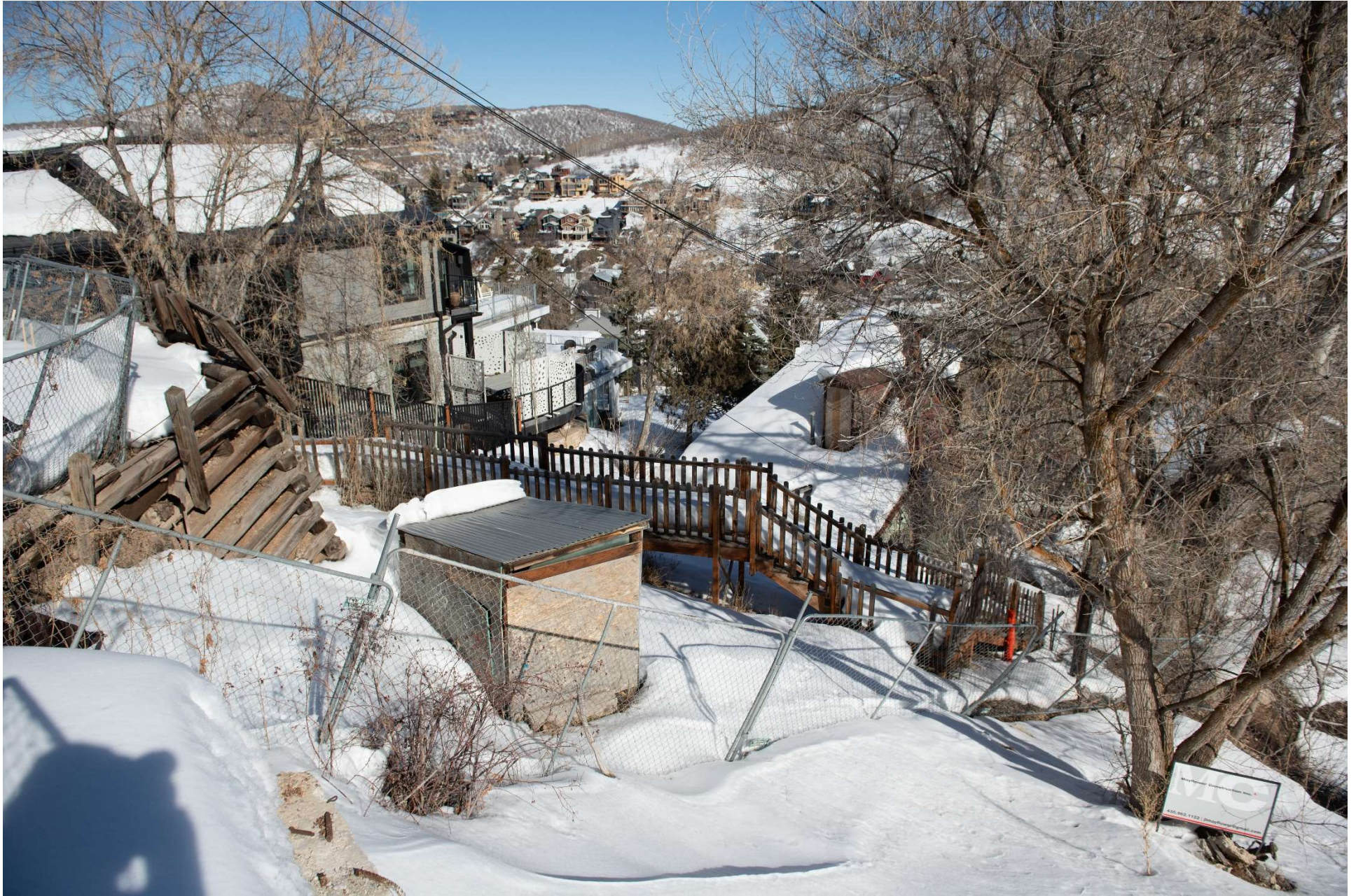
115 Sampson Ave - front - looking northeasterly
