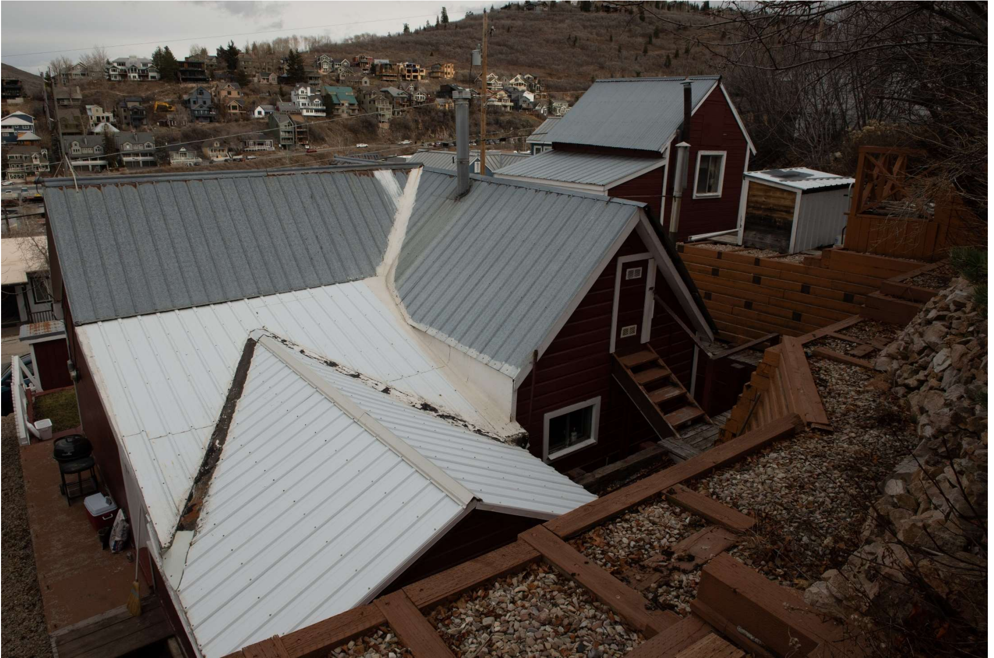
405 Woodside Avenue - rear - looking easterly
