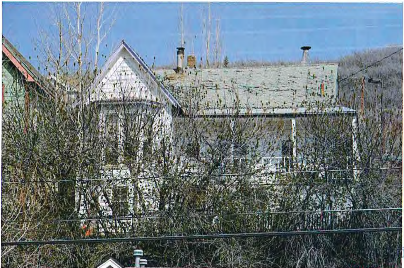
222 Sandridge Avenue looking East
