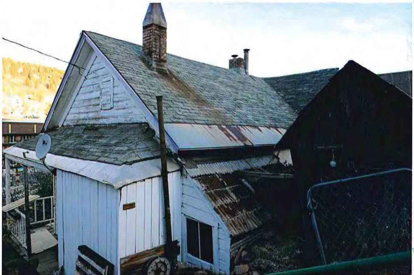
222 Sandridge Avenue looking Northwest
