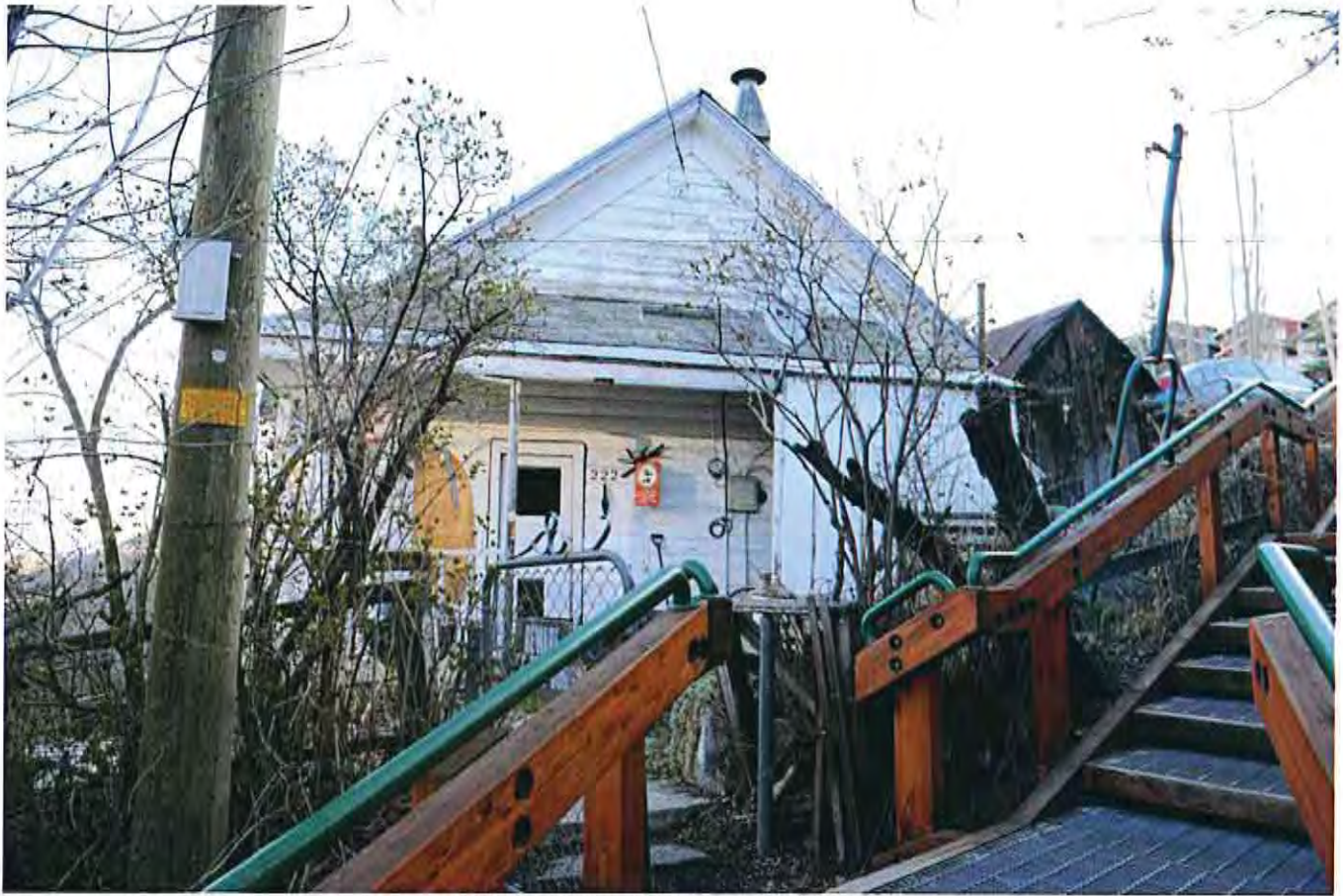
222 Sandridge Avenue looking North
