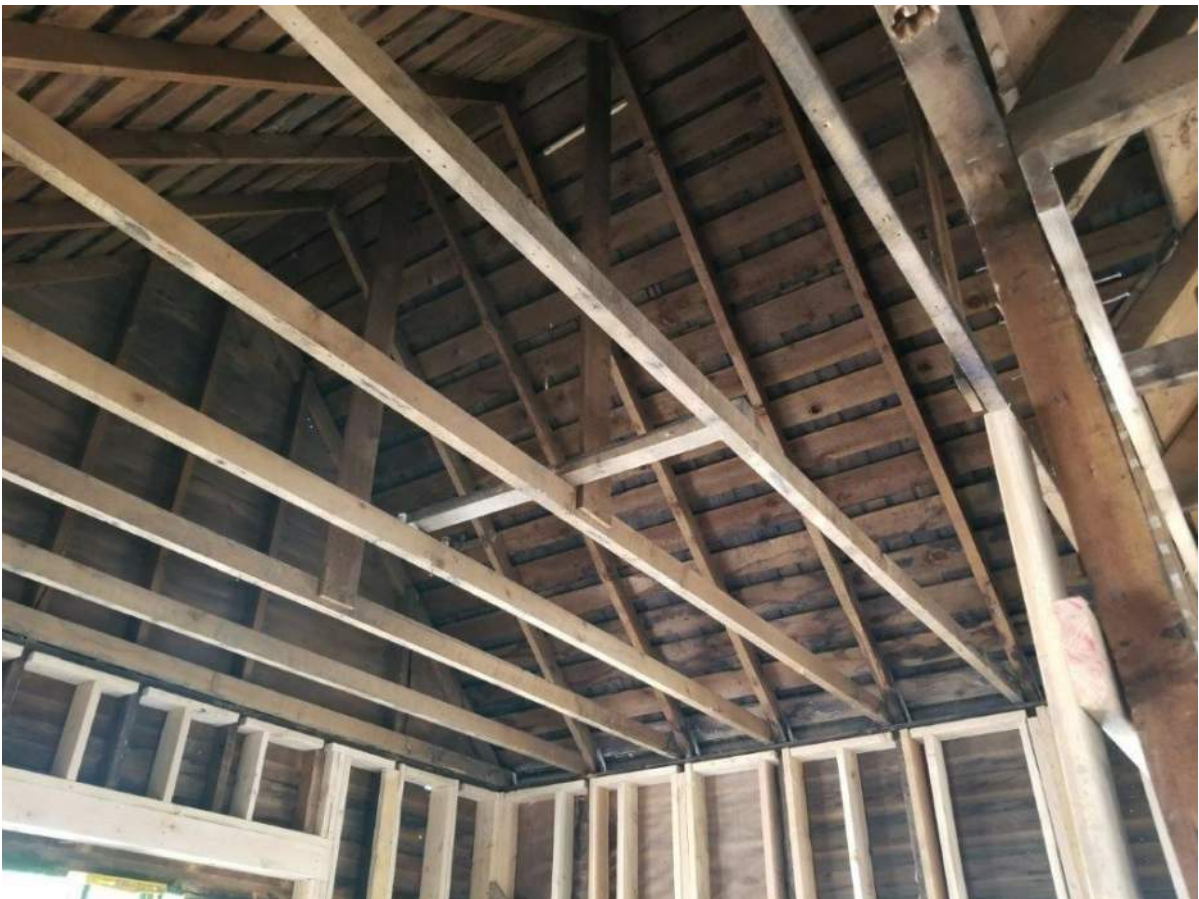
Below: Roof structure of the historic house. Note the intersection of the gable ell to the side-gable of the original hall-parlor house form in the upper right hand corner.
