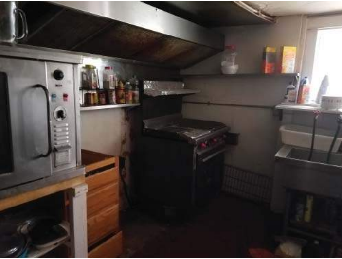
71 - L1 - Kitchen - NW Wall
