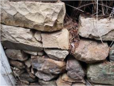
16 - West Retaining Wall Composition
