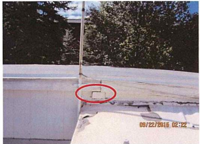
Photo 8 Note structural beam. Refer to photo 9
