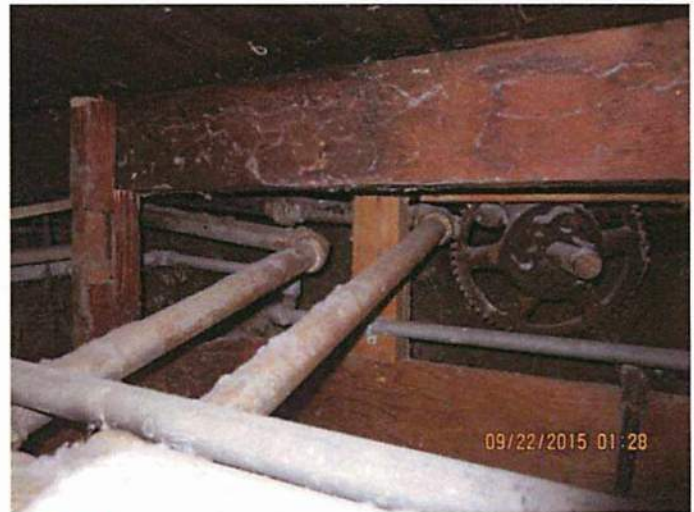
Photo 4 Unsecured gas lines, unknown valves that are not properly maintained or marked
