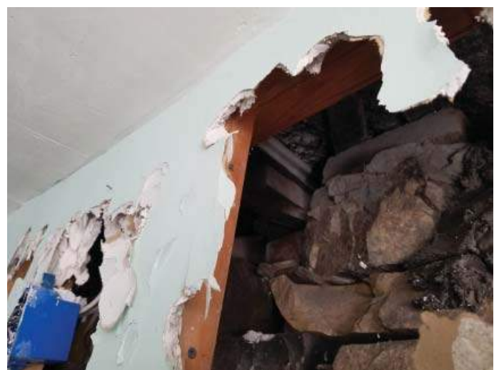
57 - L0 - S. side of Central Stone Wall
