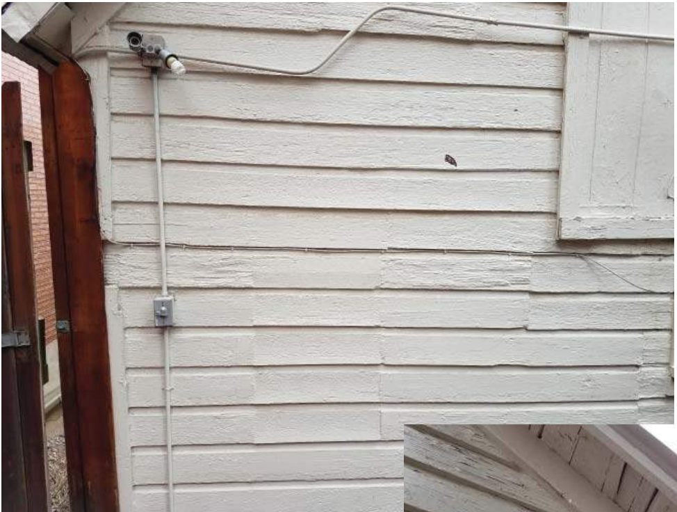
22 - Patched Siding on Wall
