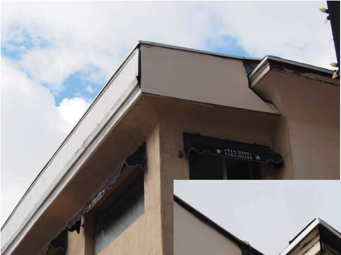
31 - NE Eave Detail
