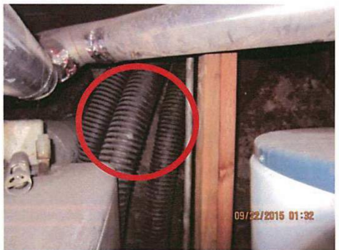
Photo 6 A drainage system was improperly installed and permitted to drain directly on top of the dirt floor causing decay, mold and erosion
