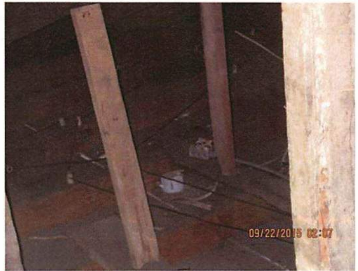
Photo 18 General inspections noted that the knob and tube is most likely active
