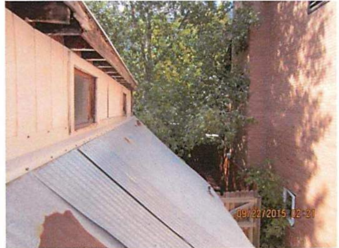
Photo 31 Roof shows sign of decay and rot damage, soffit and fascia are missing, possible location of water infiltration
