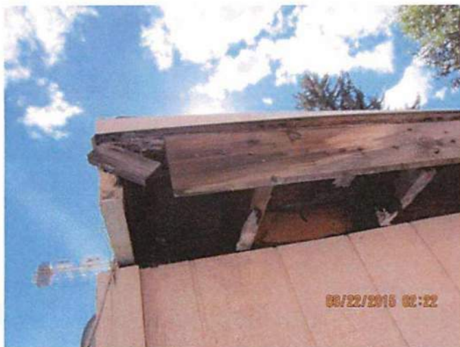
Photo 32 Roof shows sign of decay and rot damage, soffit and fascia are missing, possible location of water infiltration
