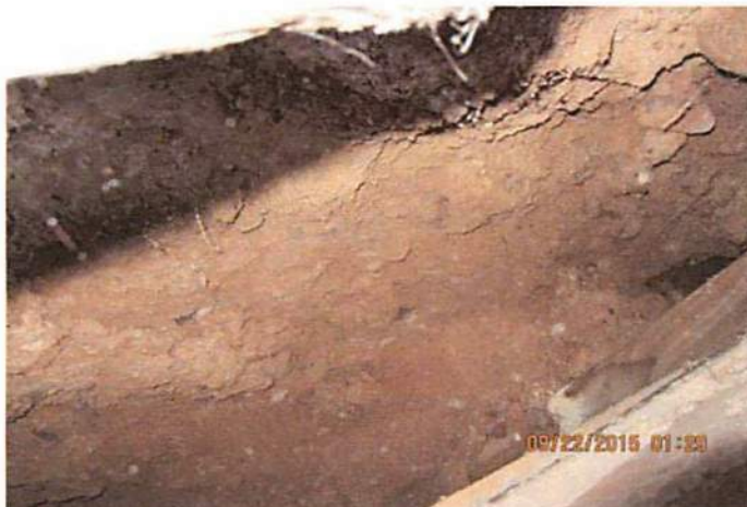
Photo 9 Back side of photo 8
