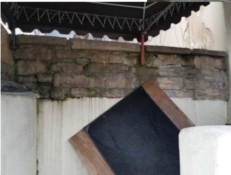
27 - East Retaining Wall
