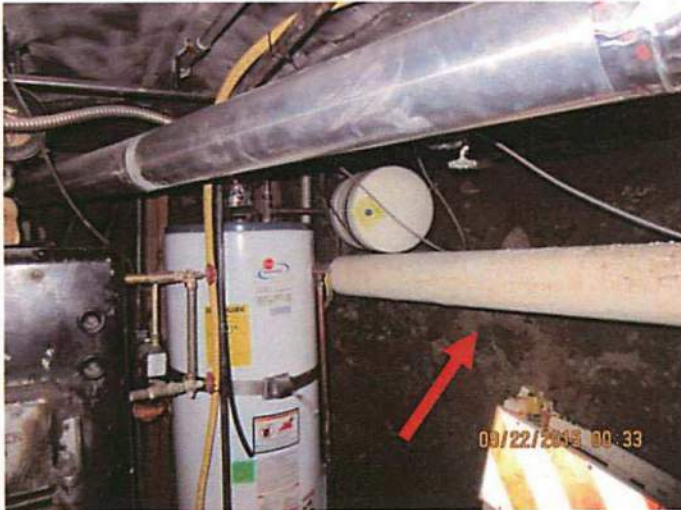
Photo 1 The structure has no concrete or stable foundation. The foundation consists of rubble, dirt and loose stone matter.
