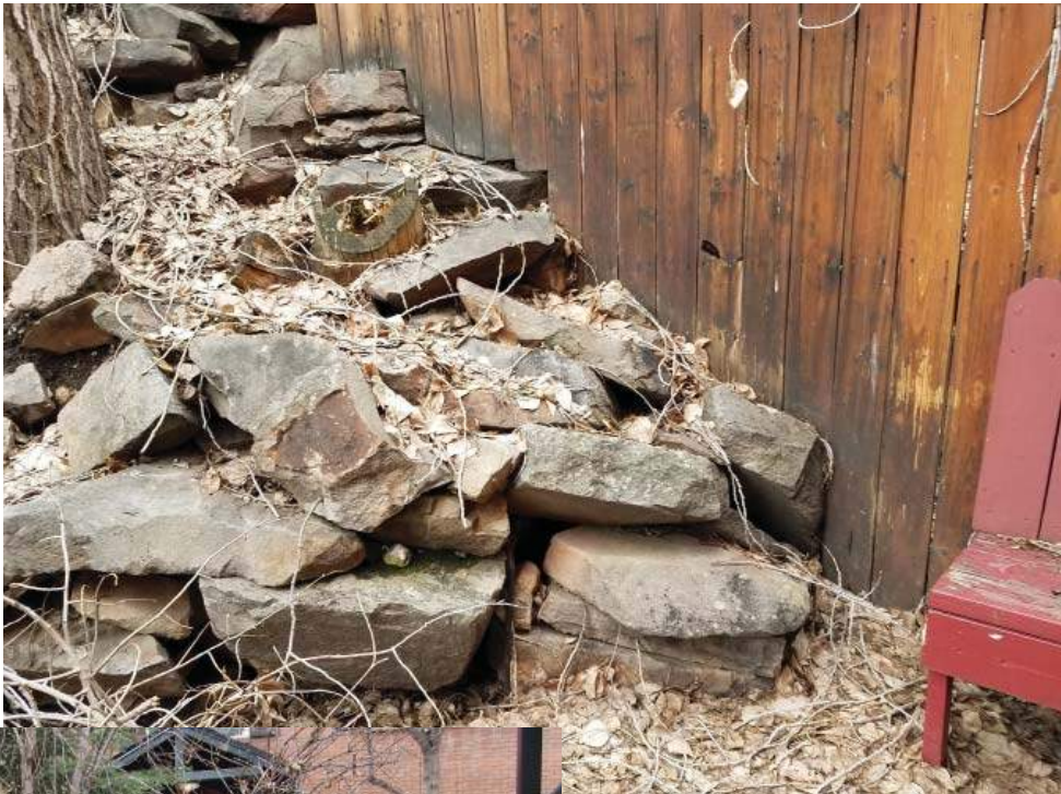
16 - West Retaining Wall Composition
