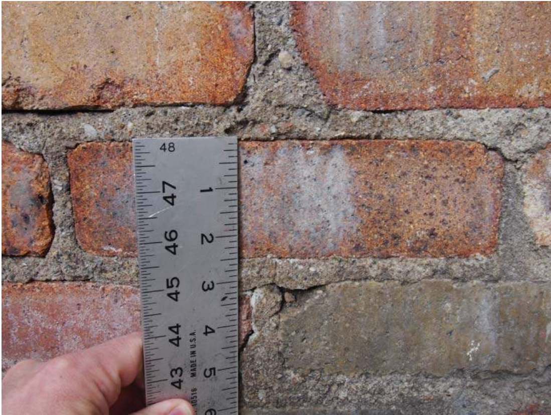
29 - Chimney Brick Height
