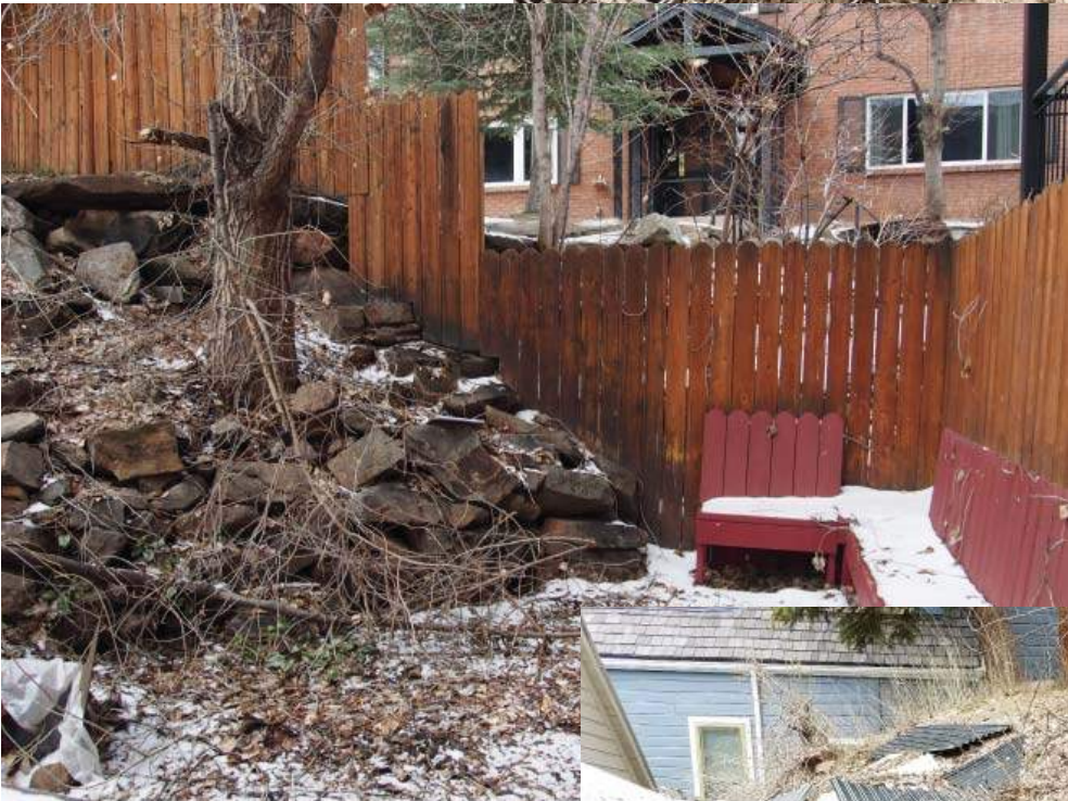
17 - West Deck & Retaining Wall
