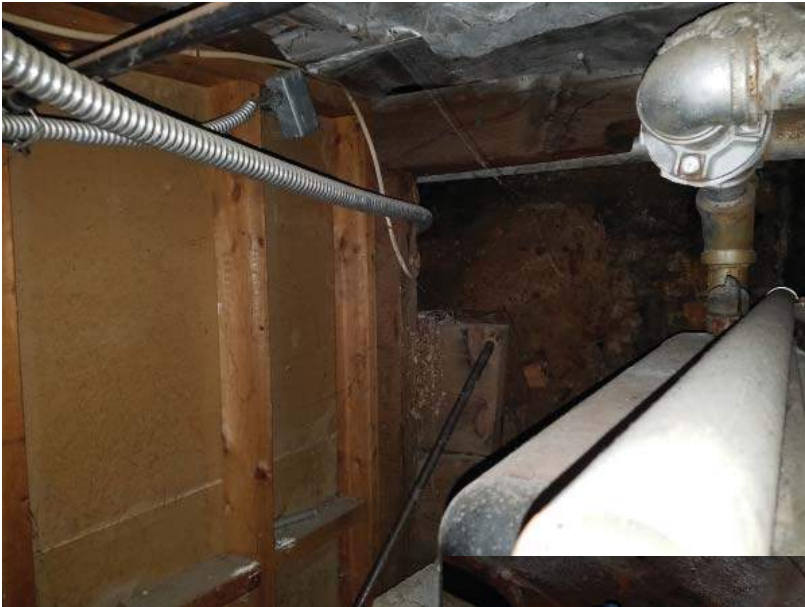
58 - L0 - South Foundation in Mech.
