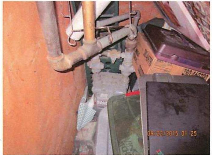
Photo 2 Gas meter is located in a hidden room with possible improper connections to the building. The room is located in the front of the deli between the entry doors
