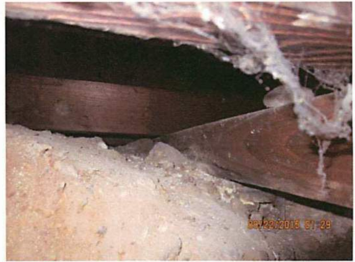
Photo 20 Floor joist are bearing directly on top of soils. This is not permitted by code
