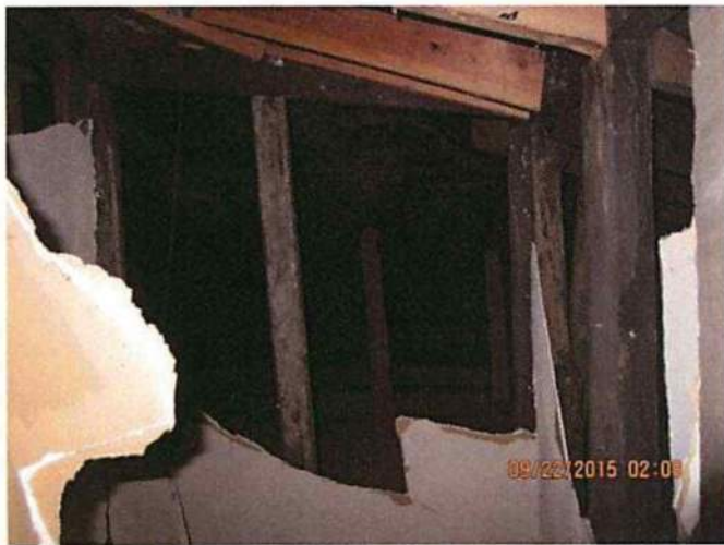
Photo 7 Roof has been repaired, support members not properly installed. Engineer to evaluate and justify
