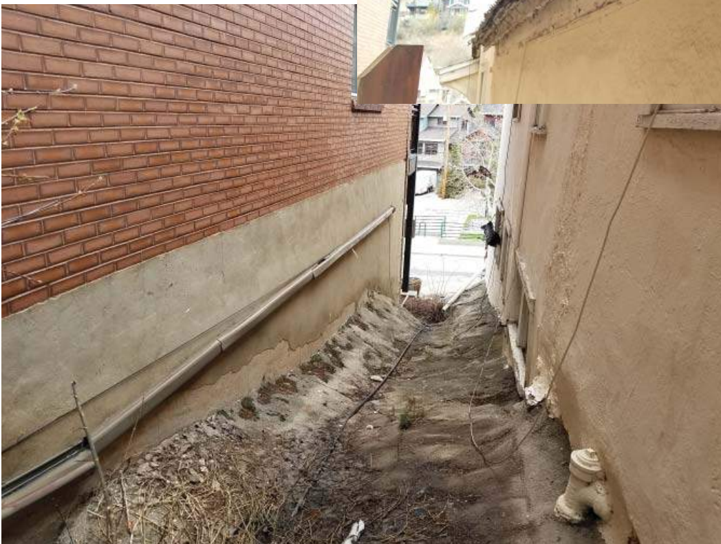
10 - North Concrete Site Detail
