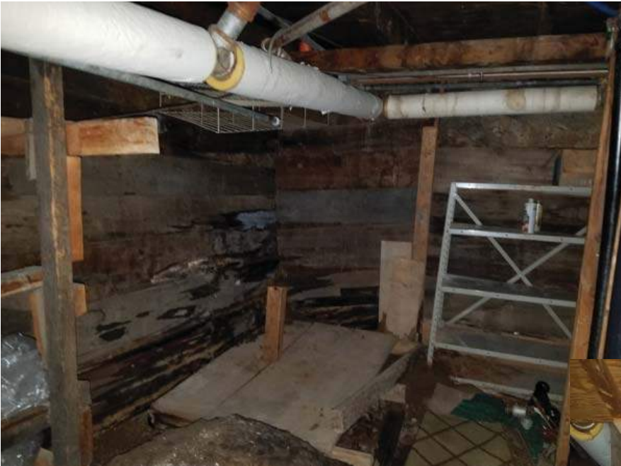
61 - L0 - Wood Shoring
