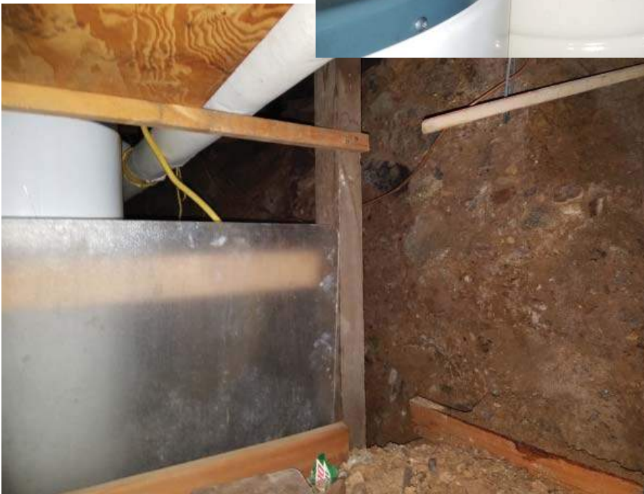
60 - L0 - Dirt Foundation
