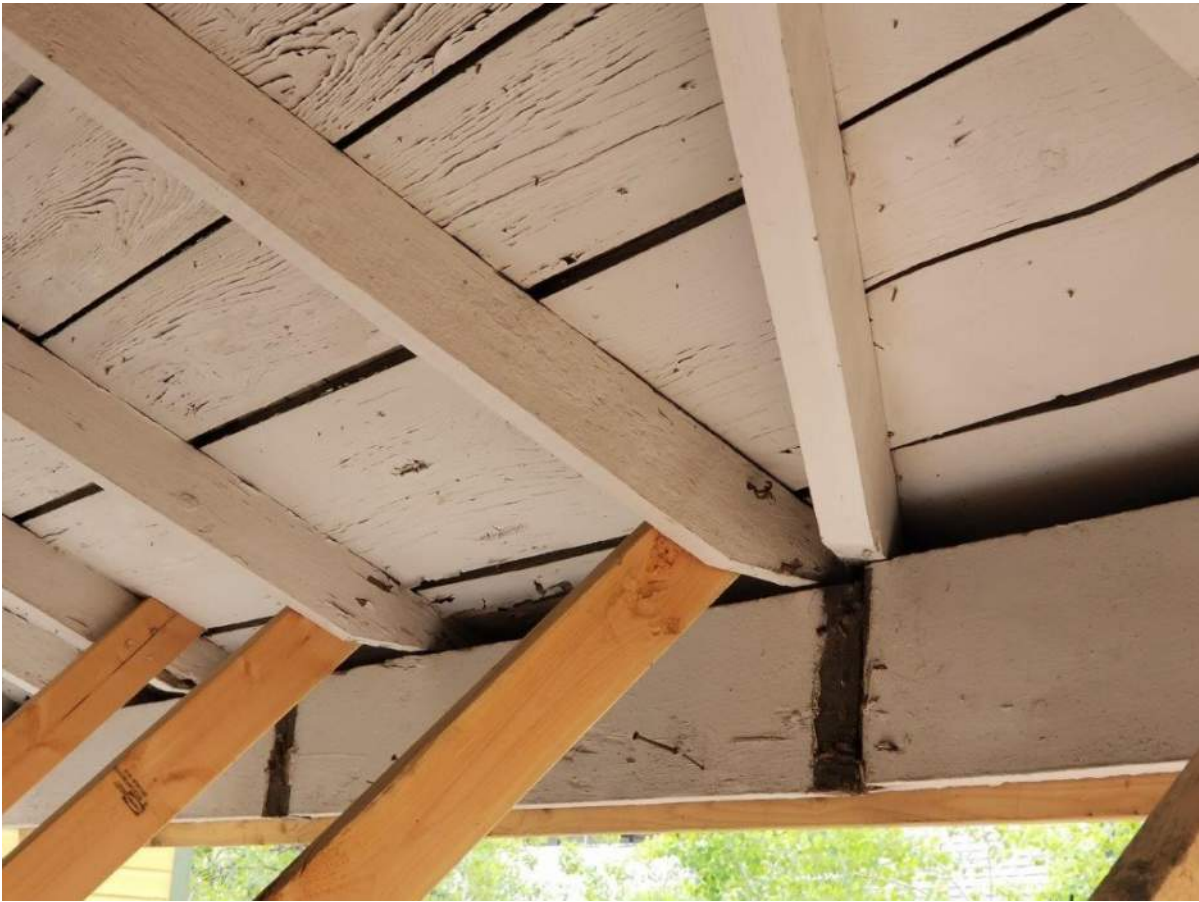
Above: Porch roof.
