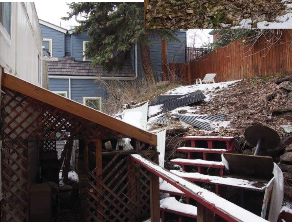
15 - West Site Conditions
