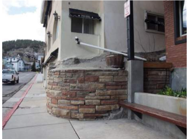
Retaining Wall #2 (North Side of Façade)
