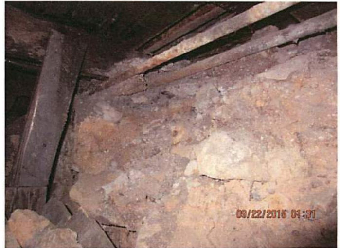
Photo 6 Water lines used for the heating of the building are damaged by decay and deterioration. Erosion and sloughing of the rubble foundation. Severe stability concerns for the structure
