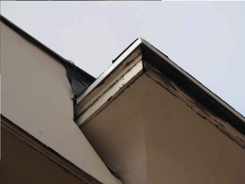
32 - NE Eave Detail
