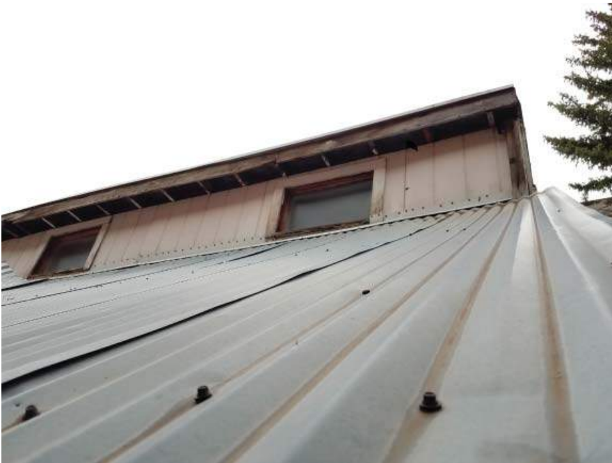
8 - North Corrugated Roofing
