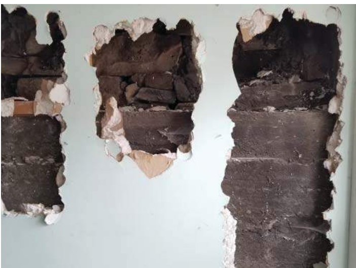
56 - L0 - Detail of Wall
