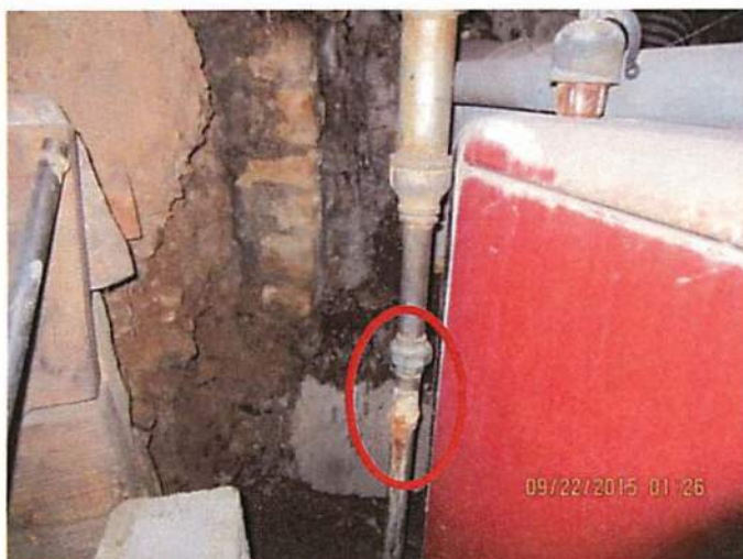
Photo 9 Gas line shows decay and deterioration needs to be shut off ASAP
