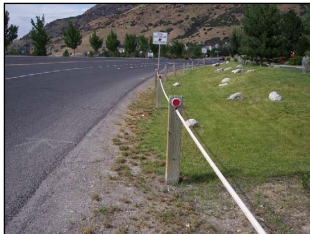
Figure 2 – Transparent Fencing
