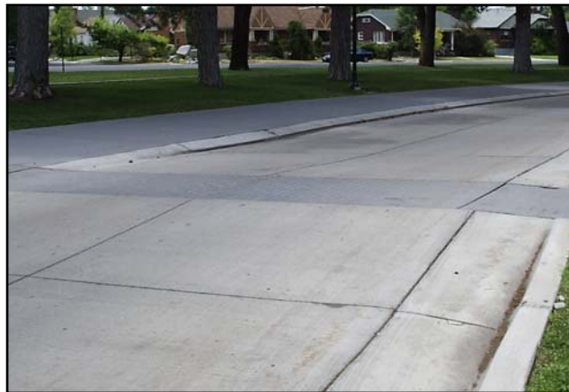
Figure 3 – Raised Crosswalk
