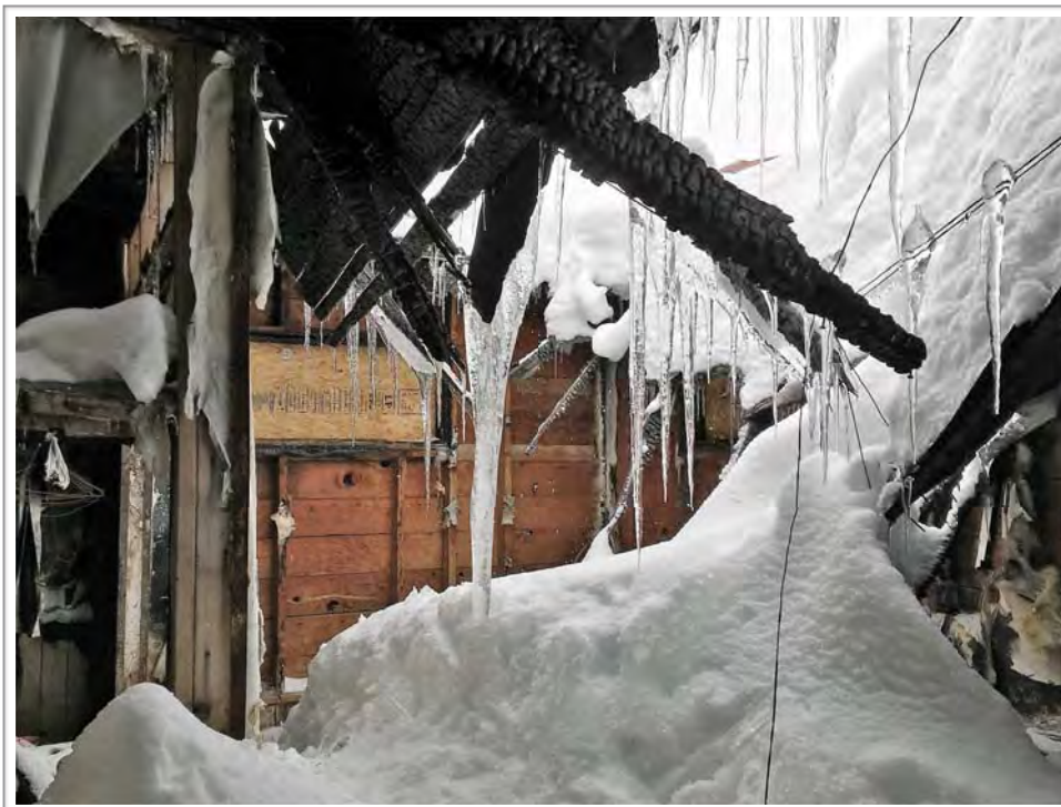
Photo #14: Fire Damage @ Rear Addition
