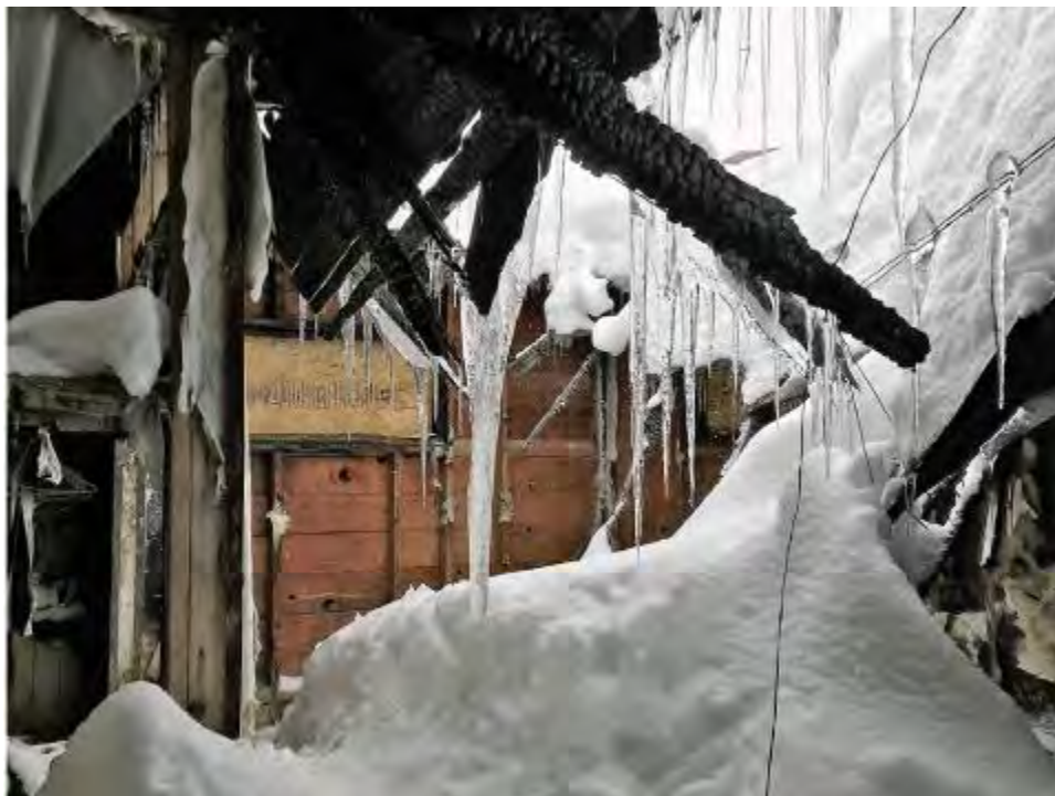
Photo of interior of c.1969 addition and historic wall of the house. Due to the hole in the roof of the c.1969 addition, the back portion of the historic house and the c.1969 addition have been largely exposed to the elements.
