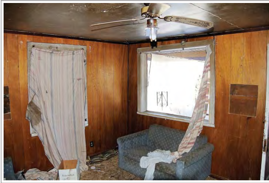
Photo #35: Interior Main Room (2)
