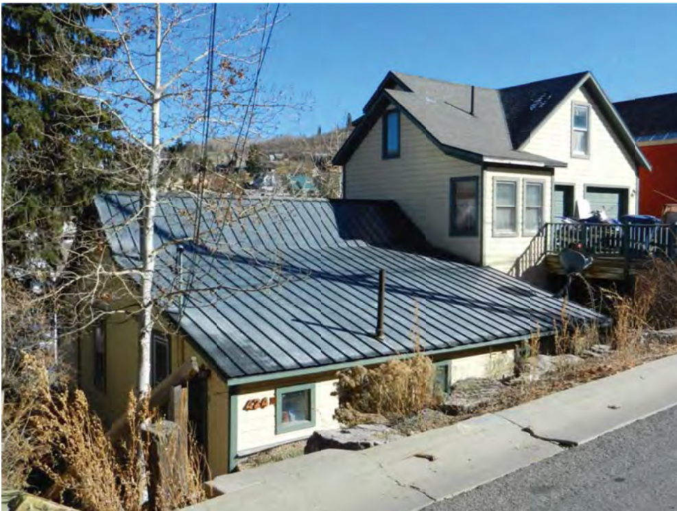
424 Woodside Avenue. Northwest oblique. November 2013.
