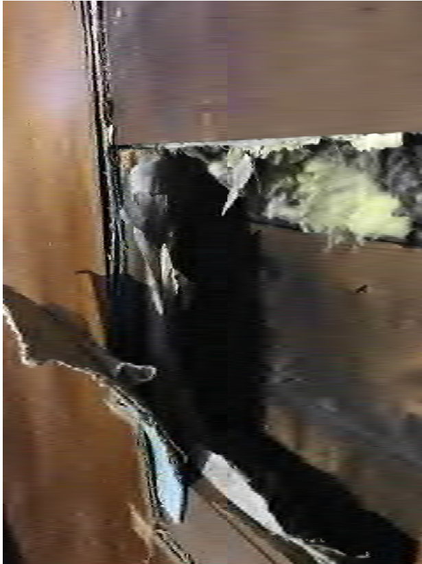
Figure 5 - Existing wall framing with lap board siding
