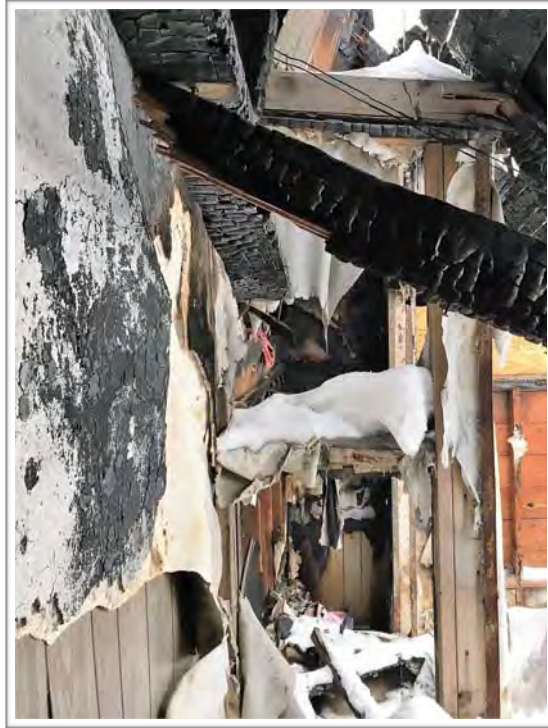
Photo #14: Fire Damage @ Rear Addition
