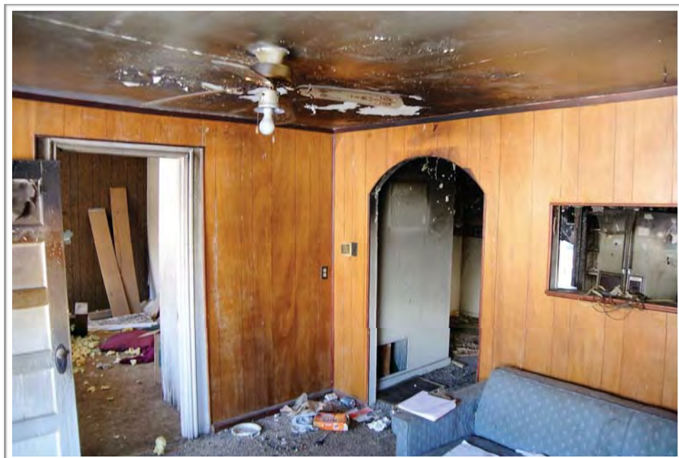
Photo #34: Interior Main Room (1)
