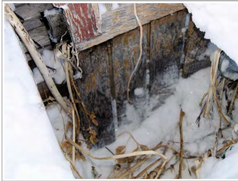
Photo #10: Floor Construction on Grade
