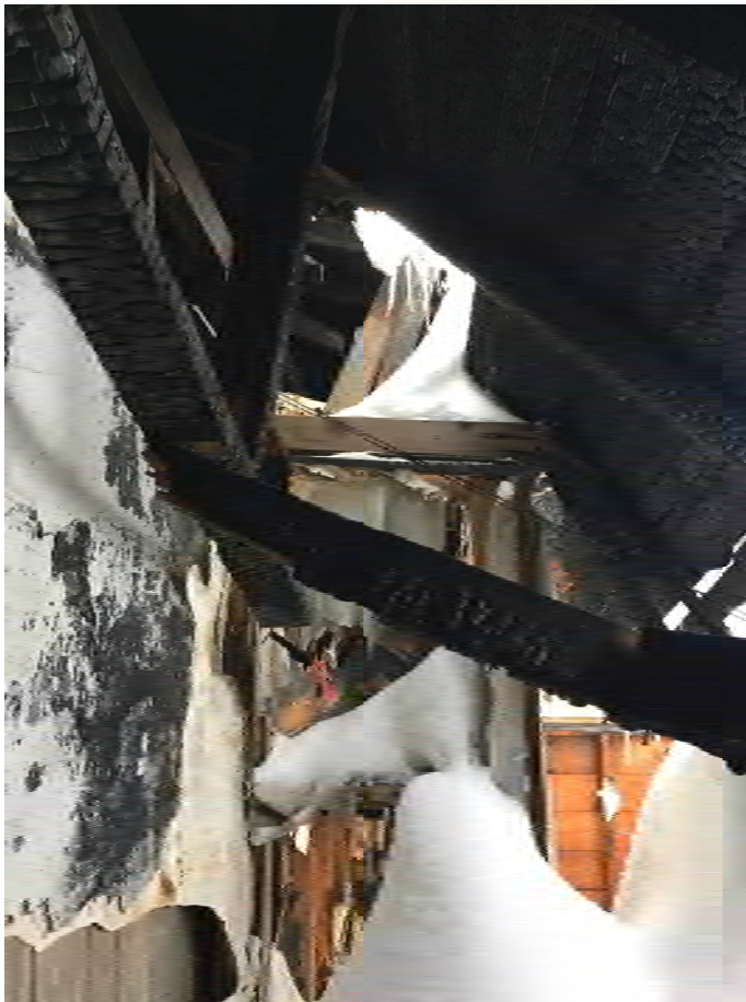
Figure 4 - South Area of roof
