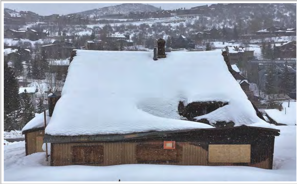
Photo #3: South Elevation
