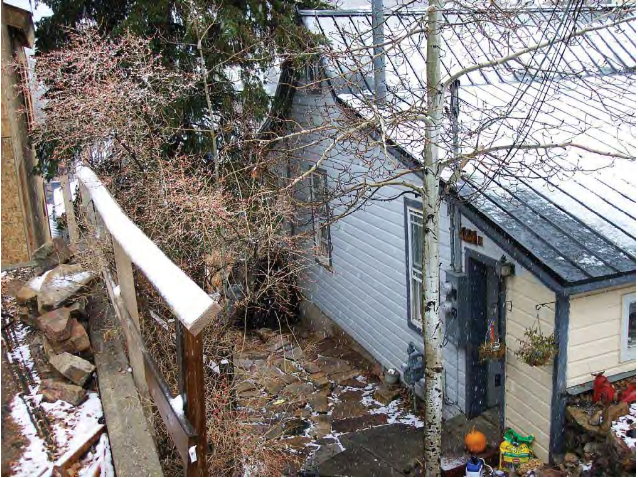
Roof looking southeast
