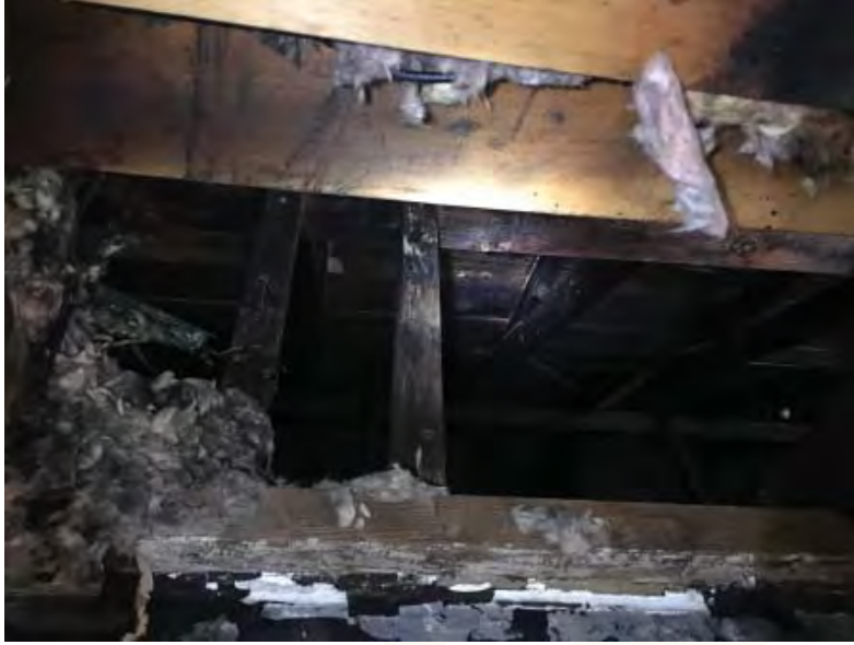
Figure 3 - South Perimeter Wall looking into Attic
