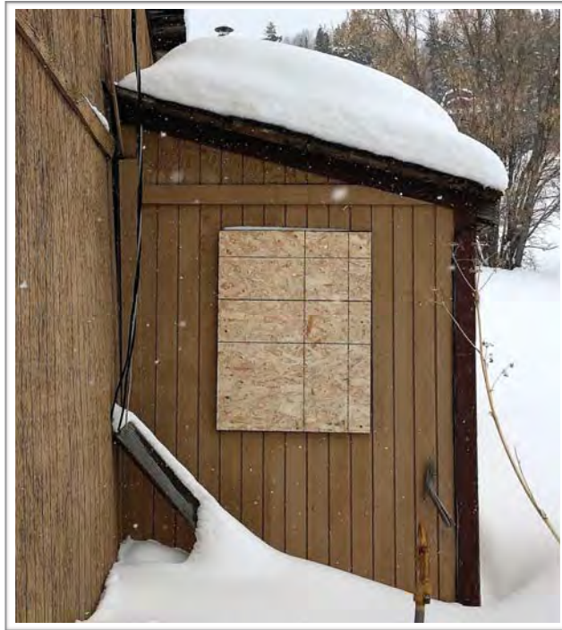
Photo #7: Side Addition (Non-Historic) w/ Historic (?) Roof
