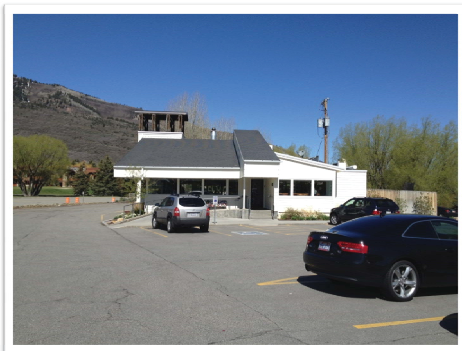
Figure 4 – on site project east elevation
