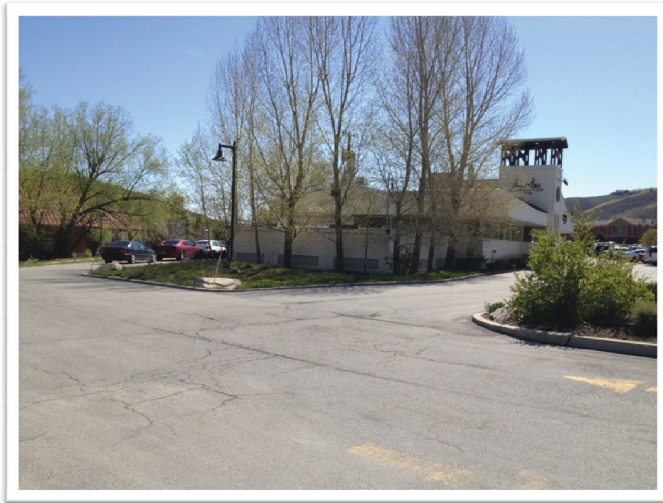
Figure 2a – on site project west elevation
