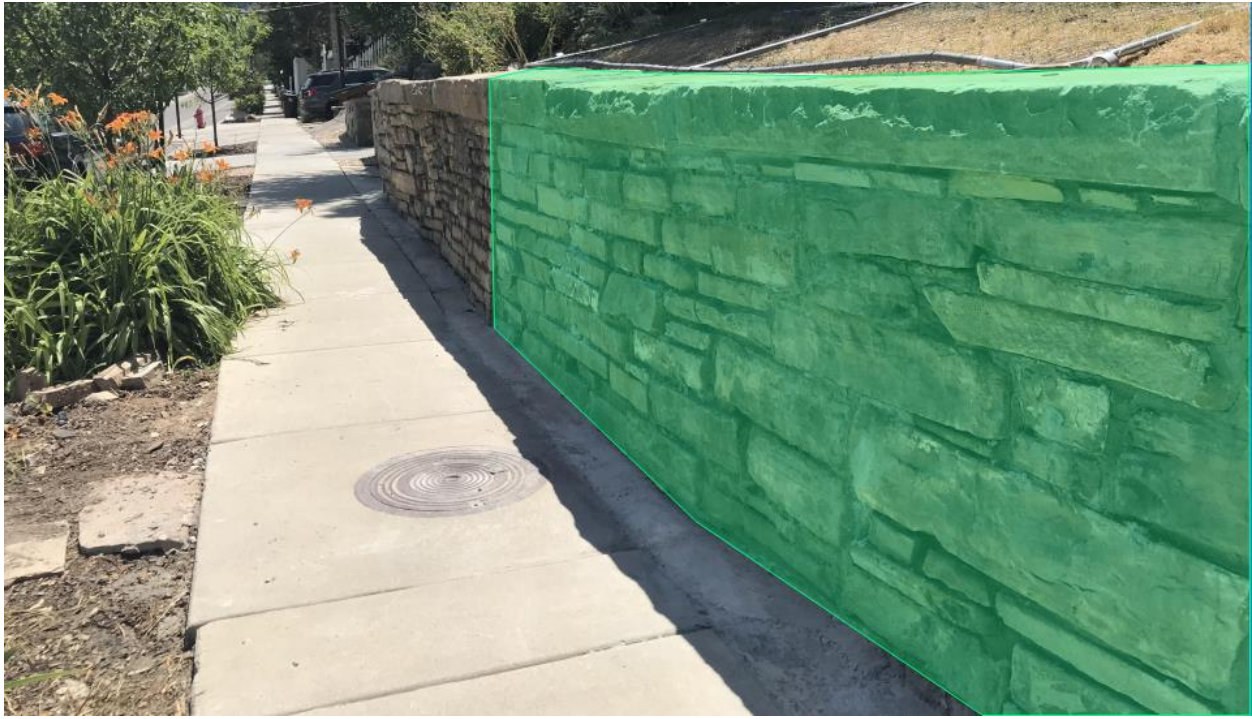
Figure 12: Repaired section of wall to remain.
