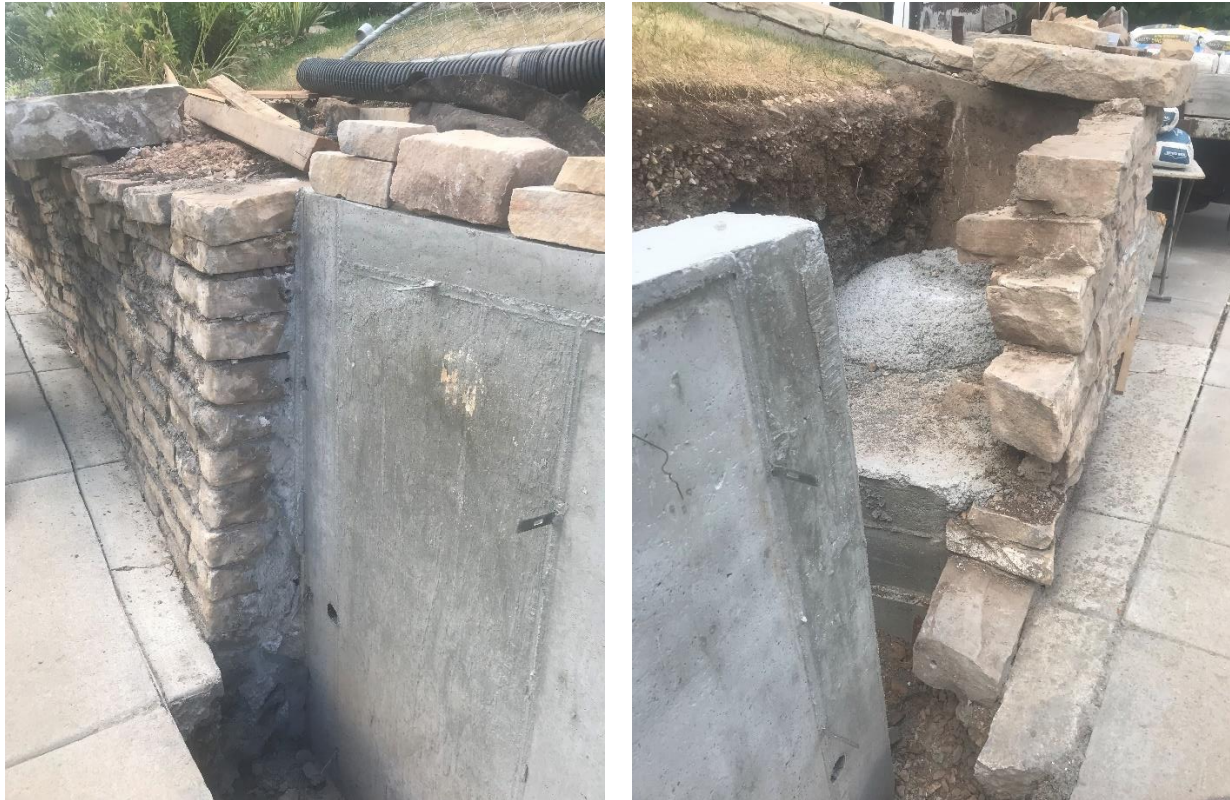
Figure 4: Looking south along wall (left); Looking north along the wall (right).
