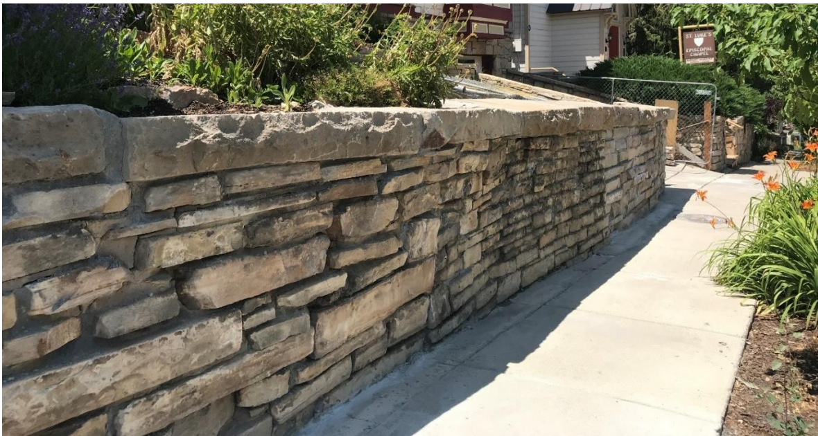
Figure 5: Historic wall in 2018, post repair.
