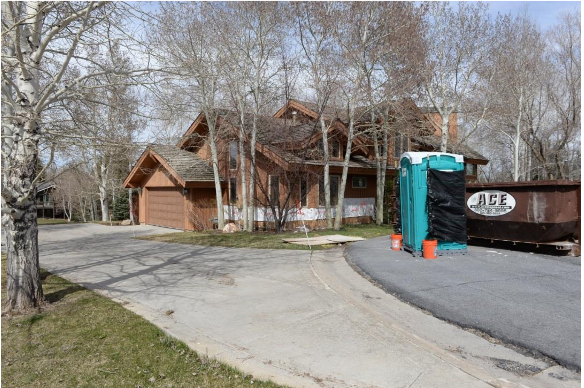
Thaynes Canyon No. 6, Lot 2 – Looking northeasterly
