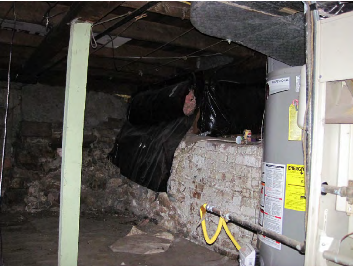
Photo 17: Stacked stone wall
