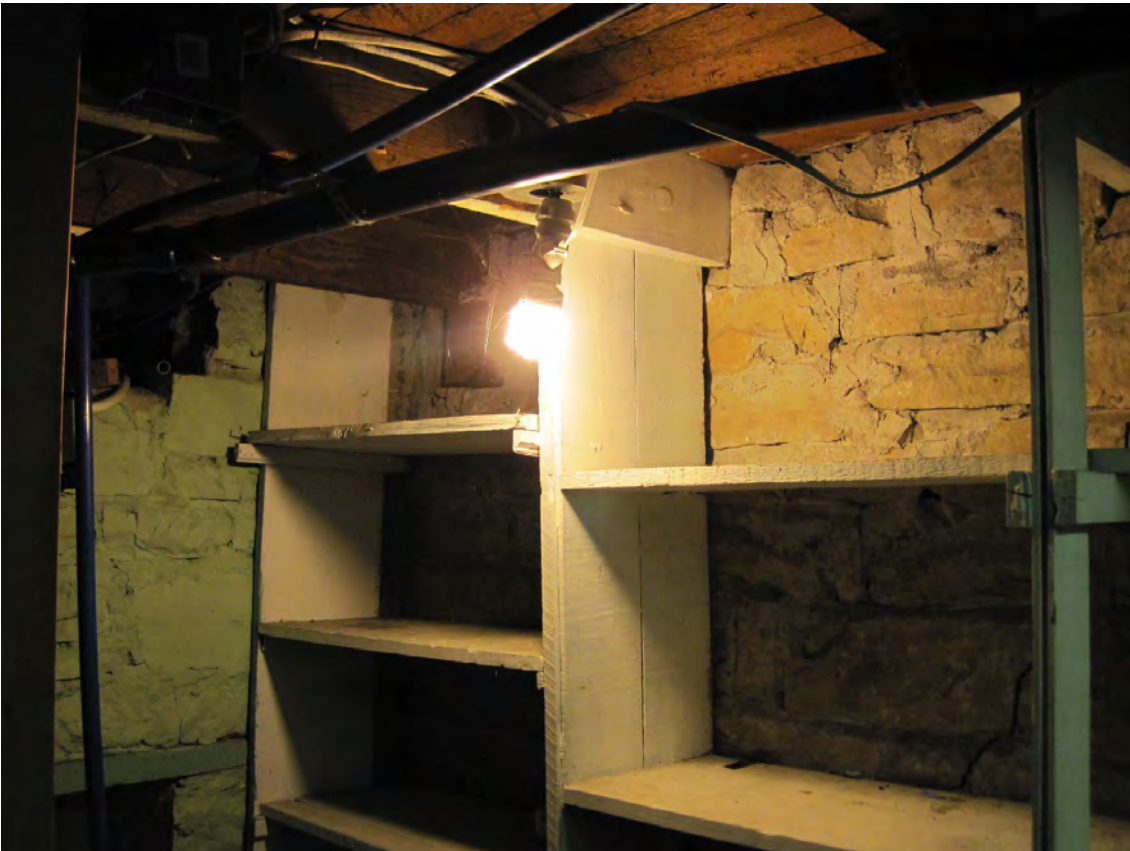
Photo 17: Stacked stone wall
