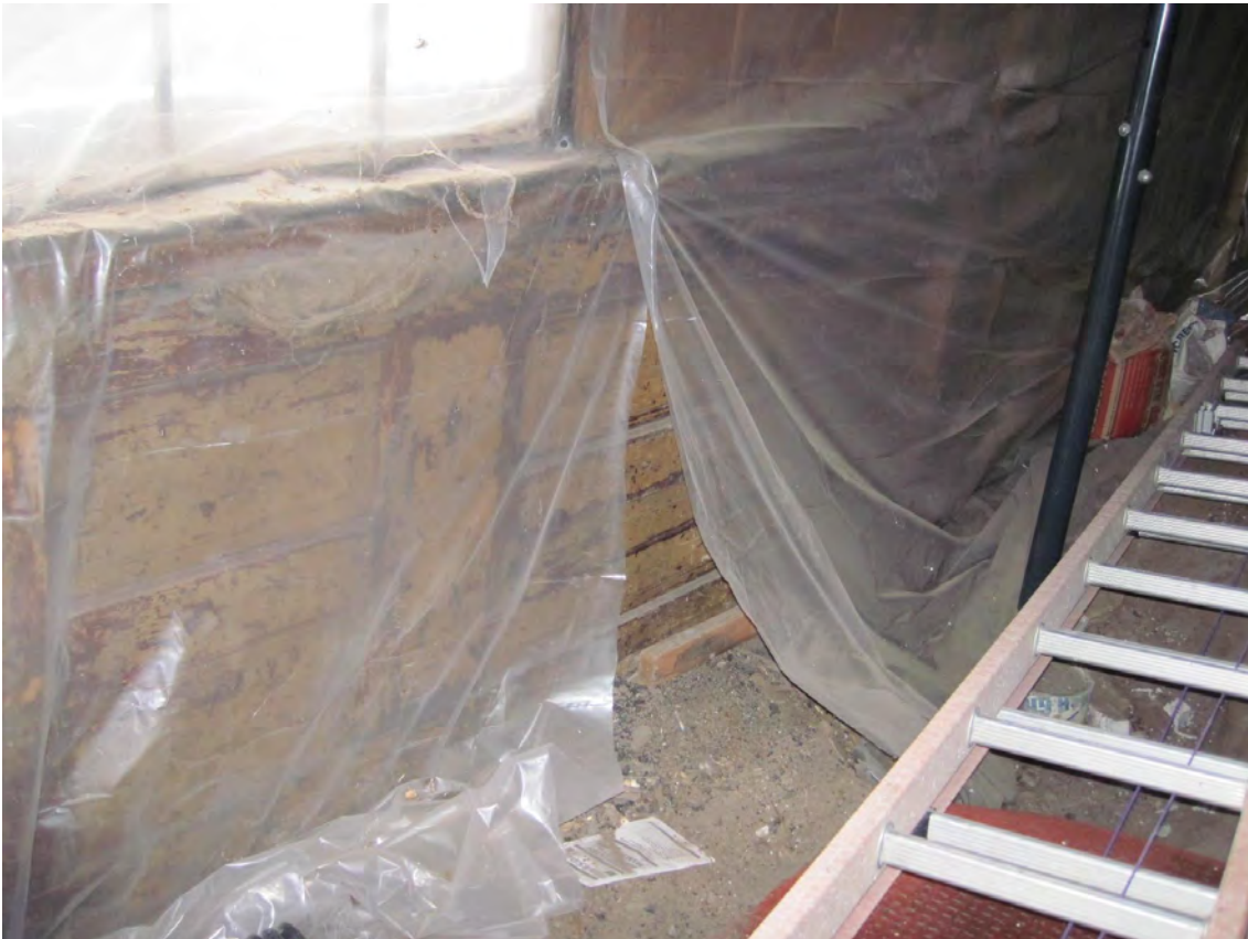
Photo 19: East bearing wall sits on soil
