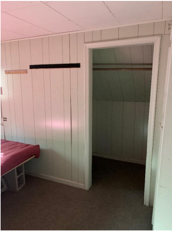
Photo 37: Upper level bedroom closet
