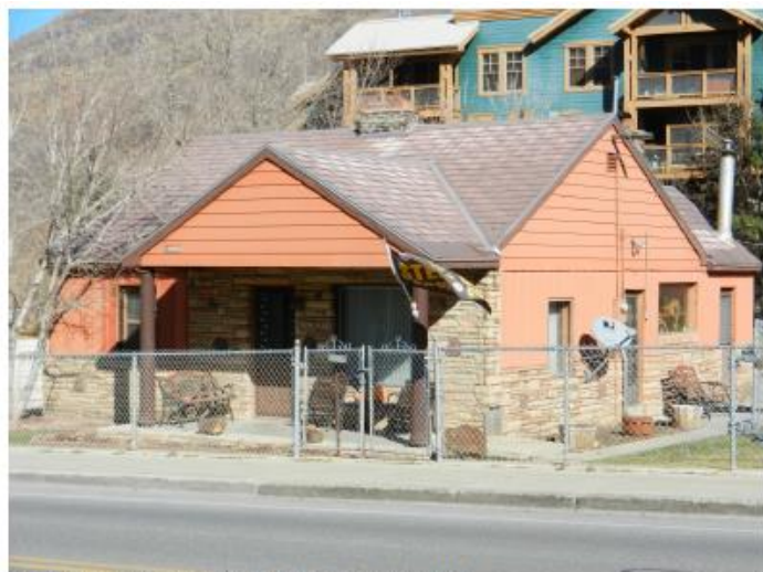
1060 Park Avenue. Southwest oblique. November 2013.
