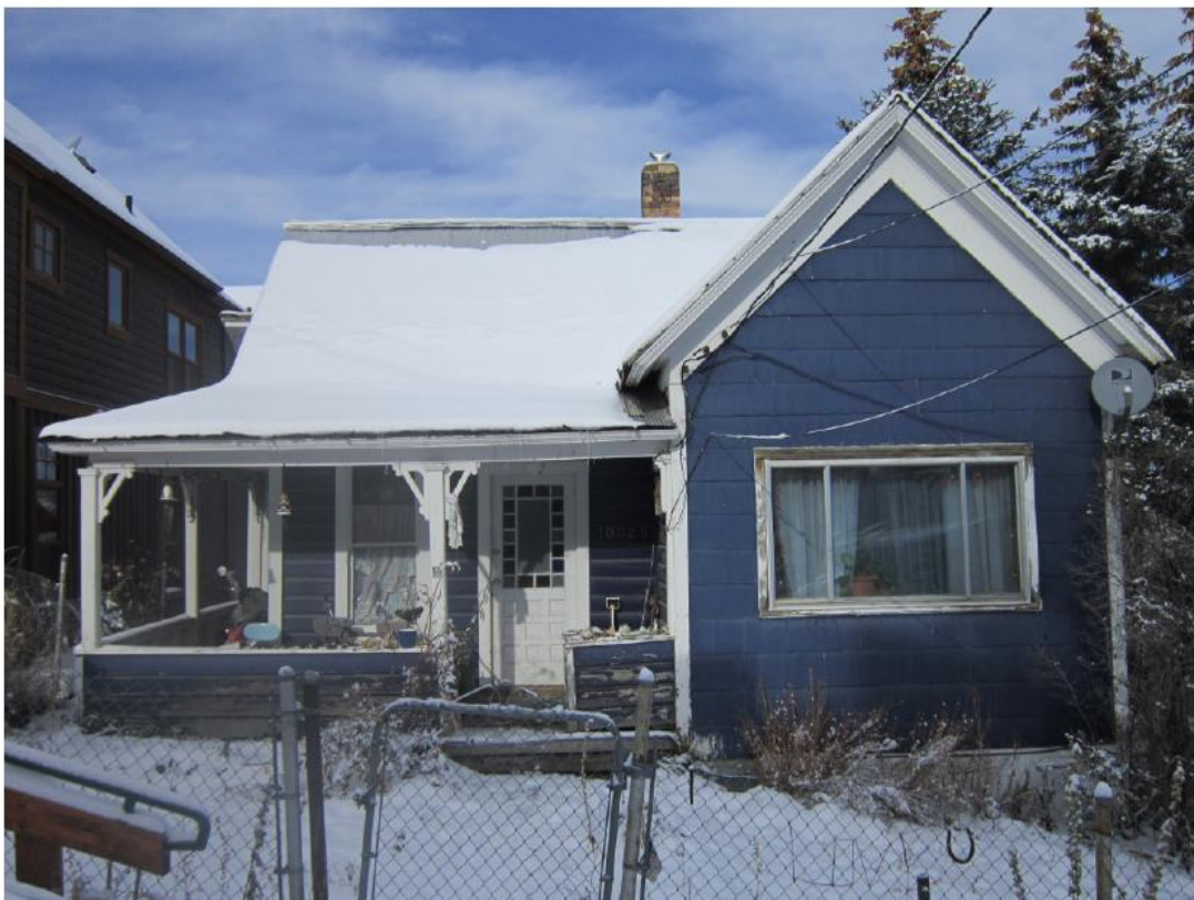
1002 ½ Norfolk Avenue. South elevation. November 2013.
