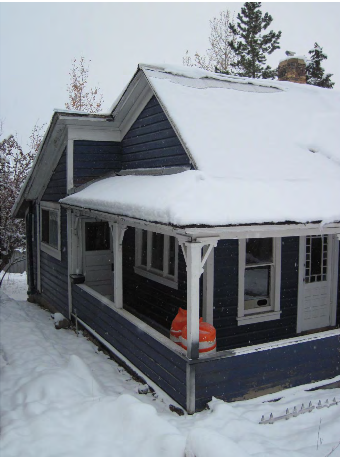
Photo 12: South / West elevation
