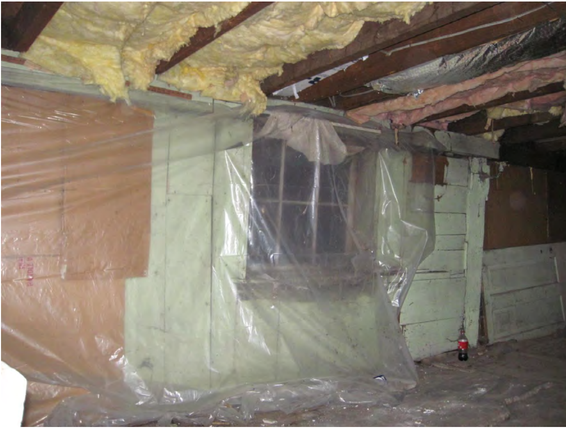
Photo 19: East bearing wall sits on soil
