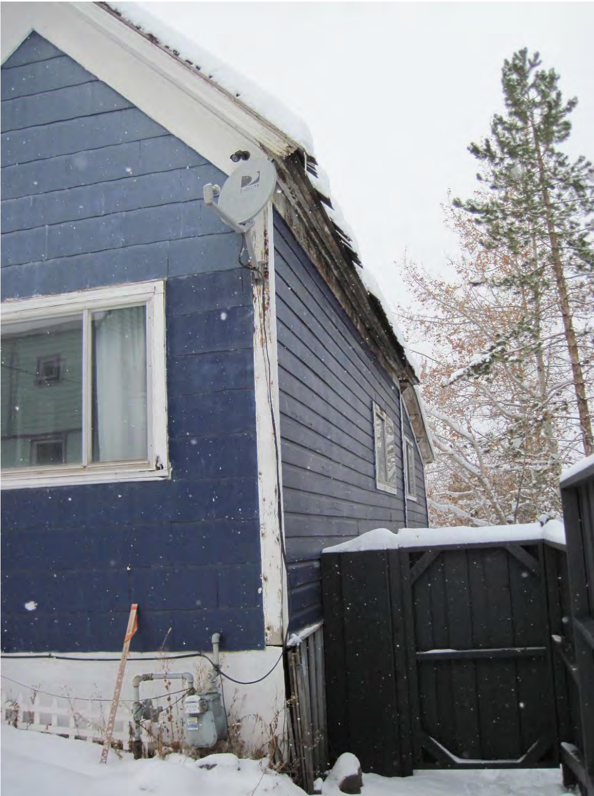
Photo 13: South / East elevation
