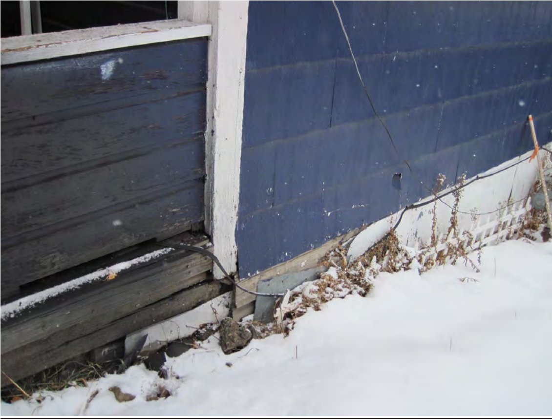
Photo 24: Porch at west elevation, sits on stacked stone and soil
