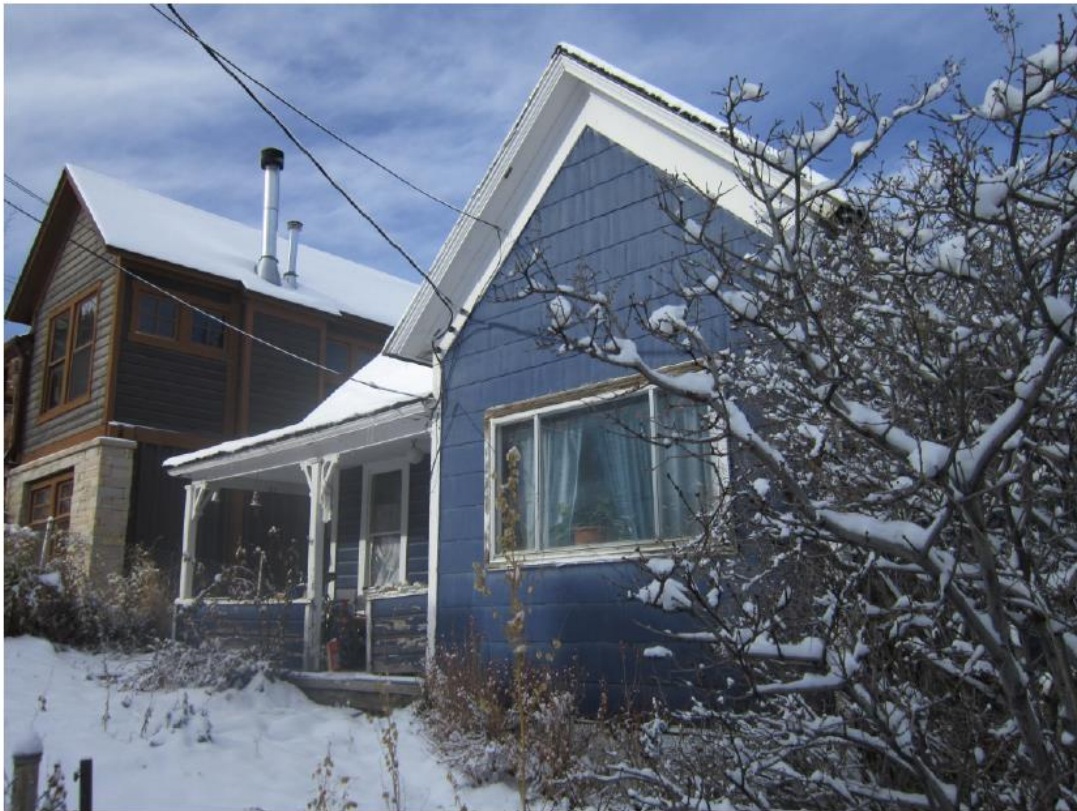
1002 ½ Norfolk Avenue. Southeast oblique. November 2013.
