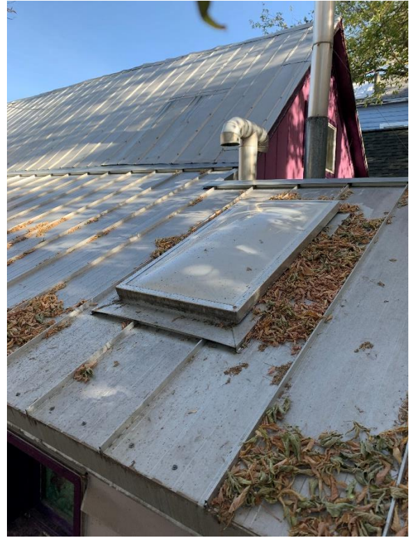
Photo 59: North elevation sky light
