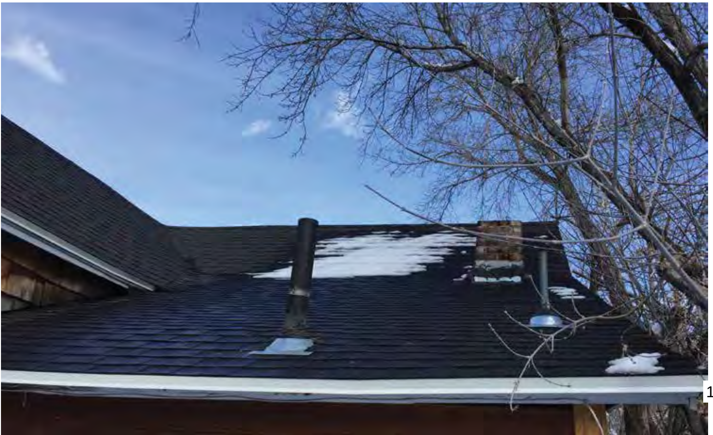
Photo #14: Roof From Rear Yard
