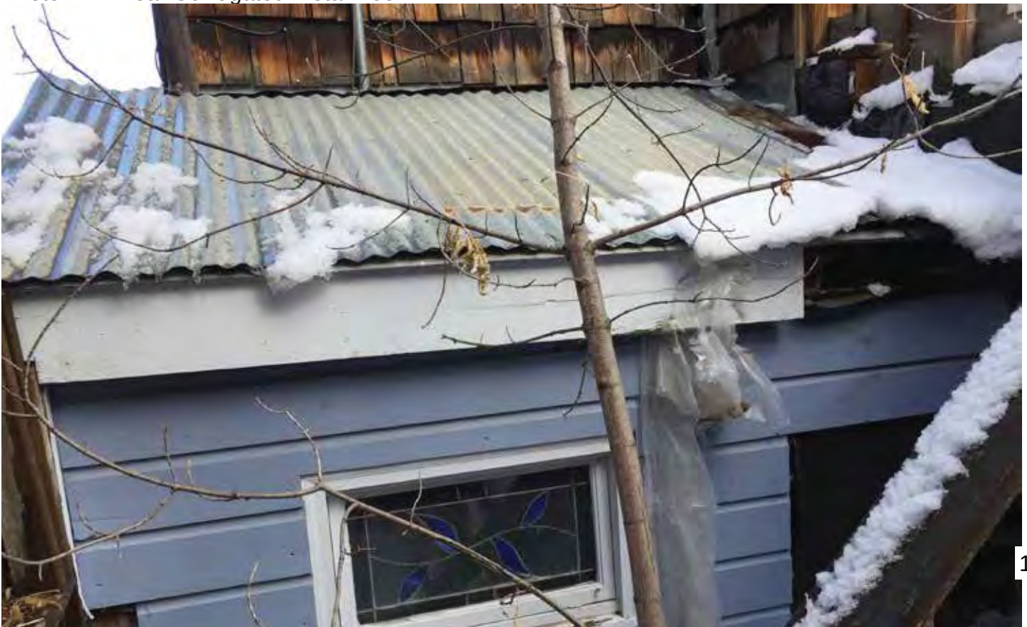
Photo #17: Rear Corrugated Metal Roof
