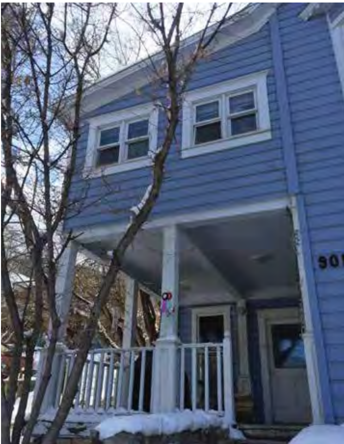
Photo #24: Front Facade Detail
