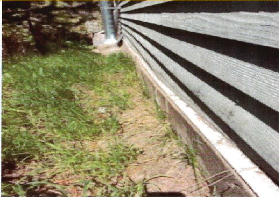
Photo 3: Exterior Concrete Frost Wall
