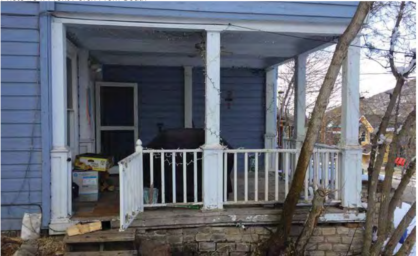
Photo #34: Front Porch From South
