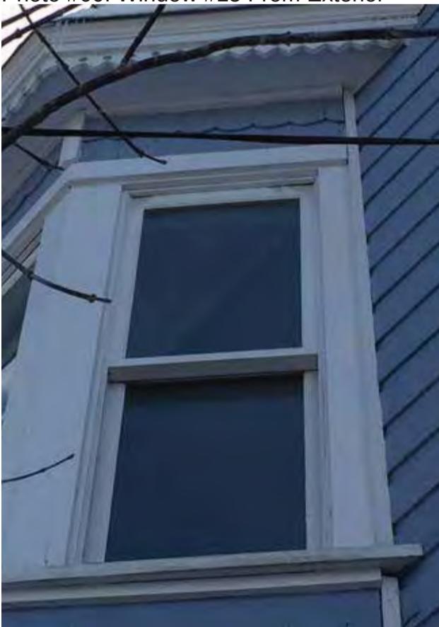
Photo #60: Window #15 From Exterior
