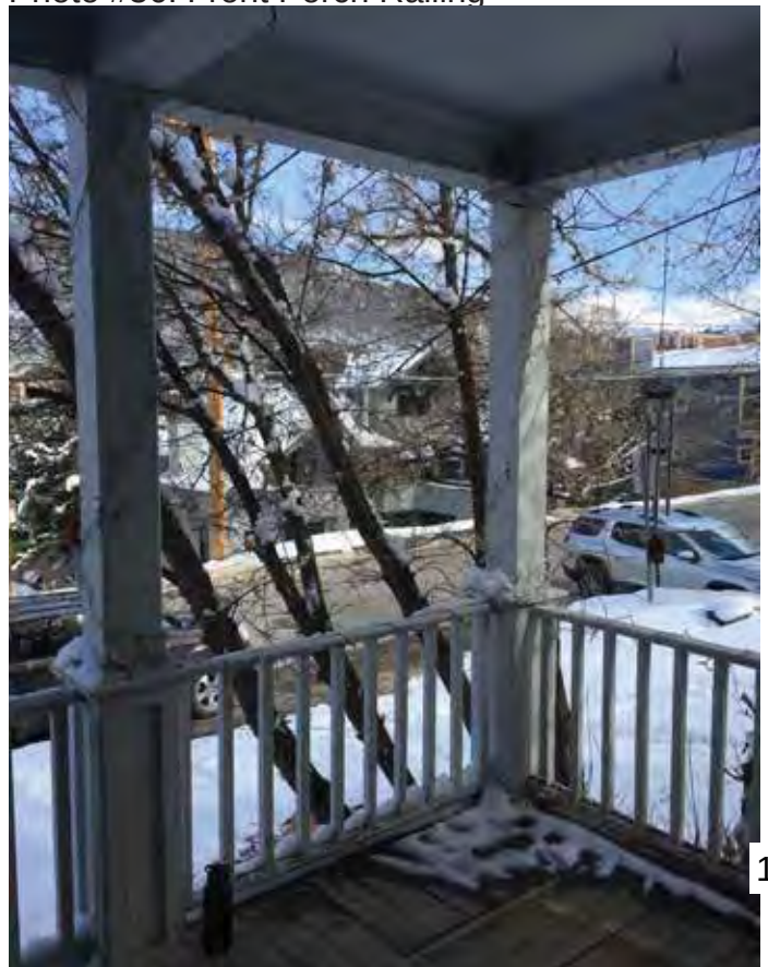
Photo #36: Front Porch Railing
