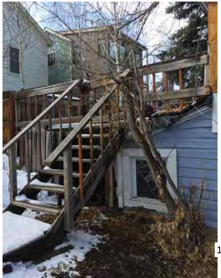
Photo #6: Stair From Side Yard
