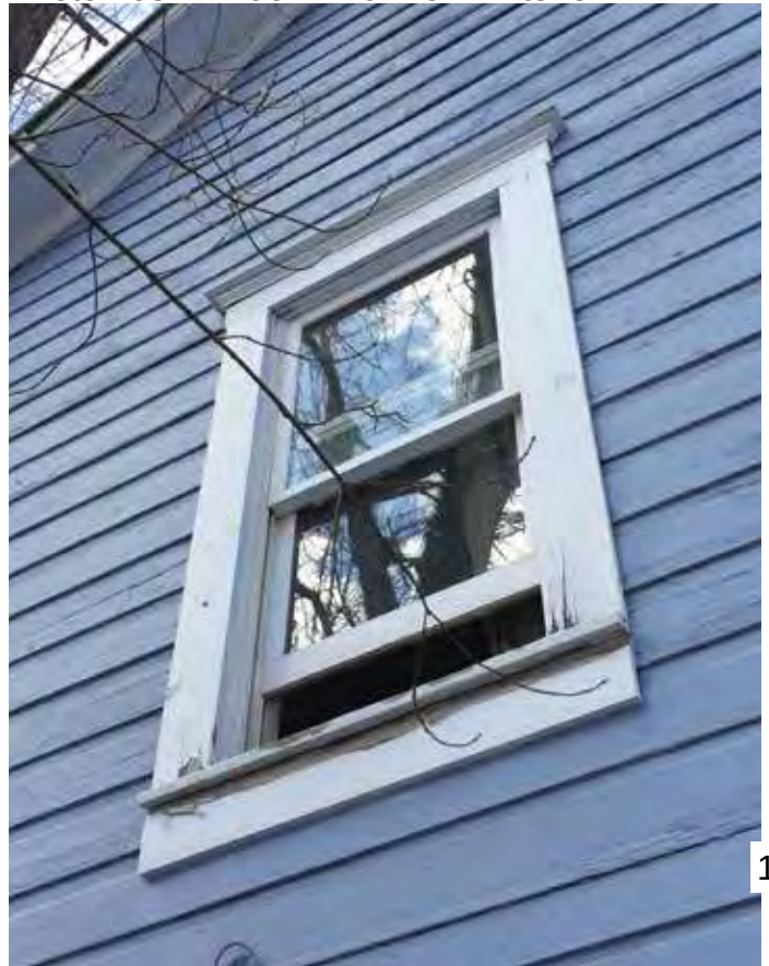
Photo #65: Window #20 From Exterior
