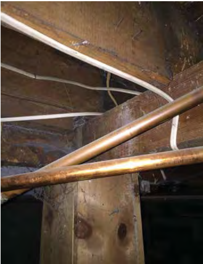
Photo #10: Posts & Beam Main Level
