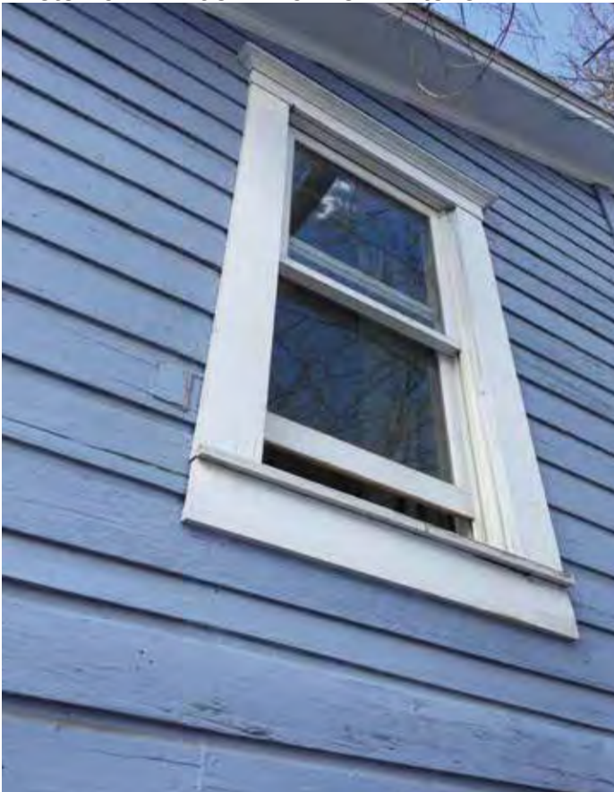
Photo #64: Window #19 From Exterior
