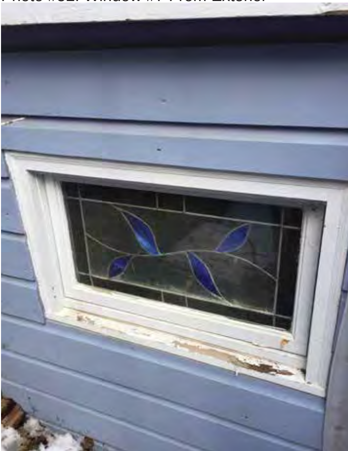
Photo #52: Window #7 From Exterior
