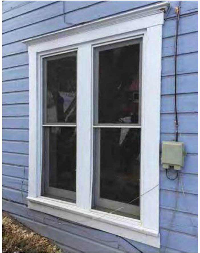
Photo #55: Window #10 From Exterior
