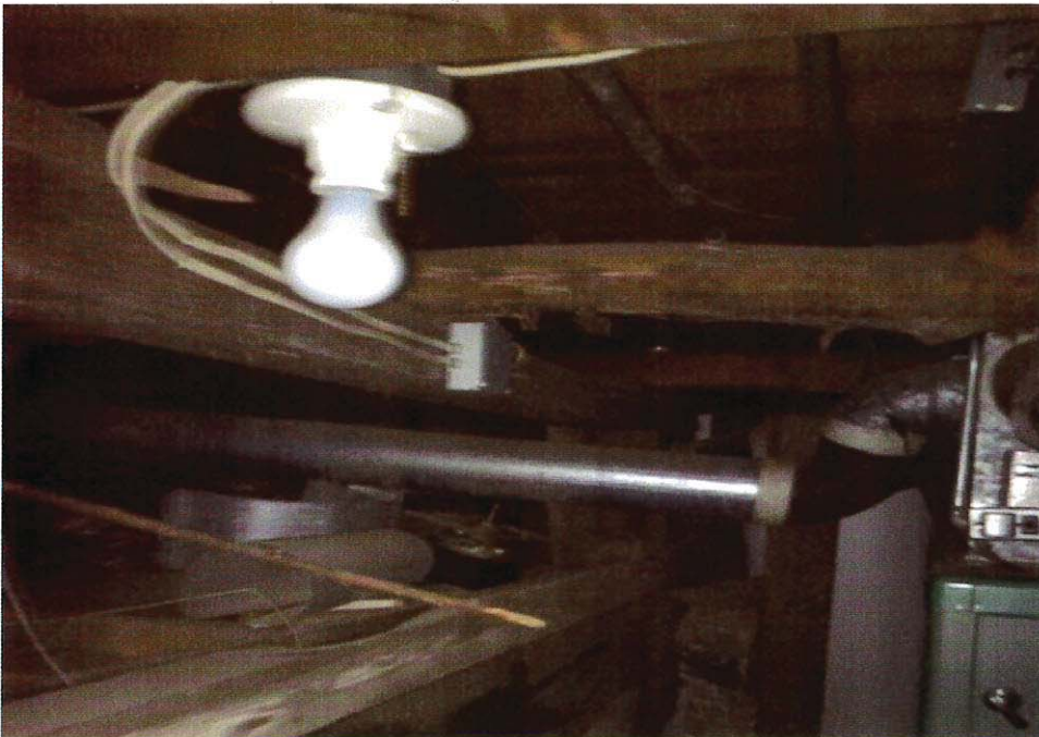
Photo 6: Sub-Floor Beams and Joists
