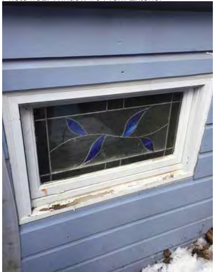
Photo #51: Window #6 From Exterior
