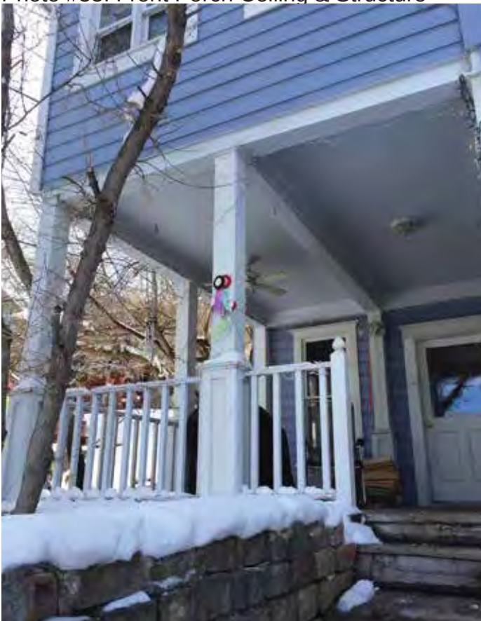
Photo #35: Front Porch Ceiling & Structure
