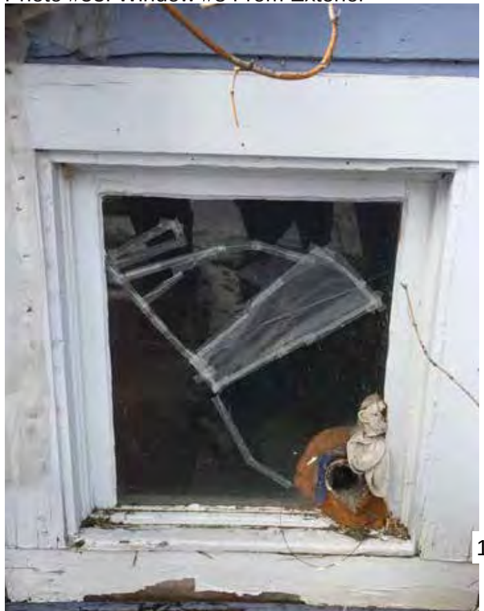
Photo #53: Window #8 From Exterior
