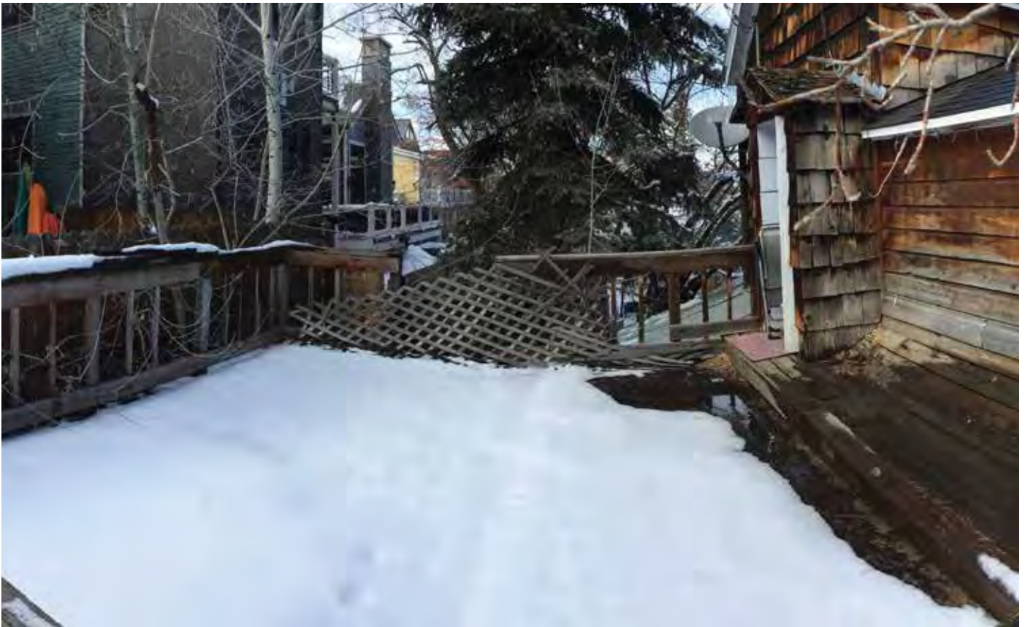
Photo #4: Rear Deck
