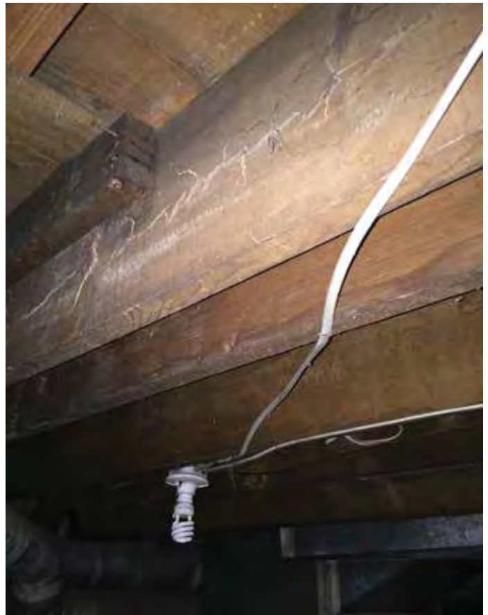
Photo #11: 2x10 Joists Under Main Level
