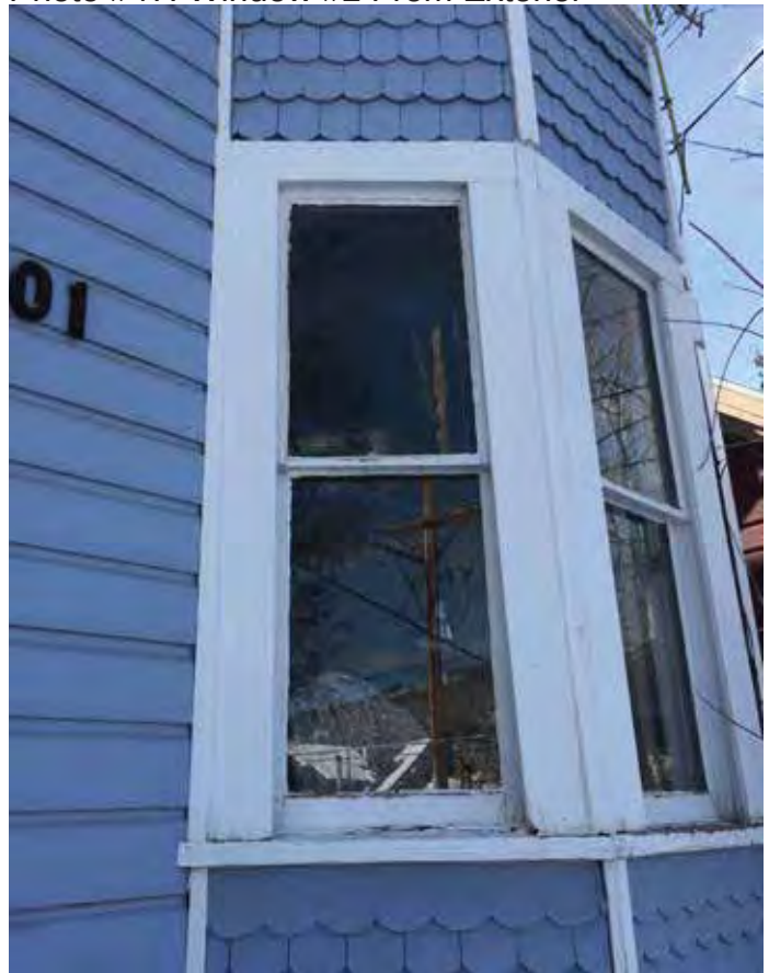
Photo #47: Window #2 From Exterior
