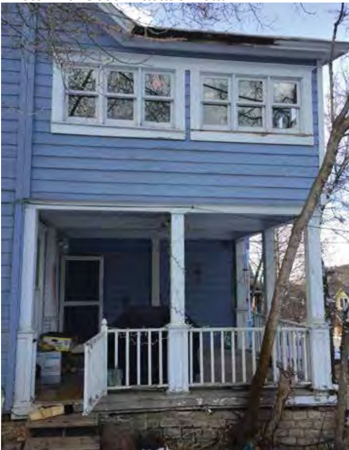
Photo #26: South Facade Detail
