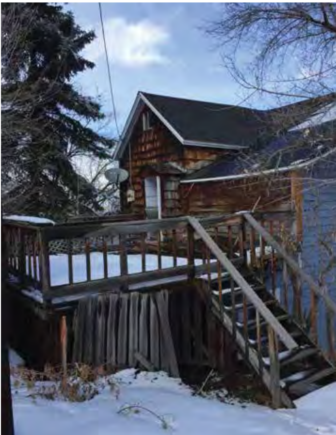
Photo #5: Rear Deck
