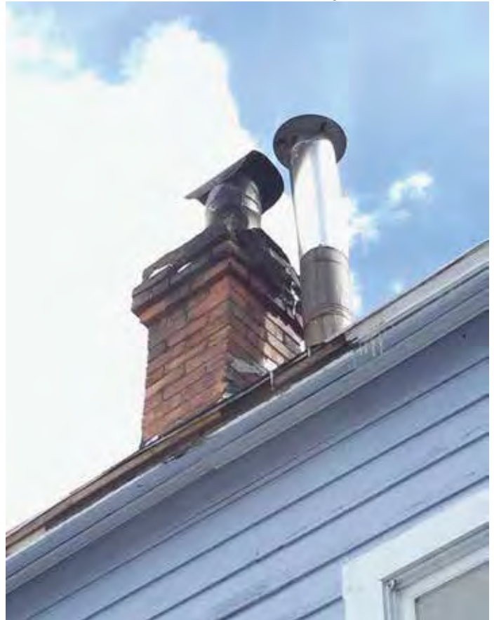
Photo #19: Zoom Out w/ Chimney Location
