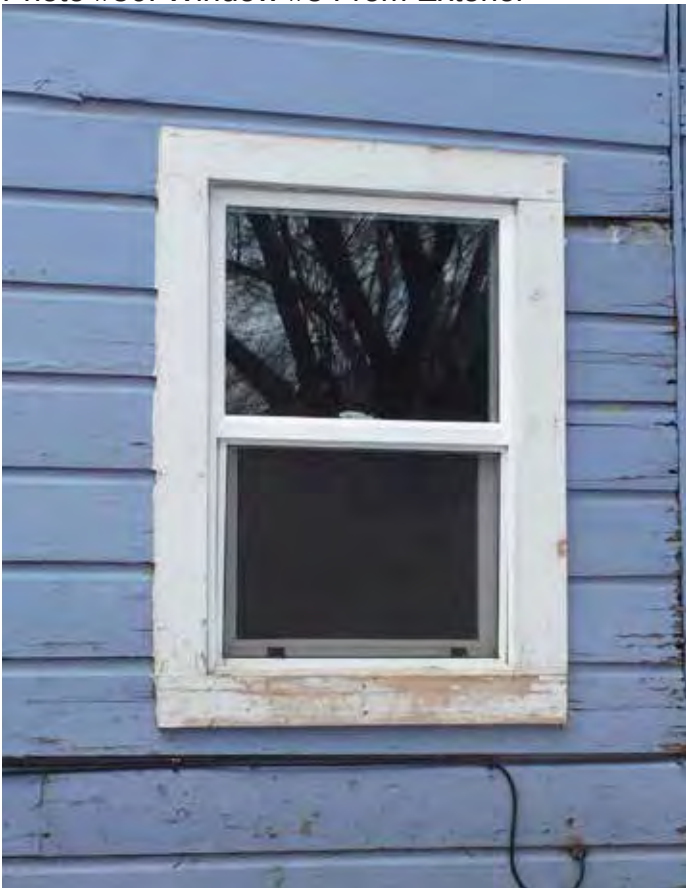
Photo #50: Window #5 From Exterior
