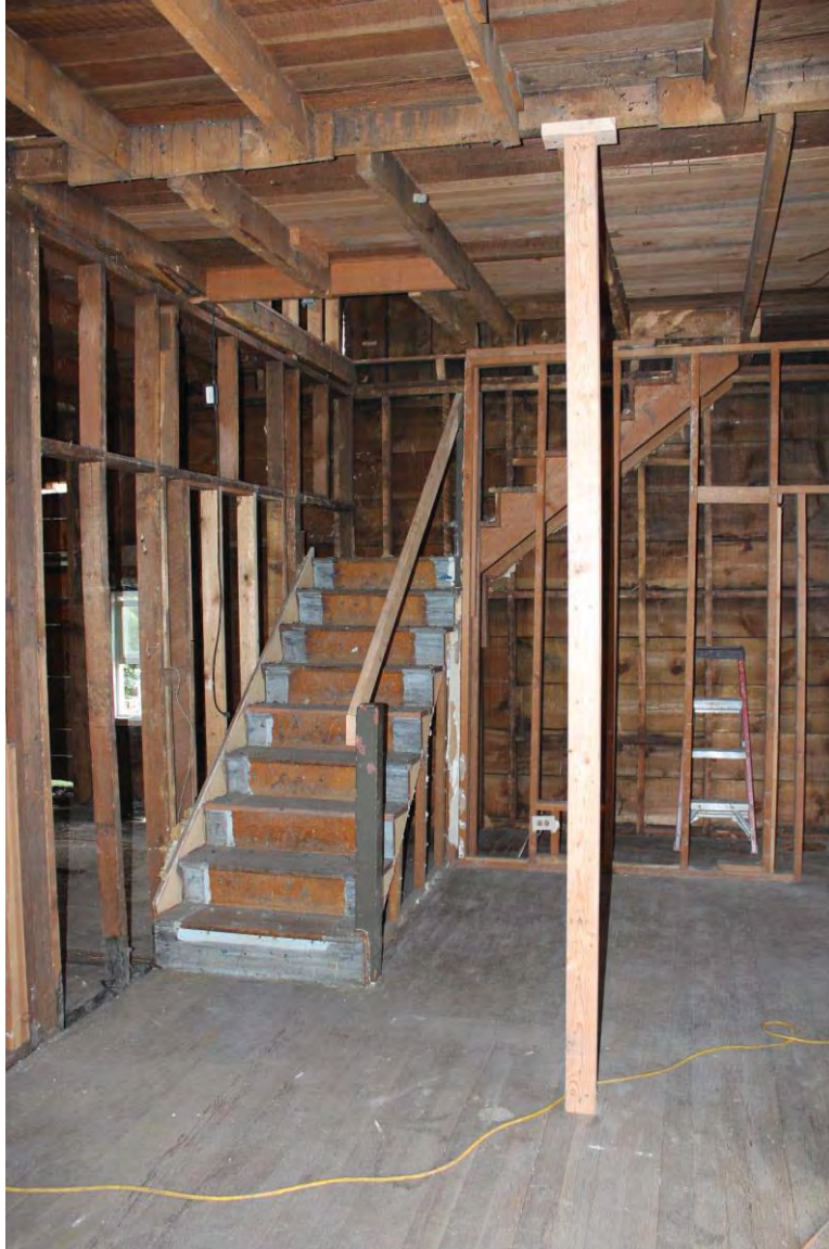
Figure 4. General view of interior, including non-historic staircase, facing northwest. Note the stud wall framing on this level.
