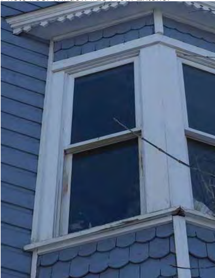
Photo #58: Window #13 From Exterior
