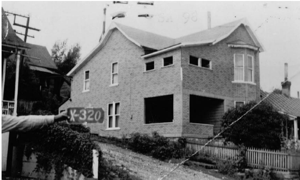
Figure 2 – Photo of 901 Woodside from the circ. 1941 tax assessment
