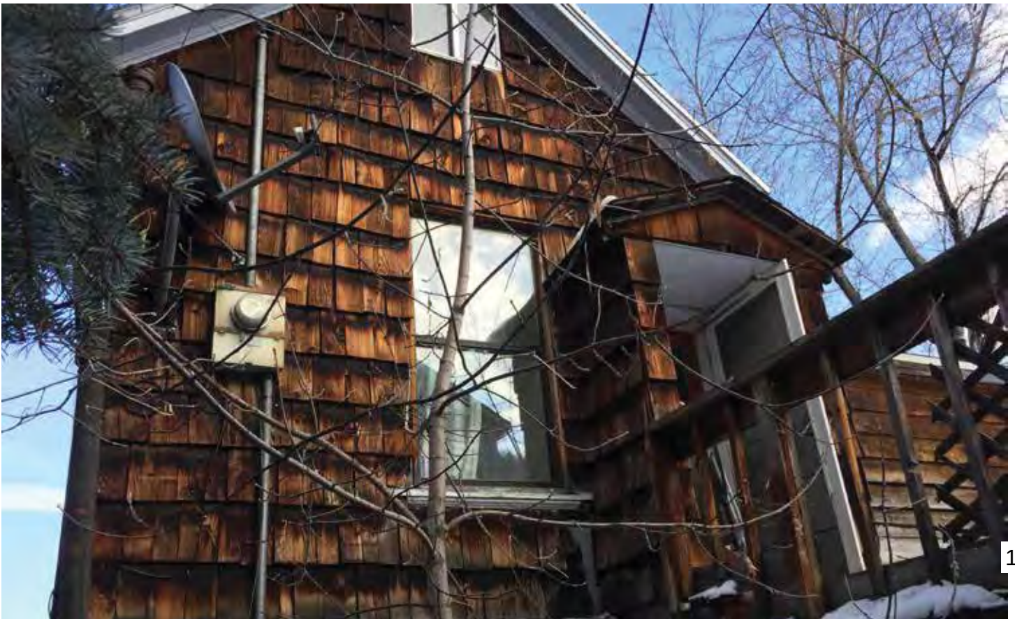
Photo #28: Left Portion of Rear Facade
