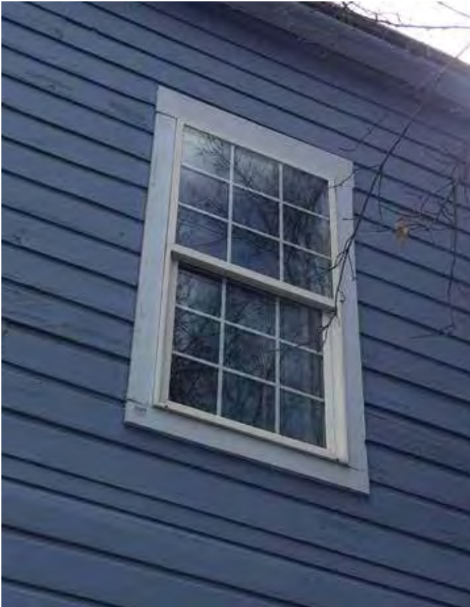
Photo #62: Window #17 From Exterior
