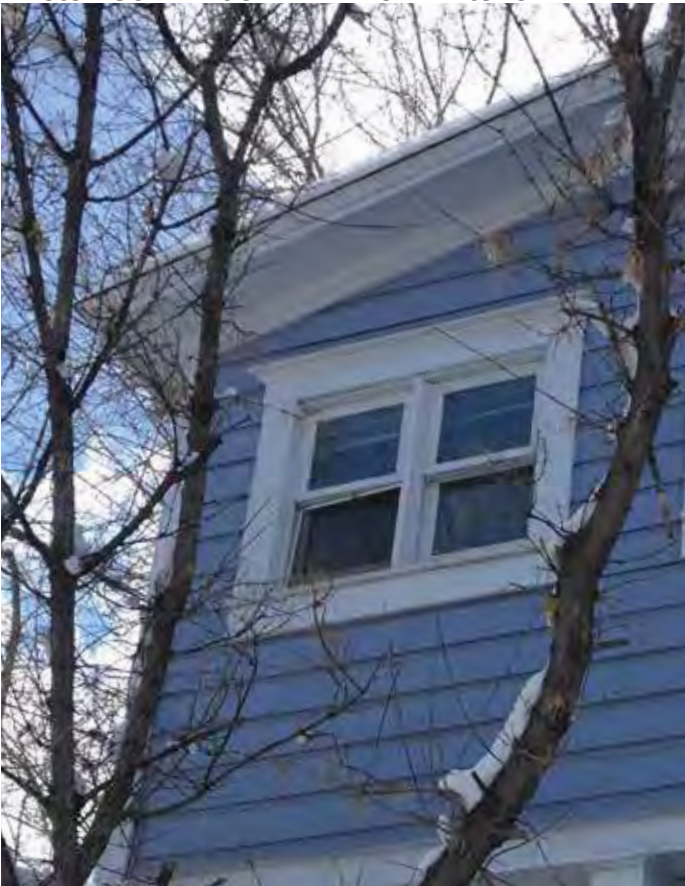
Photo #56: Window #11 From Exterior
