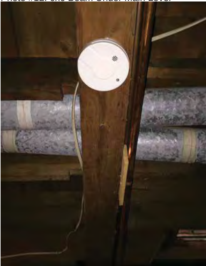
Photo #12: 6x6 Beam Under Main Level
