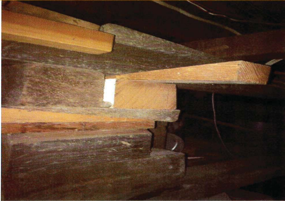
Photo 5: Sub-Floor Shimming
