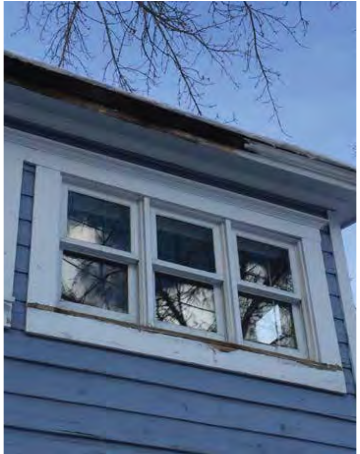
Photo #67: Window #22 From Exterior
