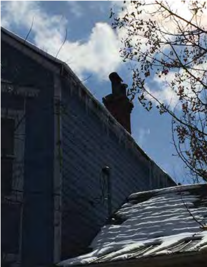
Photo #18: Brick Chimney w/ Metal Exhaust
