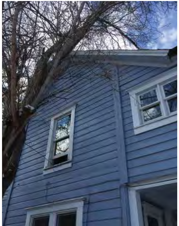
Photo #16: B.O. Soffit
