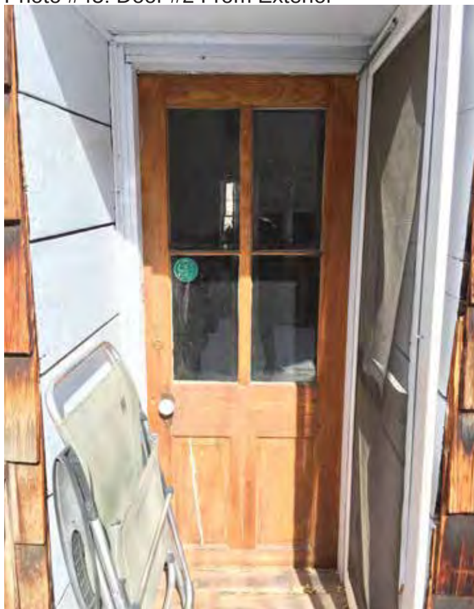
Photo #45: Door #2 From Exterior
