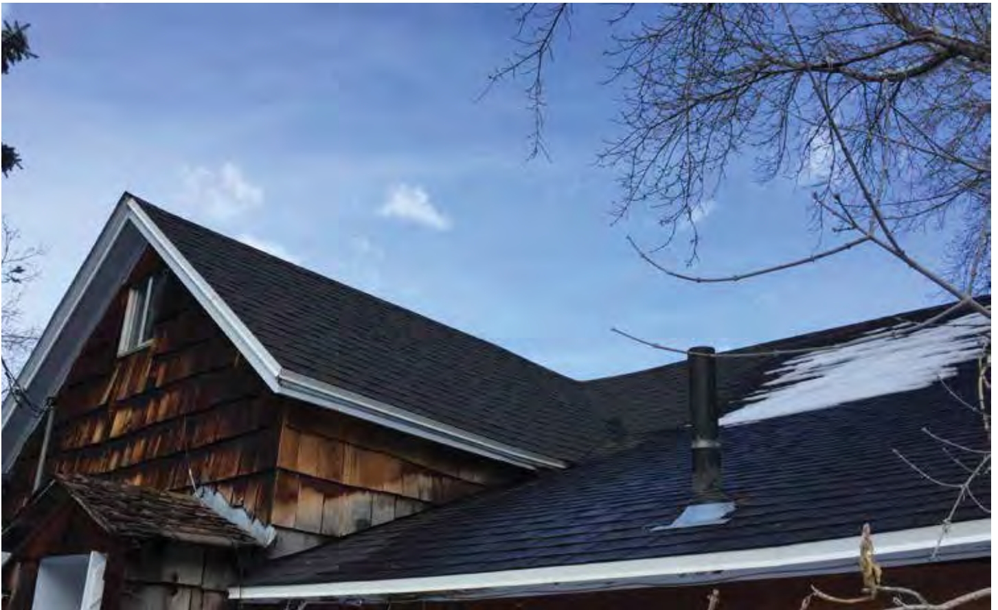
Photo #13: Southwest Corner of Roof
