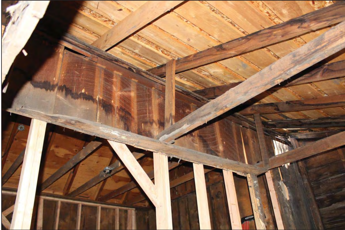
Figure 6. Detail of vertical plank construction at the top of an interior second-story wall, facing east. The lighter marks at the edges of the planks mark the former location of battens and indicate that this was once an exterior wall, most likely of the original one-story house. The remnants of a wood shingle roof are also visible at the top of this wall, an indication that the one-story house was not dismantled but rather raised in one piece in the 1890s, prior to the construction of the two-story, shed-roofed rear addition.
