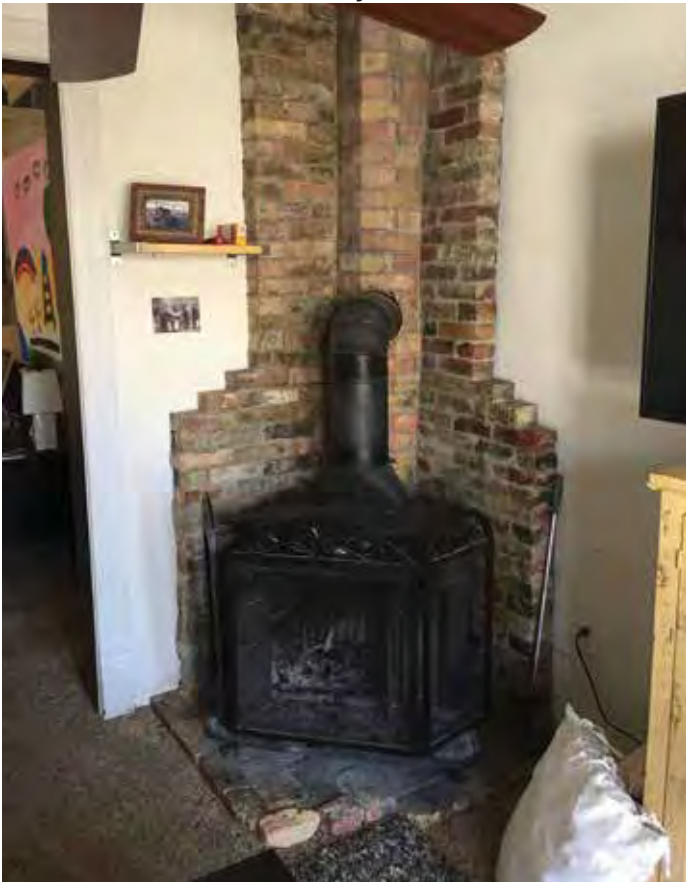
Photo #20: Brick Chimney On Main Level
