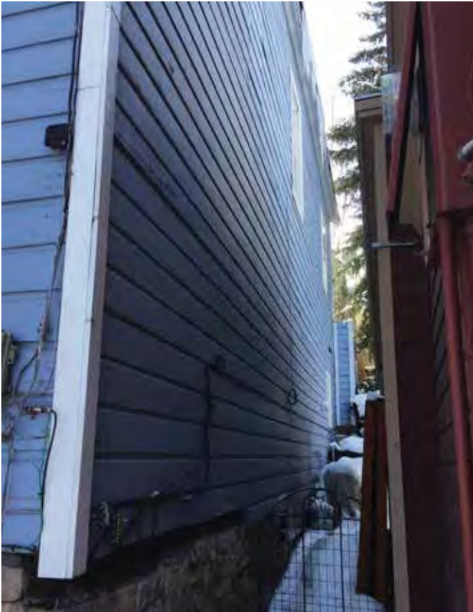
Photo #29: North Facade
