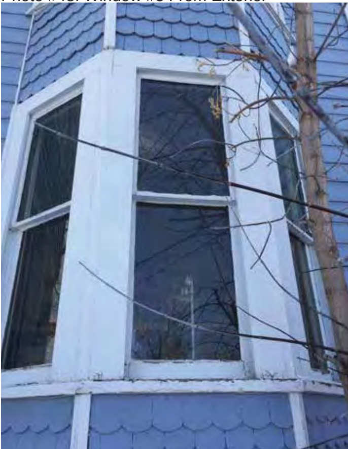
Photo #48: Window #3 From Exterior
