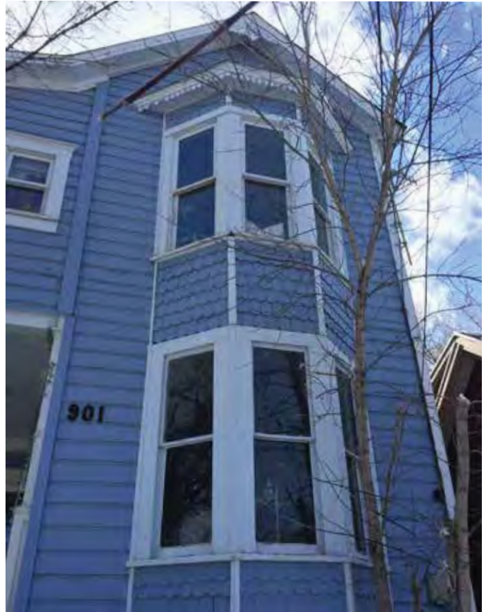
Photo #23: Front Facade Detail
