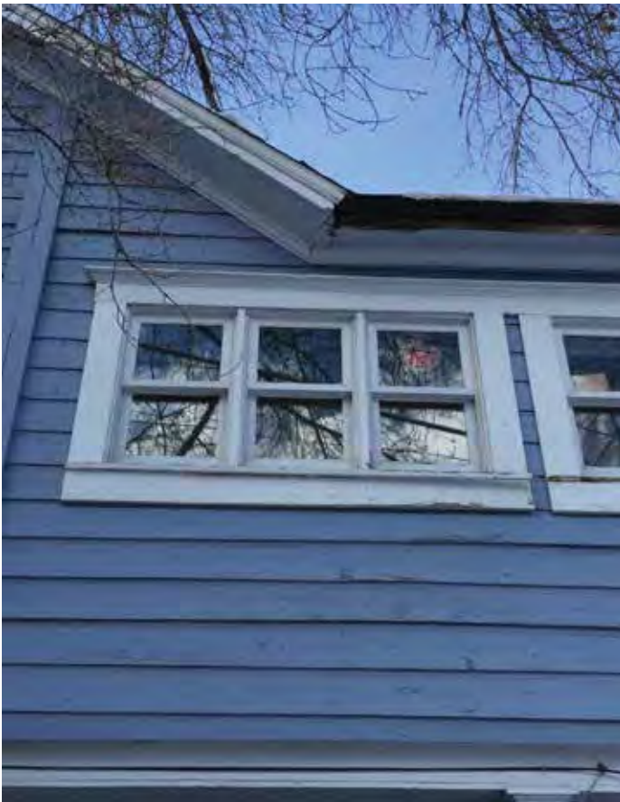
Photo #15: Roof Intersection
