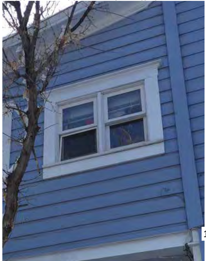
Photo #57: Window #12 From Exterior
