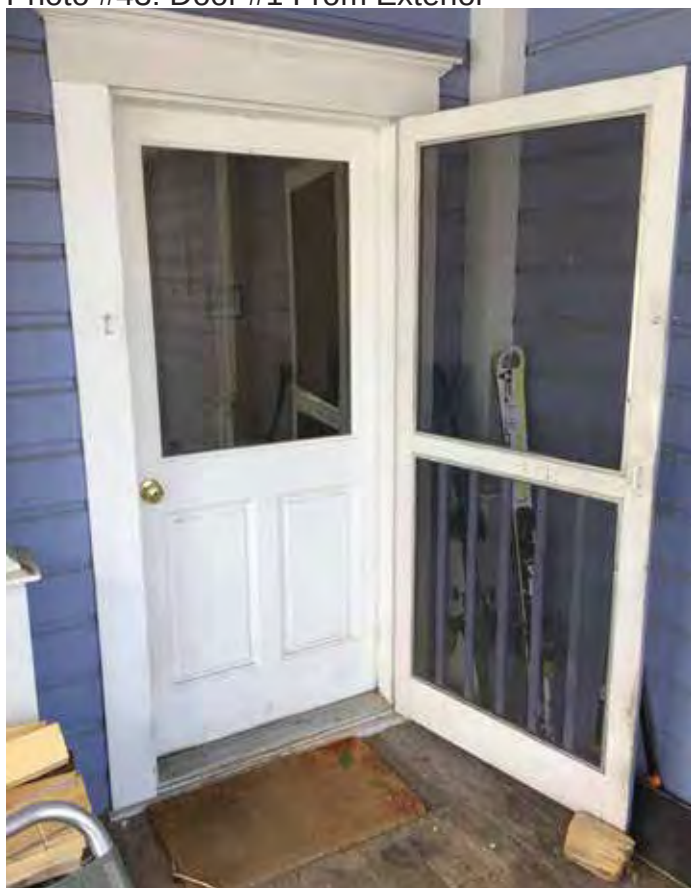
Photo #43: Door #1 From Exterior
