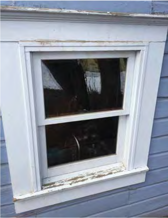
Photo #54: Window #9 From Exterior
