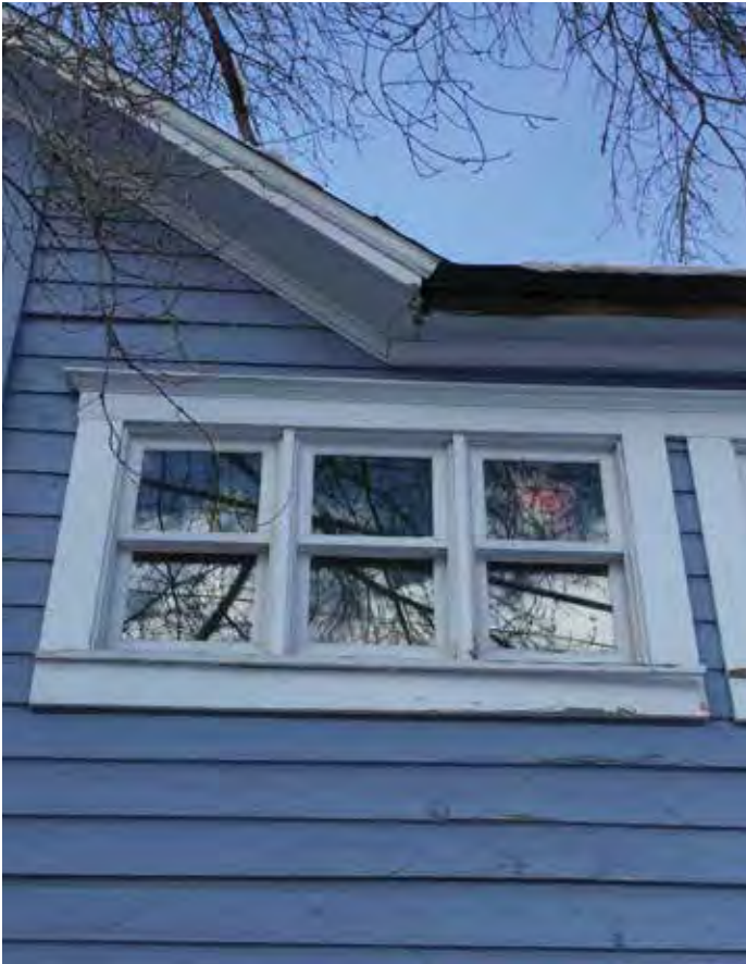
Photo #66: Window #21 From Exterior
