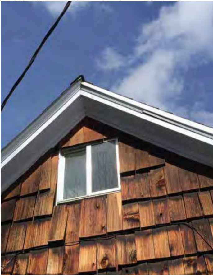
Photo #68: Window #23 From Exterior
