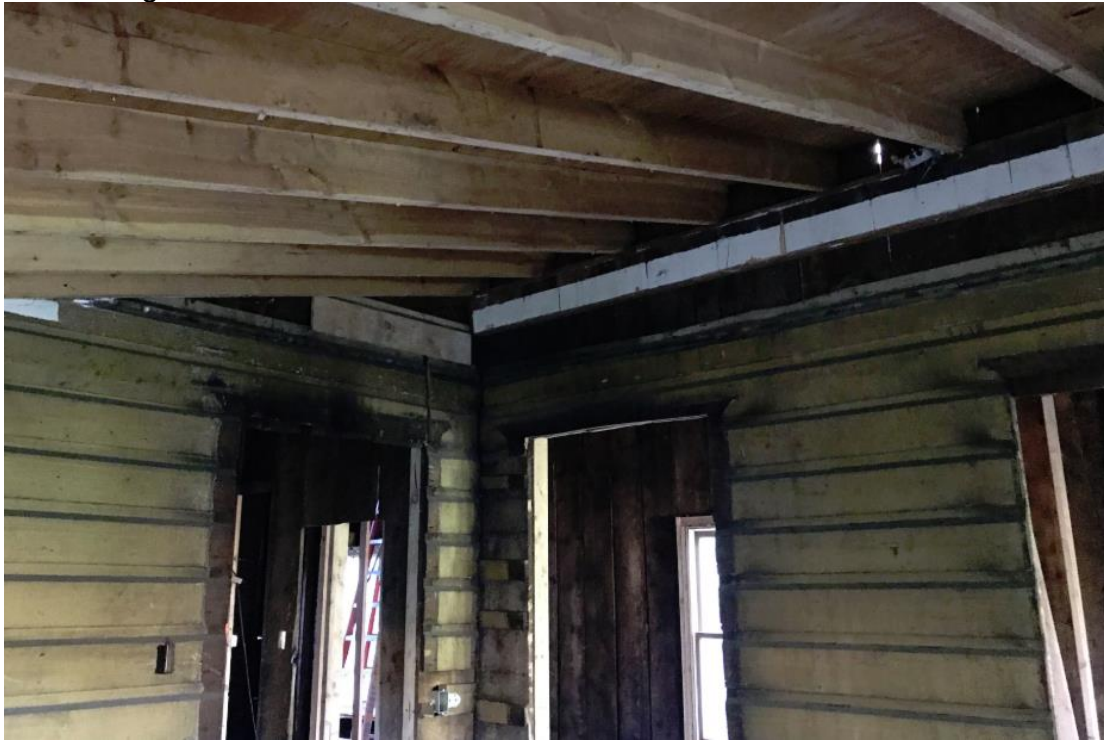
Figure 9 Photo showing the original L shaped front porch and original drop siding and evidence of original roof structure.
