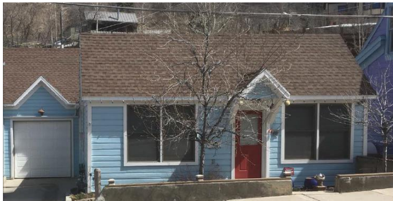
Figure 4: Photo of 158 Main Street dated 2018.
