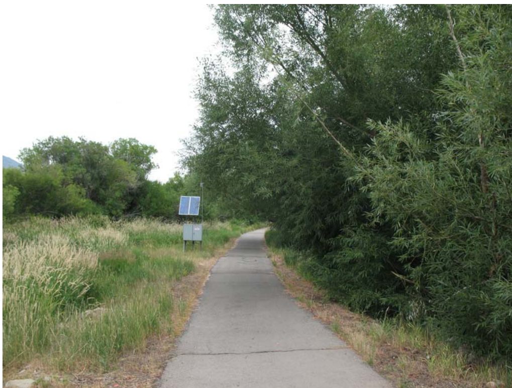
Photo 5. View to the northwest along the multi-use path from the southern end of the project area.
