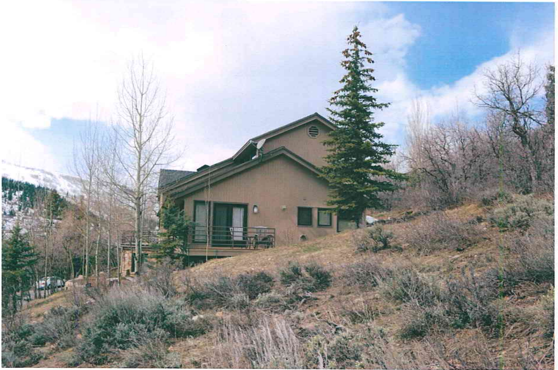
Sunnyside, Lot 11 – looking west
