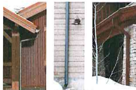
Gutters must complement the homes style
