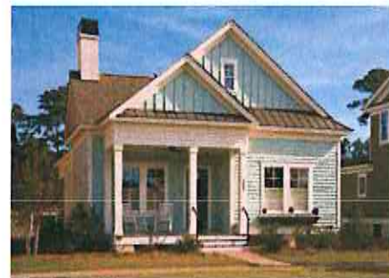
Porch roof forms are consistent with home
