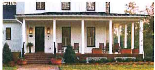
Porch raised above finished grade
