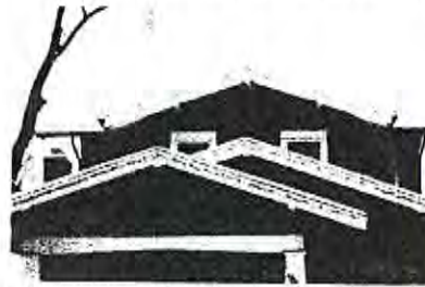
Appropriate roof overhangs
