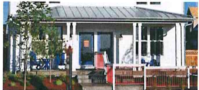
Properly detailed porch elements
