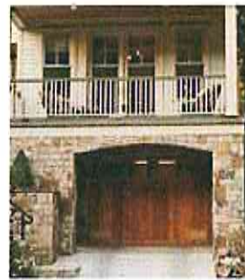
Patio over garage lessens its visual impact
