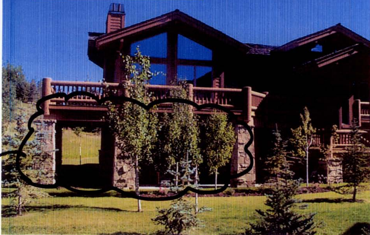
Looking north from rear of Unit 1
