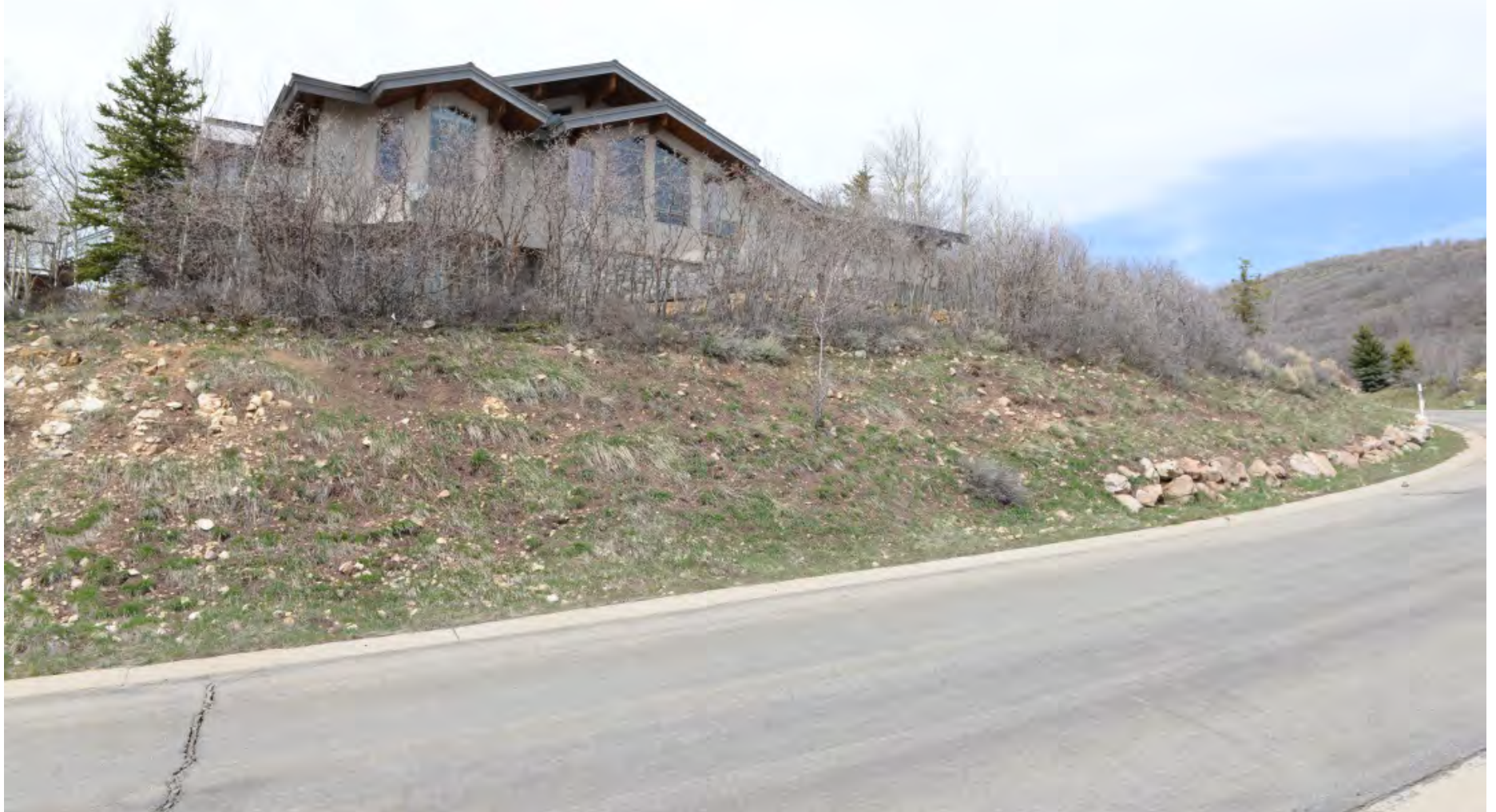
Morning Star Estates, Lot 9 – Looking west
