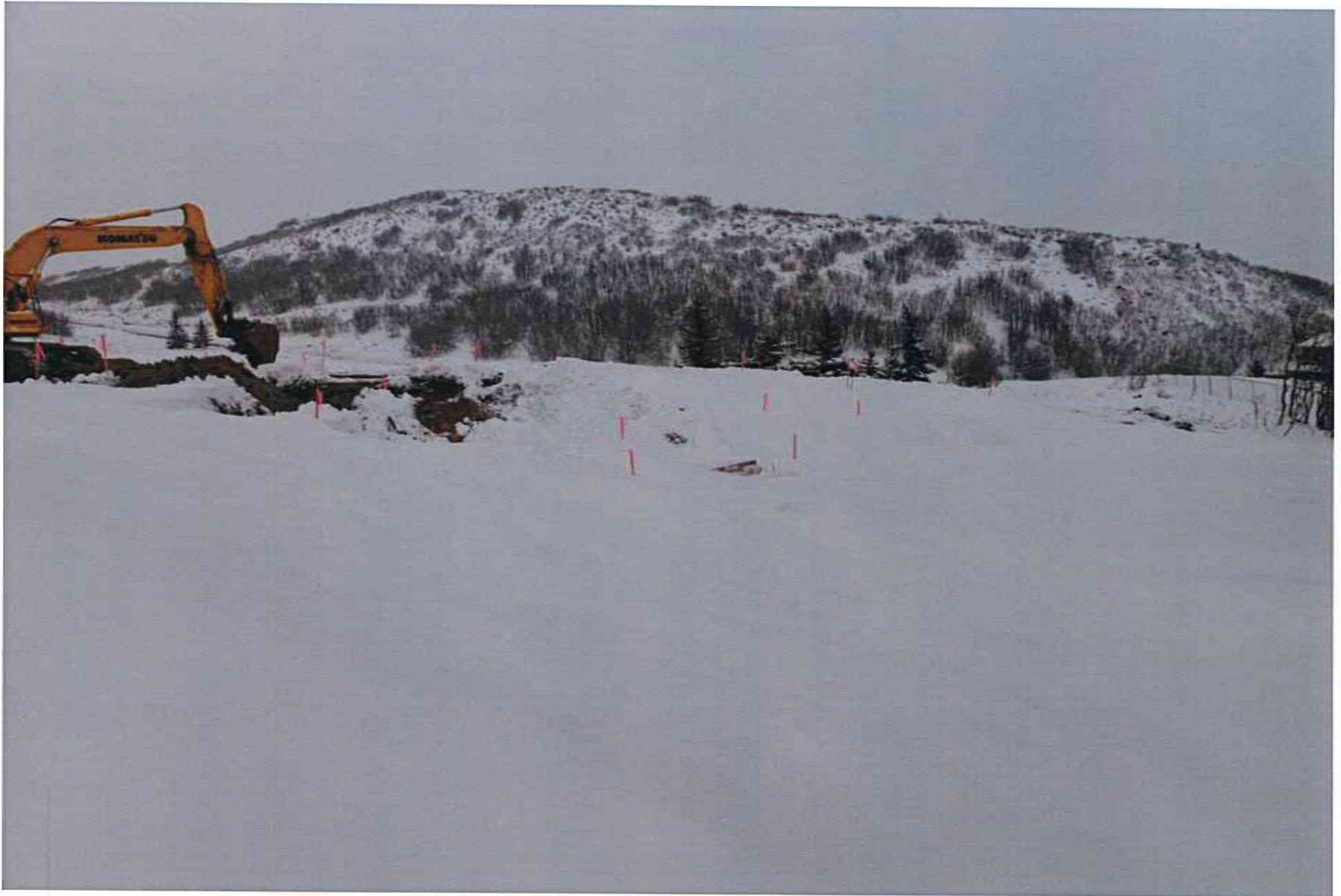
3776 Rising Star Lane - Looking northeasterly
