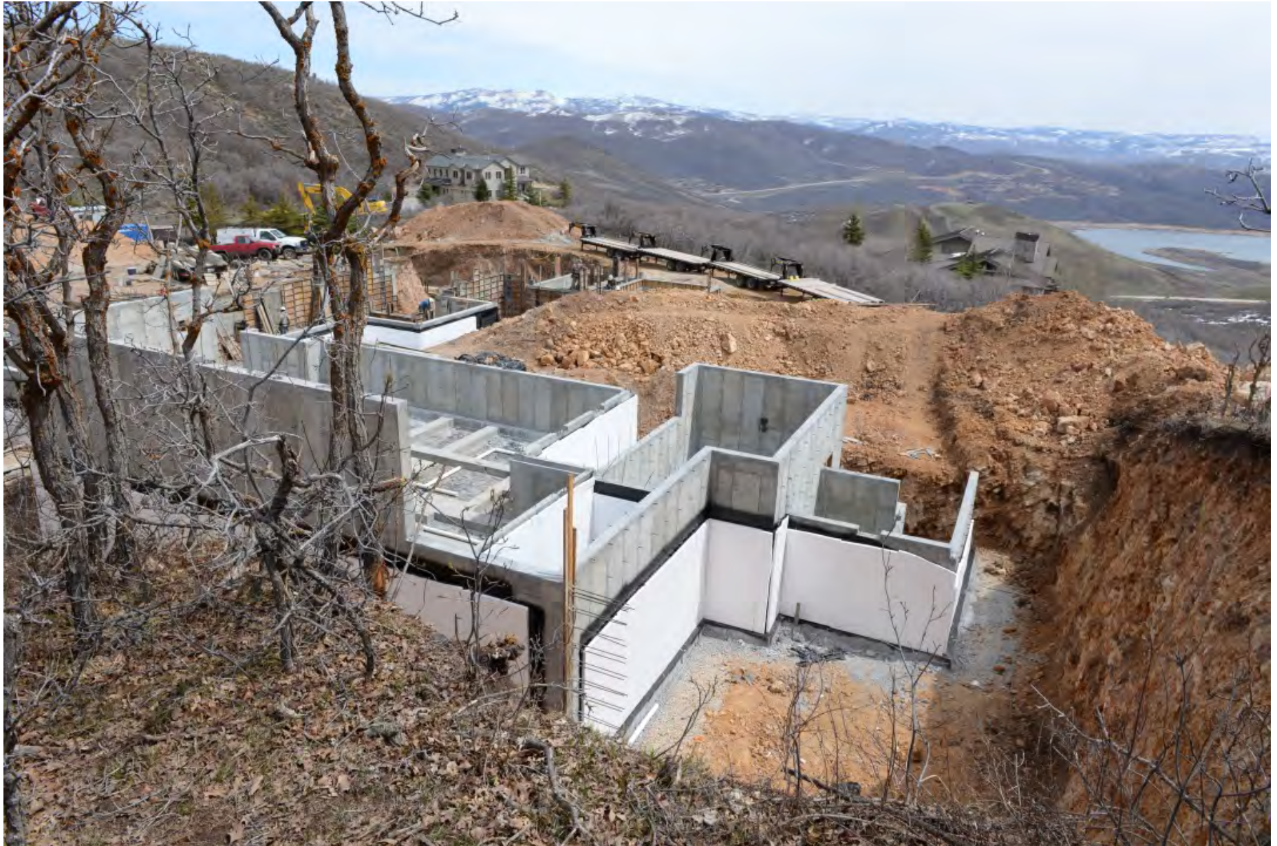
Morning Star Estates, Lot 10 – Looking east
