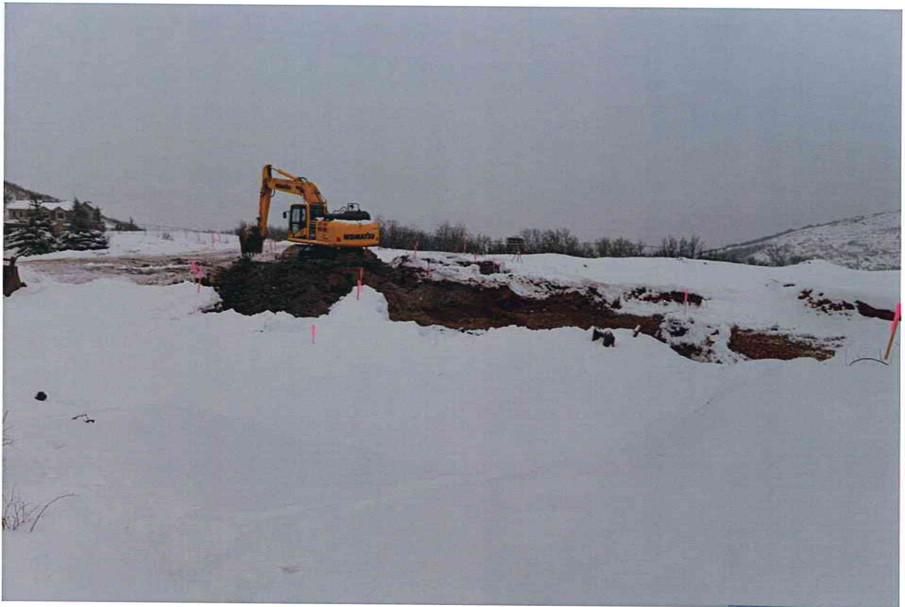
3776 Rising Star Lane - Looking southeasterly
